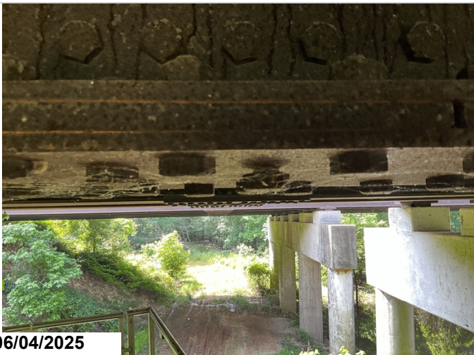
Span 22, Girder 3, Field splice, Bottom, Left: Bolt loose.
