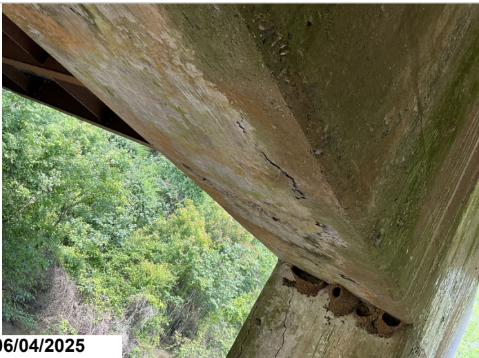
Cap, Bent 15, Bottom, Between Columns 2 & 3: 3' cracks and delaminations, and one small spall no exposed reinforcing steel.
