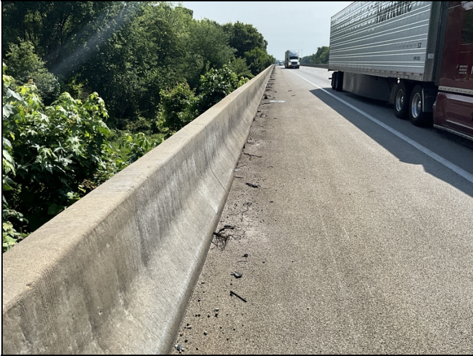
Deck Gutters, Full Length: Dirt and debris.
