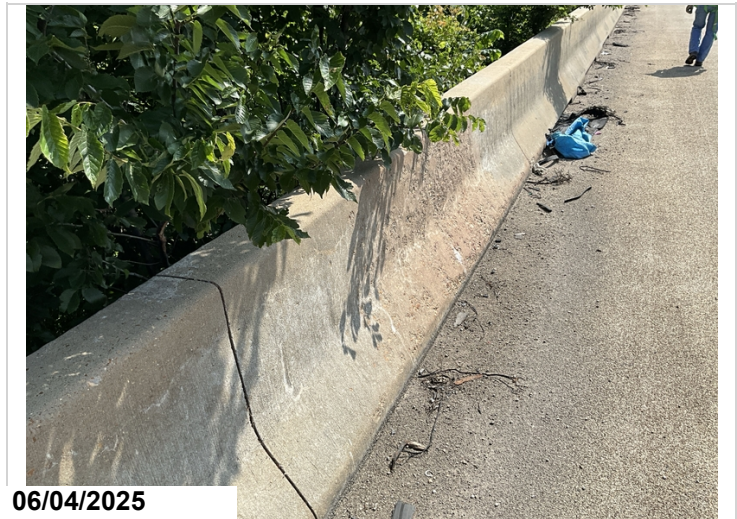
Span 12, Bridge Rail, Left: 5' of collision fire damage.
