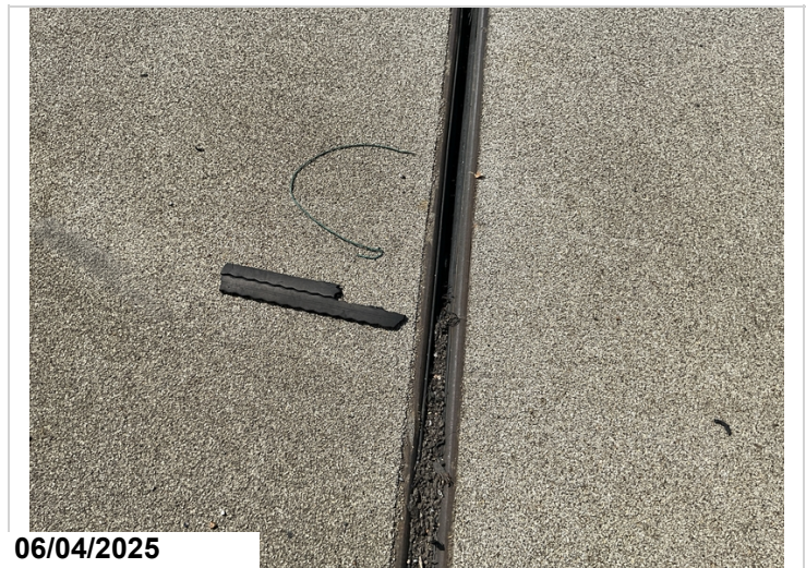
Joints, In Gutters: Debris impactation.
