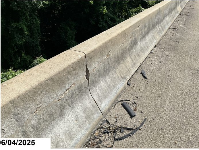
Bridge Rails, Full Length: Minor collision damage.
