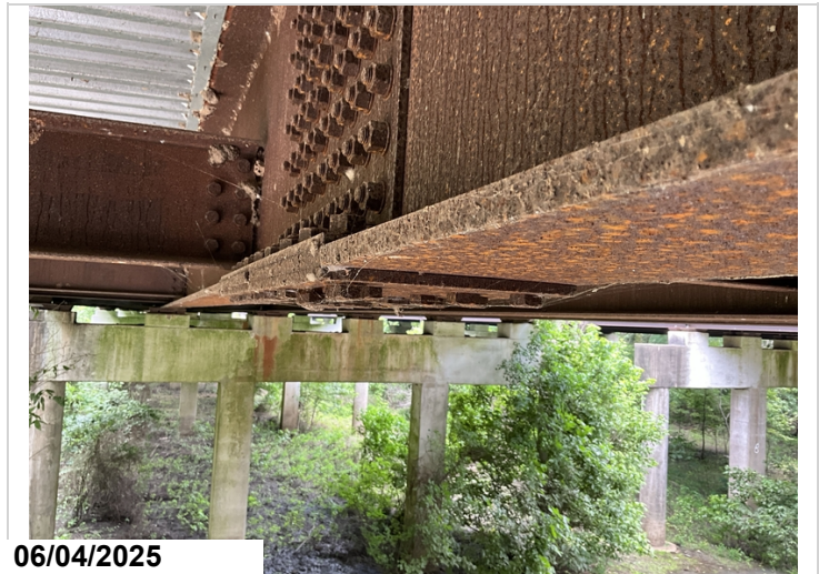
Span 7, Girder 2, Field Splice, Bottom, Left: Bolt Loose.
