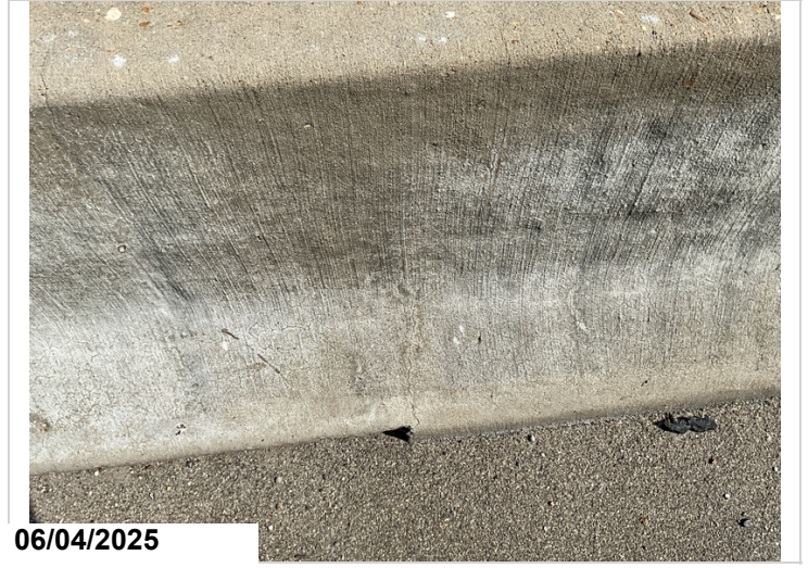
Bridge Rails, Full Length: Minor collision damage.
