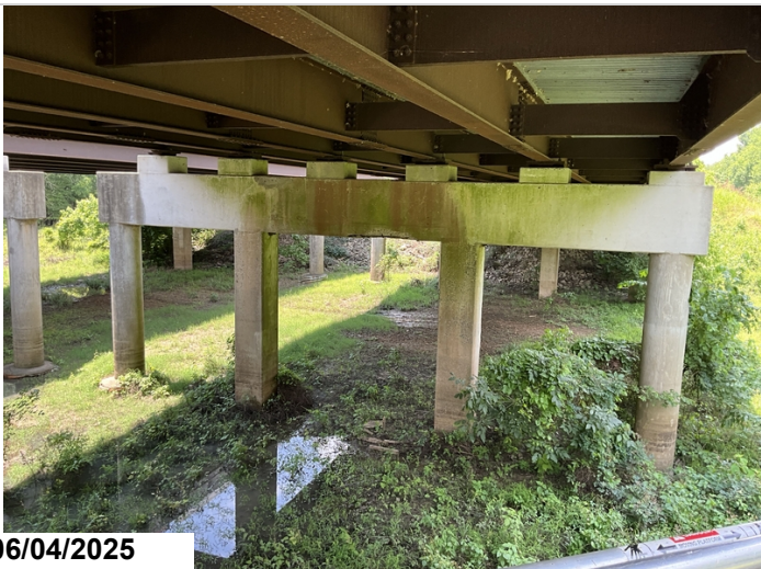
Cap, Bent 3, Ahead, Bottom, Between Columns 2 & 3: 8' of cracks with delaminations. 4' spalled with exposed reinforcing steel with moderate section loss.
