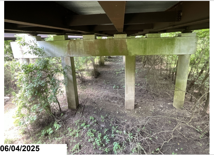
Cap, Bent 12, Ahead, Back, Bottom, Between Columns 2 & 3: 5' cracks with delaminations.
