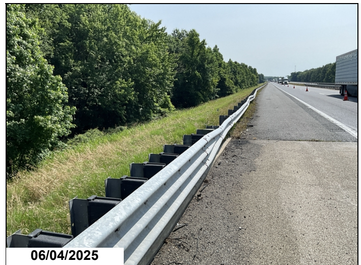
Abutment 2, Approach Rail, Left: Collision damage.
