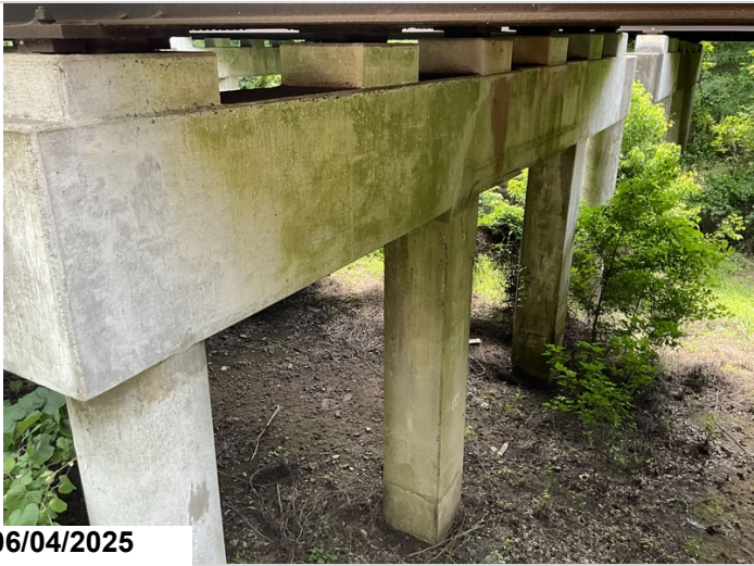
Cap, Bent 10, Back, Lower Corner, Starting At Column 2: 3' cracks with delaminations.
