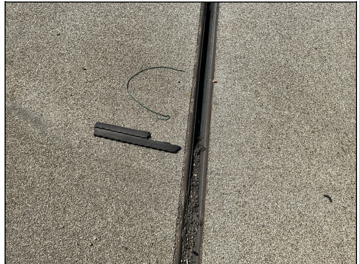
Joints, In Gutters: Debris impaction.
