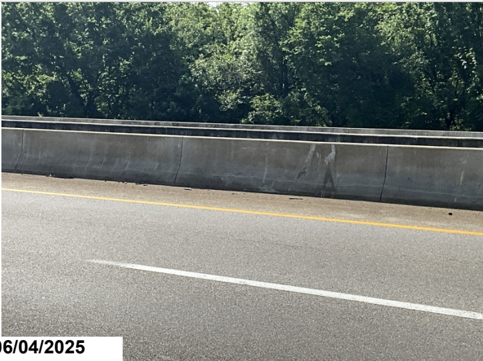
Bridge Rails, Full Length: Minor collision damage.
