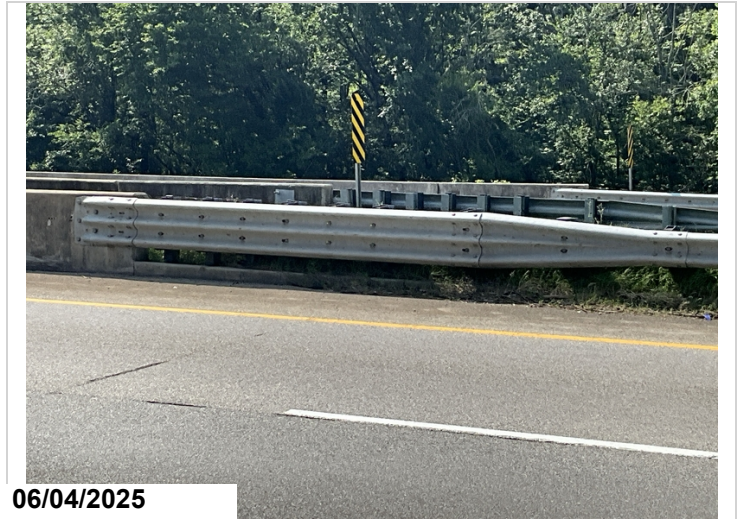
Typical approach rail transition
