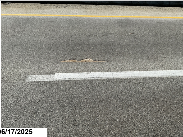
Wearing Surface, Span 22: 3" wide by 2' long wearing surface missing.
