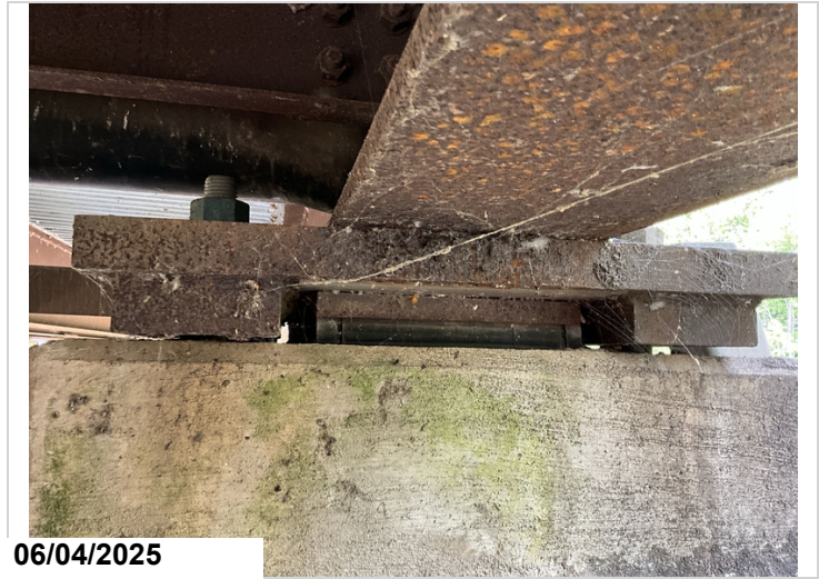
Span 16, Girder 1, At Bent 16, Bottom Of Bottom Flange: Active corrosion with laminations at bearing little to no section loss.
