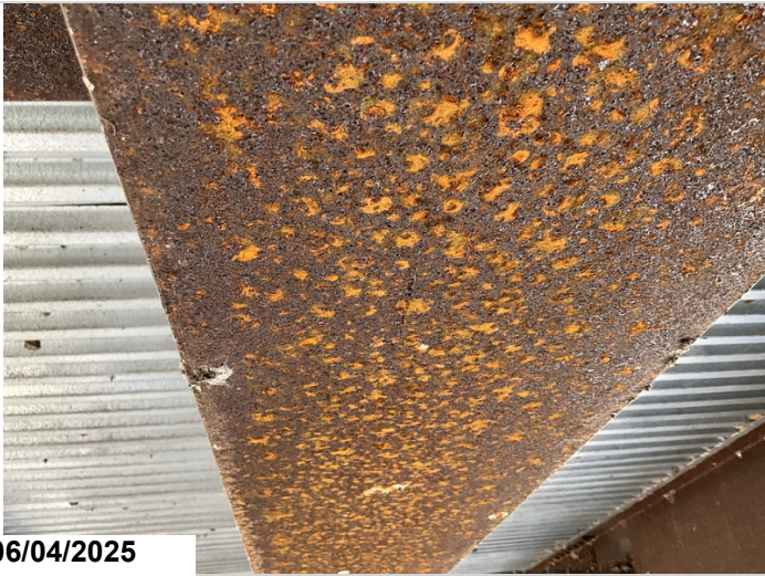
Typical minor delamination on bottom of girder.
