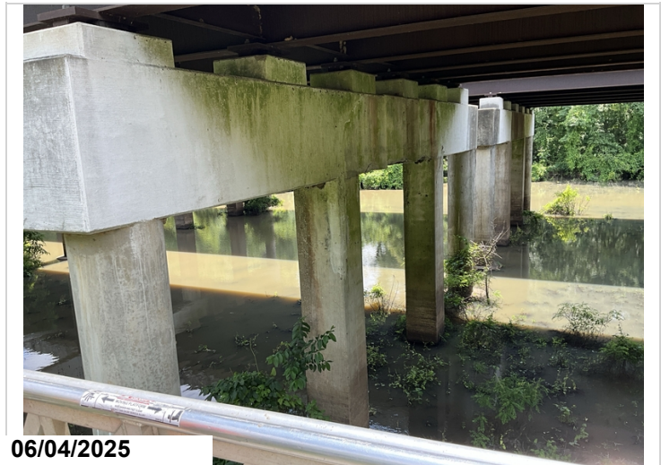
Cap, Bent 4, Back, Bottom, Between Columns 2 & 3: 6' spall with exposed reinforcing steel moderate section loss. 2' cracks with delaminations.
