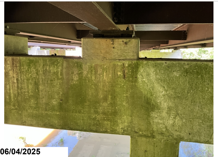
Cap, Bent 22, Ahead, Under Girder 3: 1' exposed reinforcing steel minor section loss.
