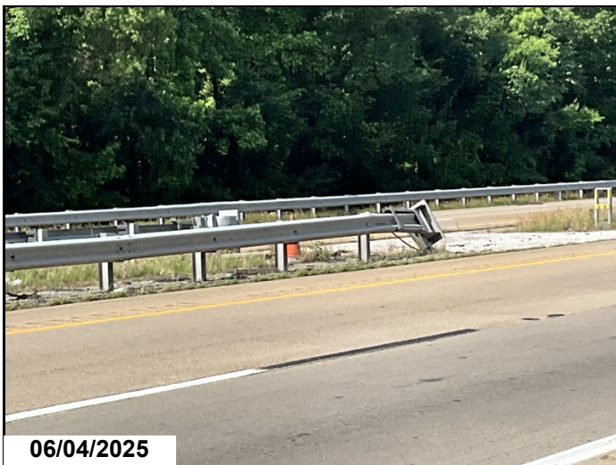
Abutment 1, Approach Rail, Right, Terminal End: Collision damage.
