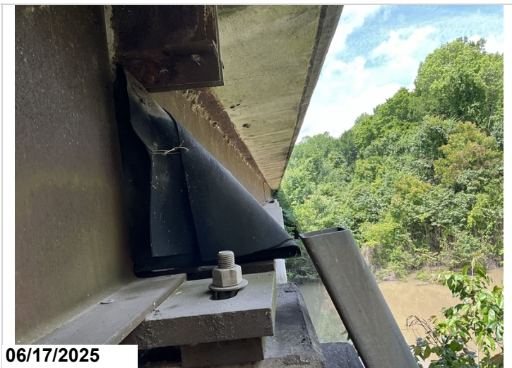
Bent 8 & 16, Joint Drain, Under Bridge: Disconnected not working.
