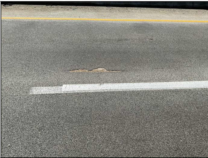
Wearing Surface, Span 22: 3" wide by 2' long wearing surface missing.
