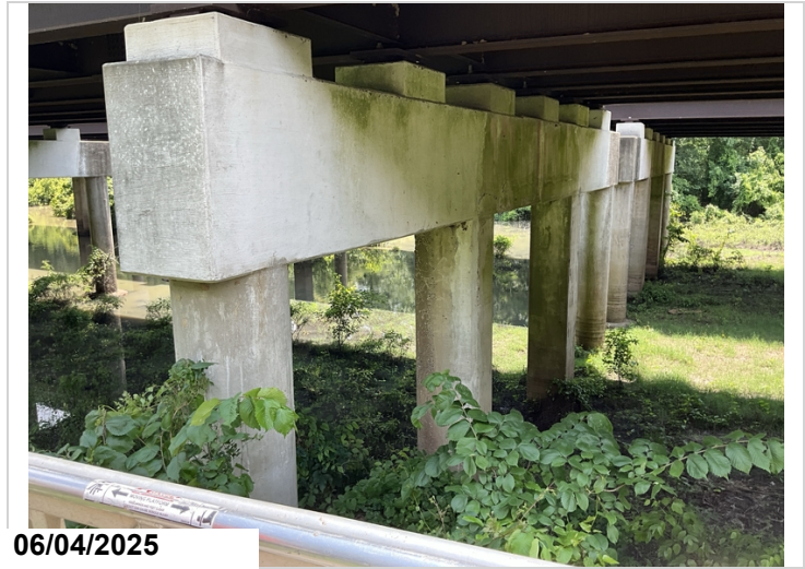
Cap, Bent 3, Back, Bottom, At Column 2: 2' cracks with delaminations.
