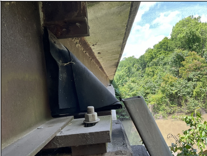
Bent 8 & 16, Joint Drain, Under Bridge: Disconnected not working.
