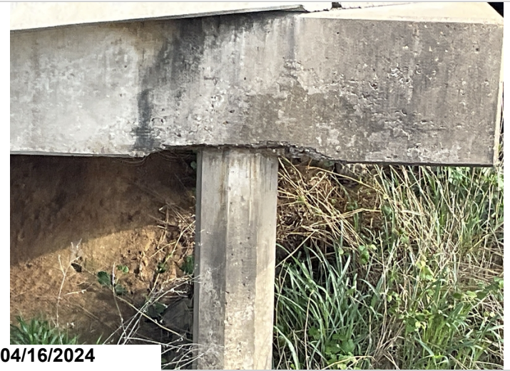
Bent 3, pile cap, back face, at bottom: 3' spall with exposed reinforcing steel with minor section loss on bottom edge at pile 8.
