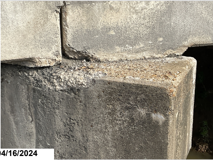
Bent 2, pile cap, right end, top: is scaling with one foot spall back face top edge no exposed rebar.
