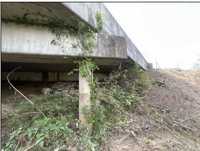
Vegetation growing beside, under and onto bridge.
