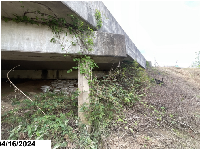
Vegetation growing beside, under and onto bridge.
