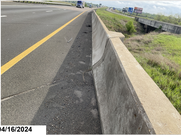
Dirt and debris in gutters
