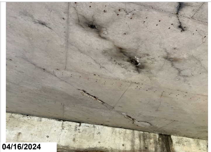
Soffit / undersurface of deck, span 3, near pile 3, at abutment 2: 2' delaminated area with a 3' spall with exposed reinforcing steel having minor section loss. Delam 2SF CS3, Rebar 3SF CS3
