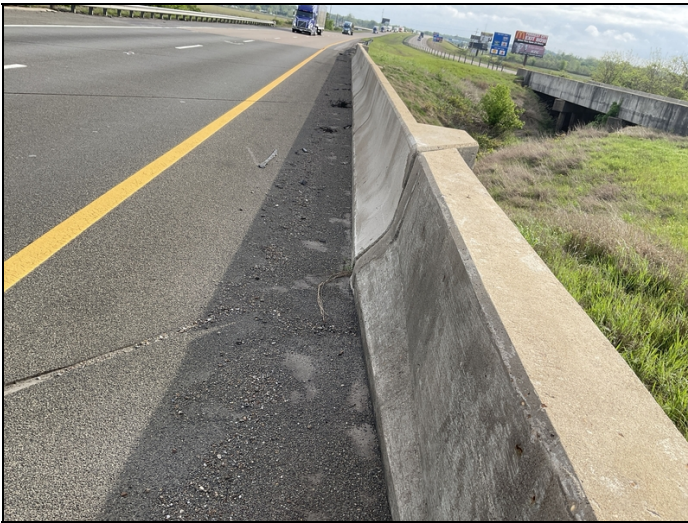
Dirt and debris in gutters
