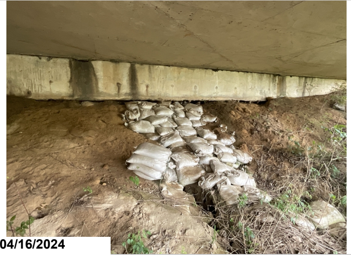
Abutment 1, slope: minor erosion a few inches deep under cap, exposing piles 3 and 4 slightly, area at pile 3 has sandbags placed.
