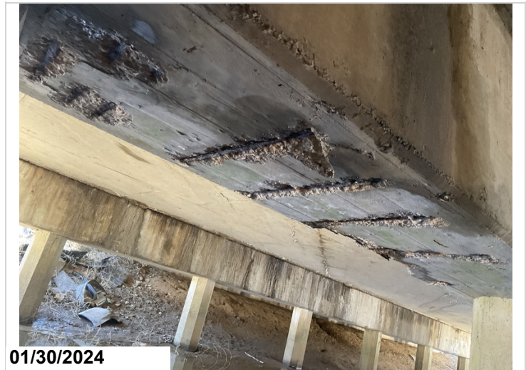
Spalling on bottom face of bent #3 cap at piles #4 and 5
