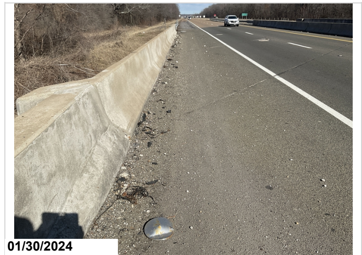
Dirt and debris in gutters
