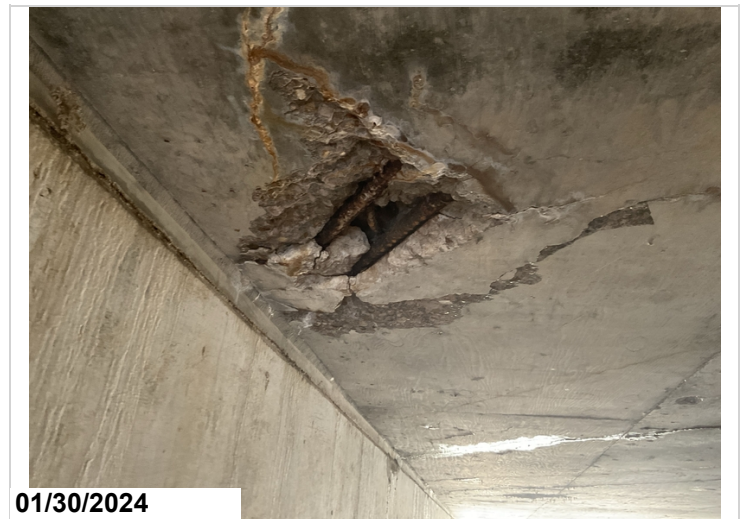
Typical soffit spall with exposed rebar span #1
