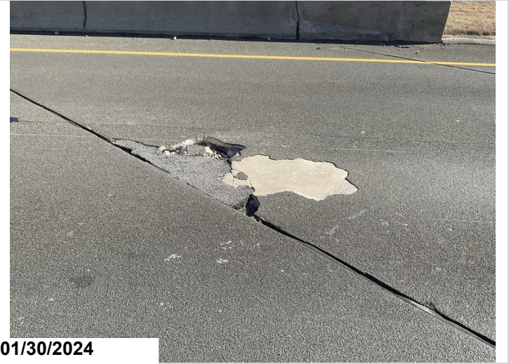
Span #1 right lane at bent #2 has a four foot long by one-foot wide ACHM patch and a two-foot spall up to four inches deep with exposed rebar and four-square feet of missing epoxy overlay.
