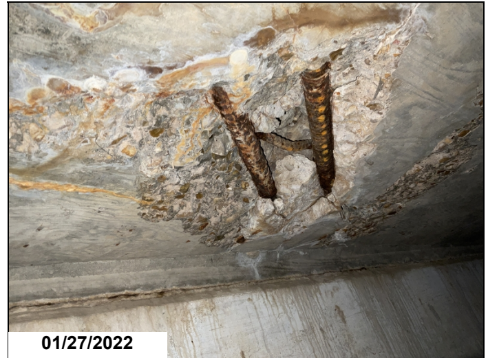
Span #1 right lane at bent #2 has a 3' x 3' spall with ACHM patch reflecting through to soffit-under surface with spall and exposed rebar.
