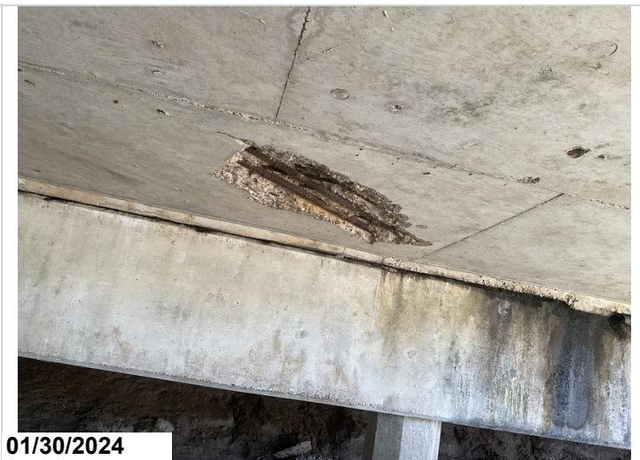
Span #2 soffit has a three foot spall near bent #3 pile #6 with exposed rebar with minor section loss.
