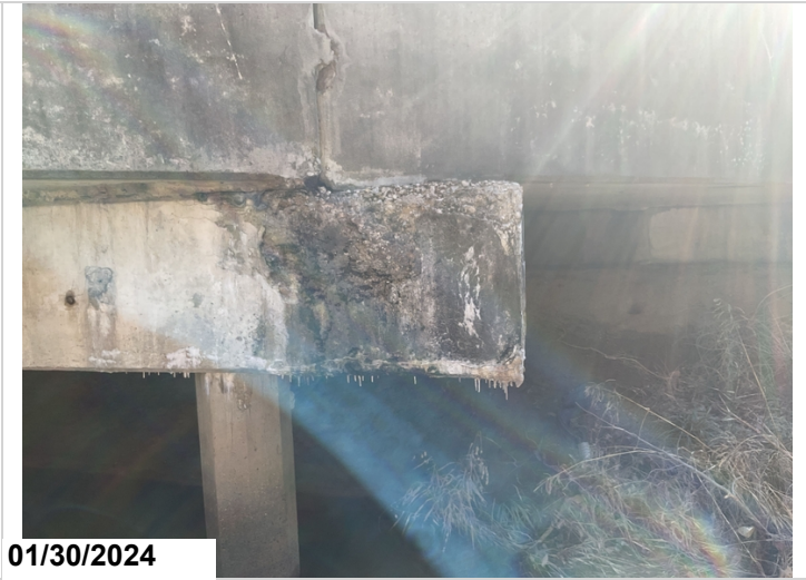
Bent #2 cap left end has heavy scaling with loose aggregate
