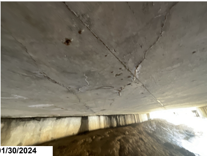
Typical soffit cracks with rust staining and efflorescence
