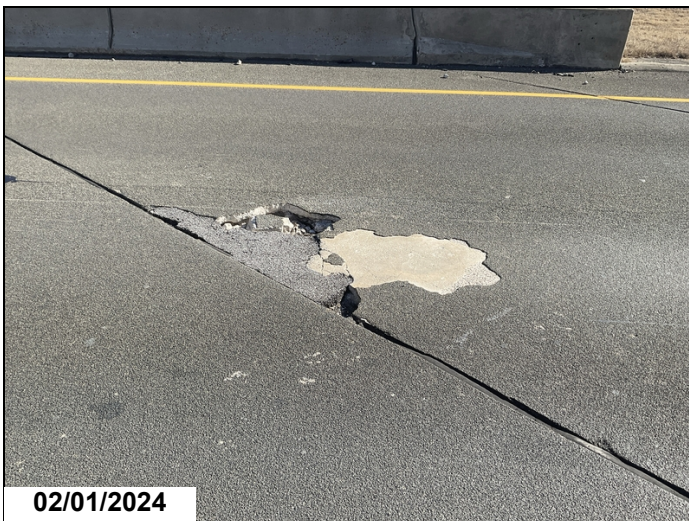
Span #1 right travel lane at bent #2 has a four foot long by one-foot wide ACHM patch and a two-foot spall up to four inches deep with exposed rebar and four-square feet of missing epoxy overlay
