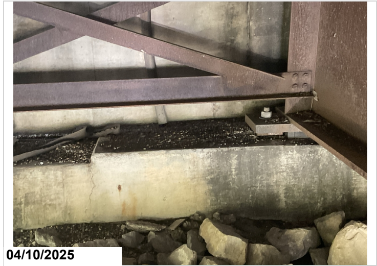
Dirt and debris on abutment caps
