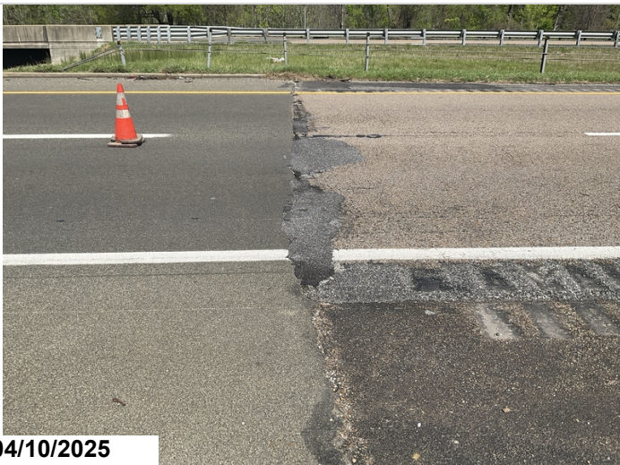
Abutment 2, approach roadway, left lane: asphalt minor spalling.
