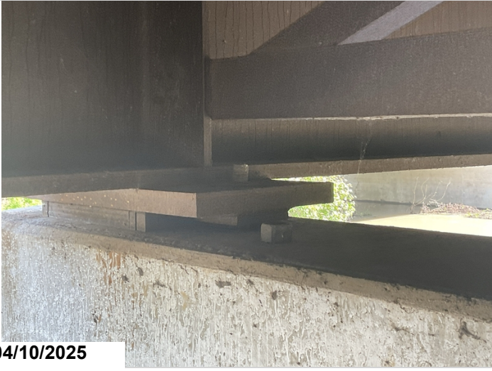
Span 1, girder ,1 bent 2, right bearing nut: sitting on bent.
