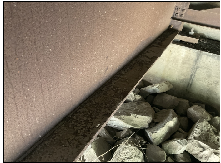
Span 7, girder 3, bottom flange and lower web, last 10': scaly rust.
