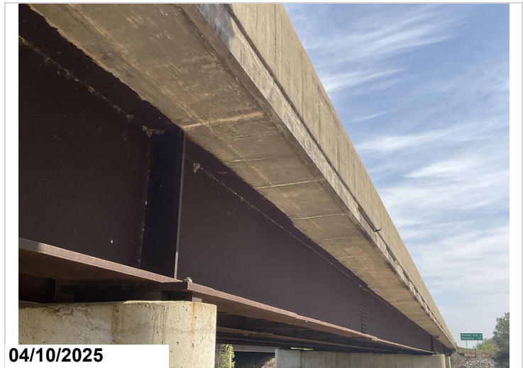
Typical cracking with light efflorescence in undersurface of overhang.
