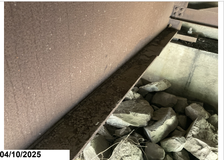
Span 7, girder 3, bottom flange and lower web, last 10': scaly rust.
