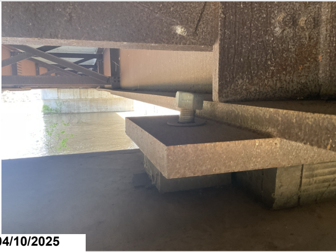
Bent 5, girder 3, left anchor bolt: moves in concrete.
