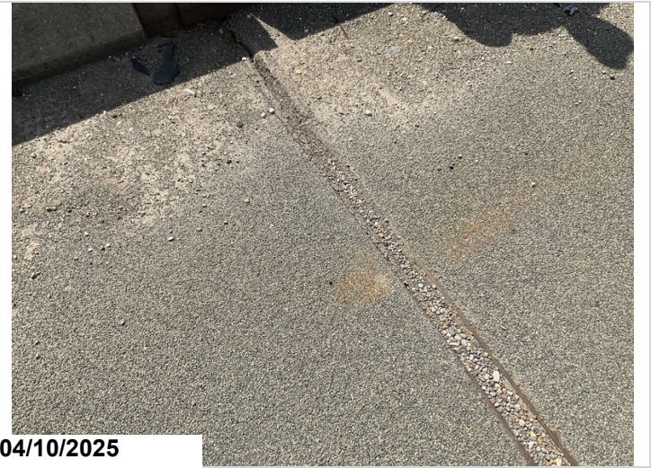
Typical debris impaction of joints.
