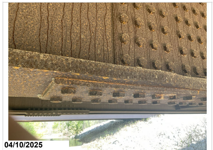
Span 7, girder 3, lower field splice: initial pack rust. Typical of girder 4.
