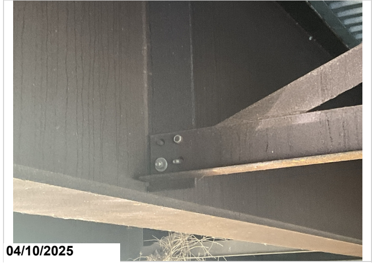
Span 1, girder 4, diaphragm 3, right lower bolts: loose with two missing nuts.
