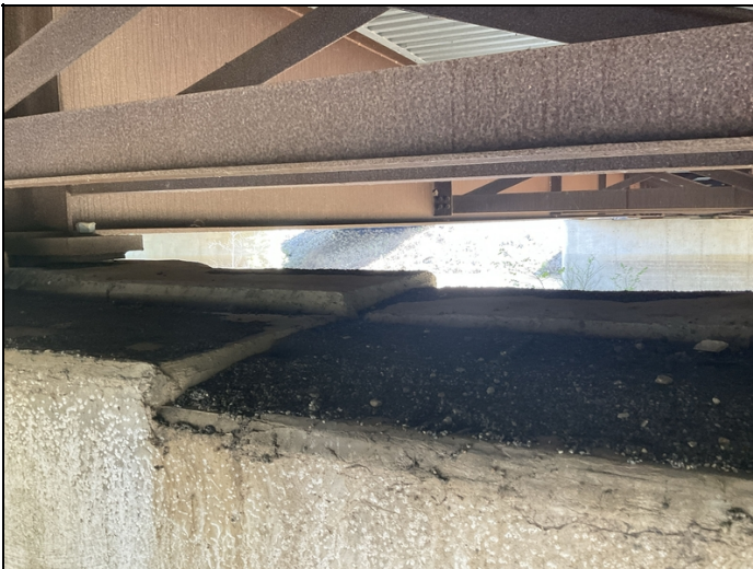
Dirt and debris on bent 5 pier cap
