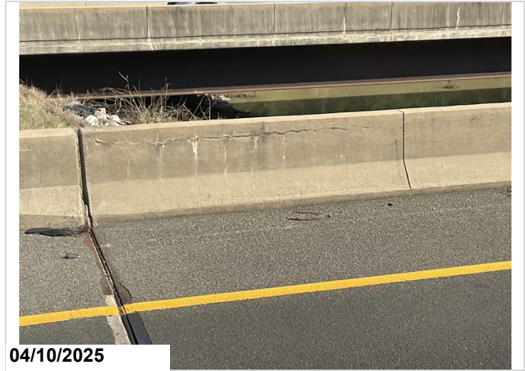
Typical longitudinal cracking in bridge rail
