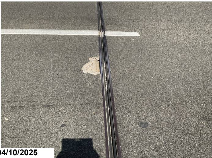
Span 5, deck, right lane, at bent 6 joint: 1' spall with no exposed reinforcing steel.
