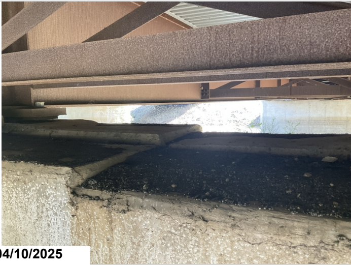
Dirt and debris on bent 5 pier cap
