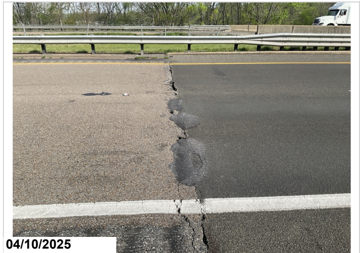
Abutment 1, approach roadway, left lane: asphalt minor spalling.
