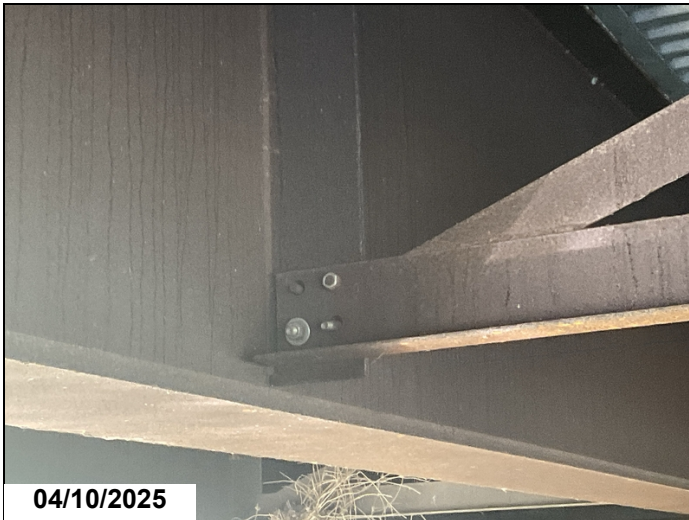
Span 1, girder 4, diaphragm 3, right lower bolts: loose with two missing nuts.
