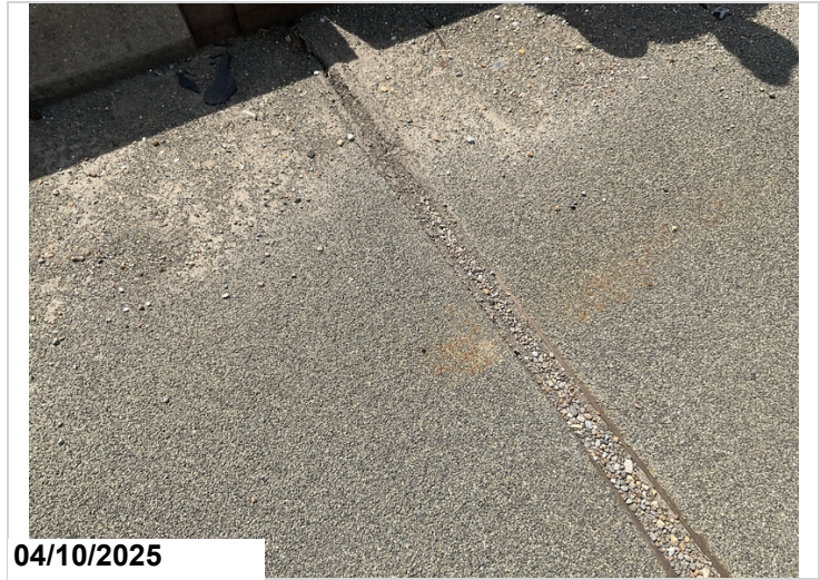
Typical debris impaction of joints.
