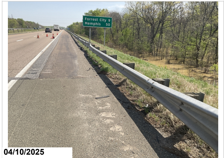
Abutment 2, approach rail, right side: approximately 40' moderate collision damage 60' from bridge end.
