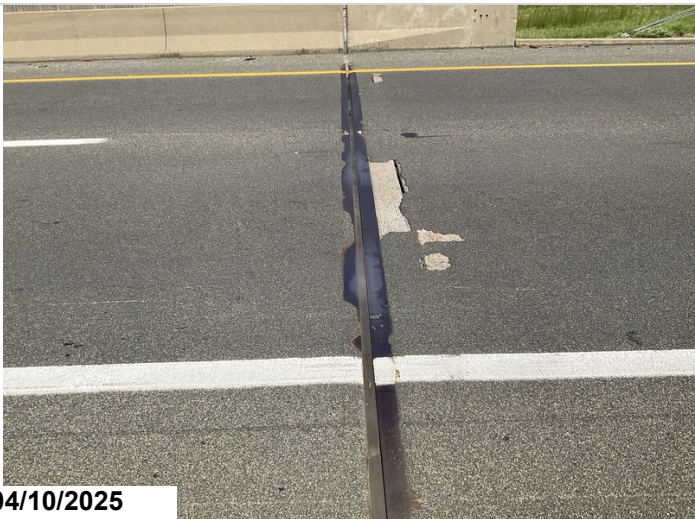
Abutment 2, pourable joint seal
