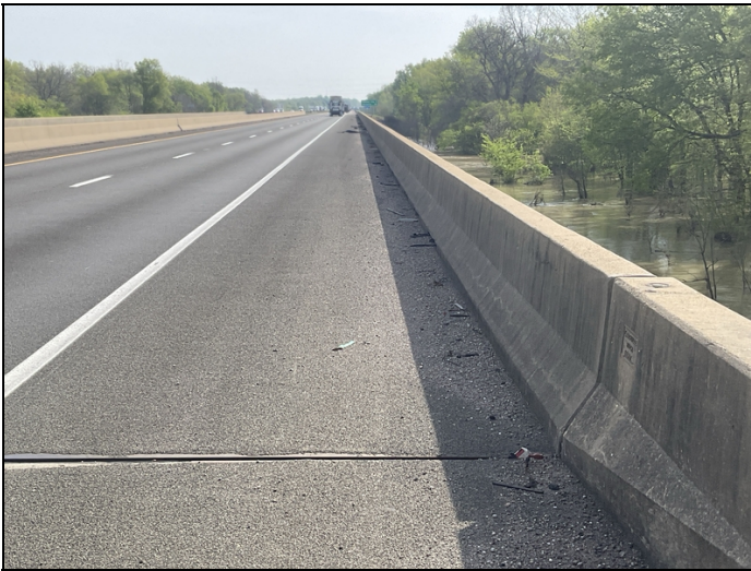
Dirt and debris in gutters
