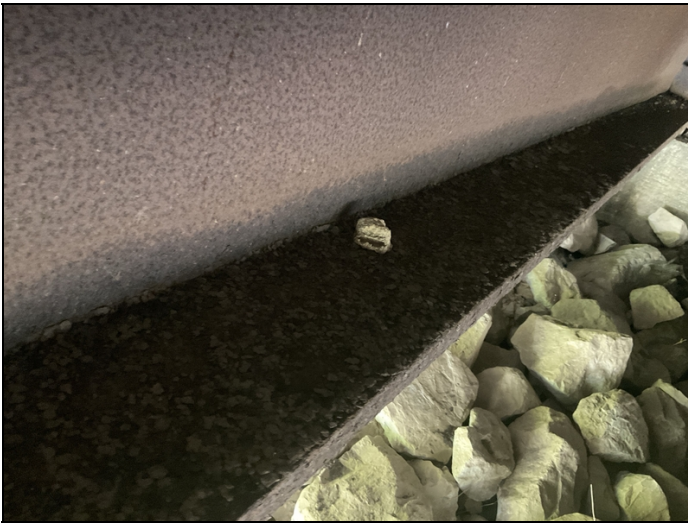
Span 1, girder 4, bottom flange and lower web: first 10' has flaky rust . Typical of girders 2,3,4.
