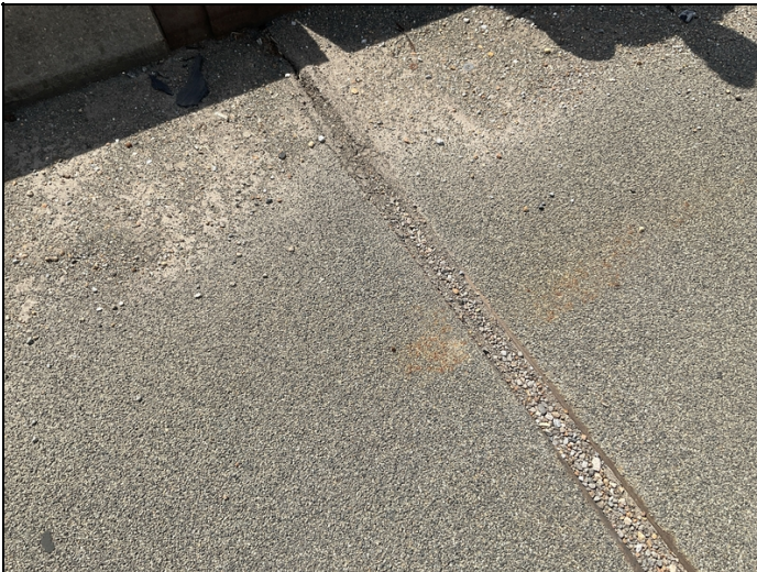
Typical debris impaction of joints.
