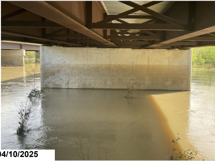
Typical intermediate bent
