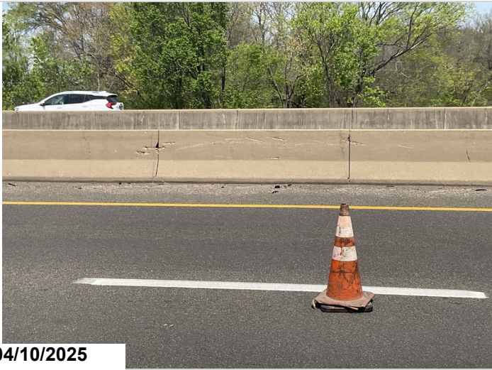
Span 3, bent 4, bridge rail, left side: 10' minor scrapes.
