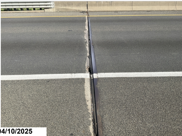
Abutment 1, pourable joint seal: splits and holes throughout 35LF total. Leakage 35LF CS4
