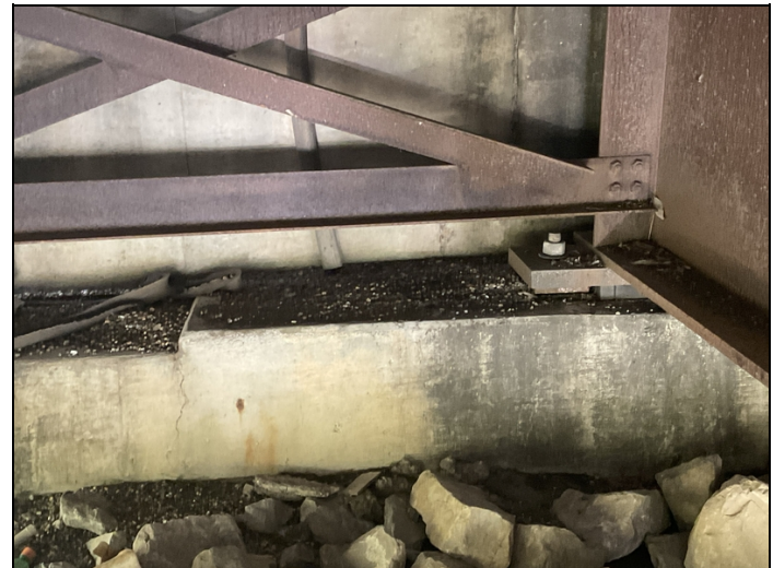
Dirt and debris on abutment caps
