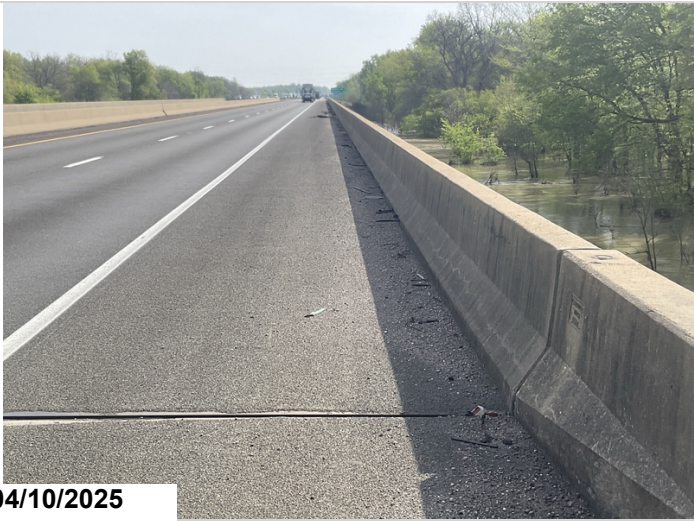
Dirt and debris in gutters
