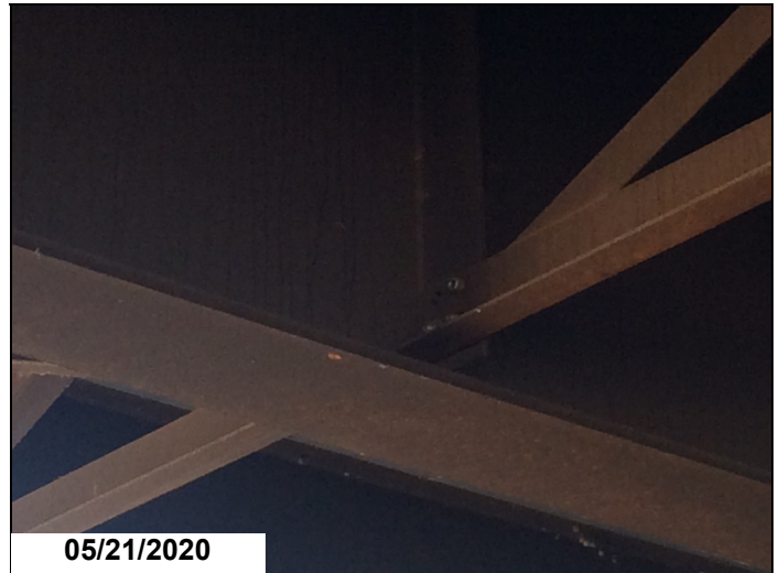
Typical loose diaphragm bolts
