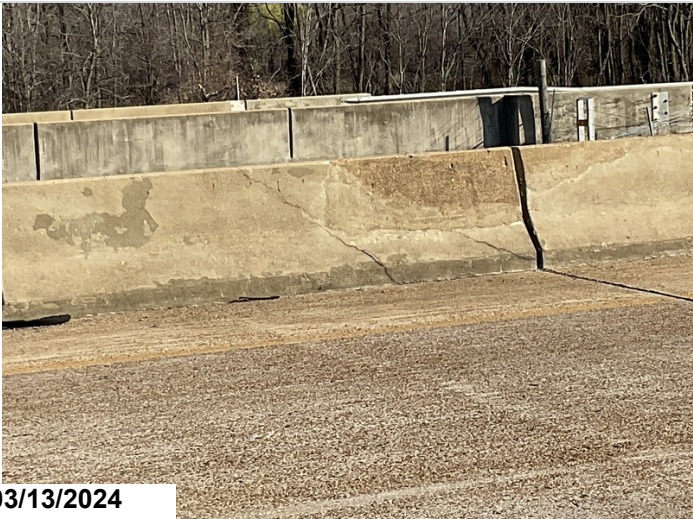
Span 4, bridge rail, left side: two 4' diagonal cracks.4LF CS3
