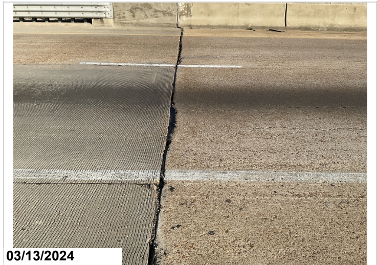
Pourable joint seal, abutment 1: 15' of seal missing
