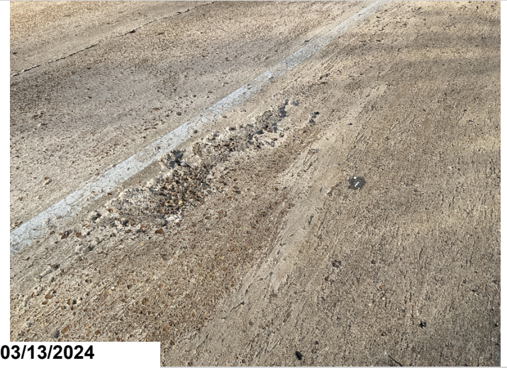
Span 4, deck, right gutter: 1' x 3' of moderate scaling. 3SQF CS3
