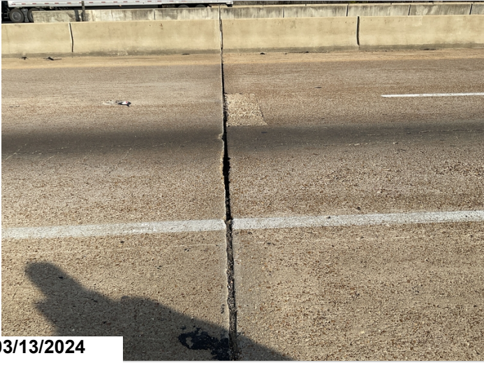
Pourable Joint Seal, Bent 2: Pourable joint seal missing across travel lanes.
