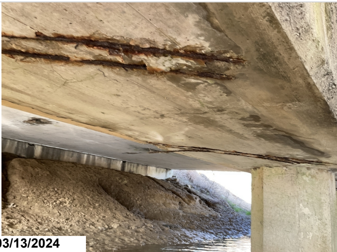
Typical exposed reinforcing steel on bottom face of pile cap
