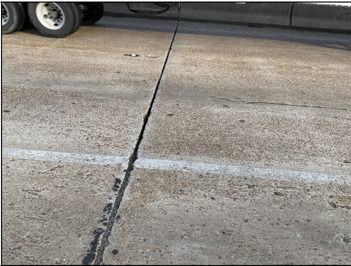
Bent 5 joint seal missing
