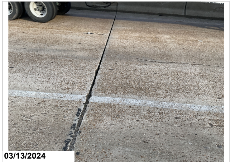
Bent 5 joint seal missing
