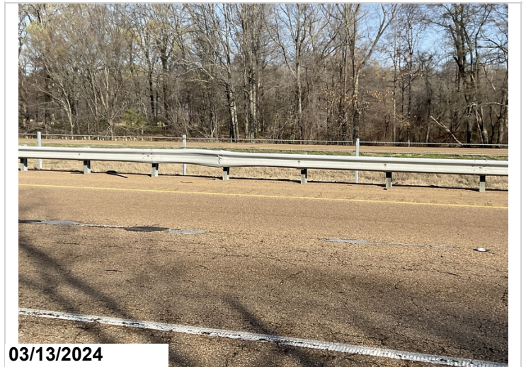
Abutment 1 right approach rail has 6' of moderate collision damage mid span.
