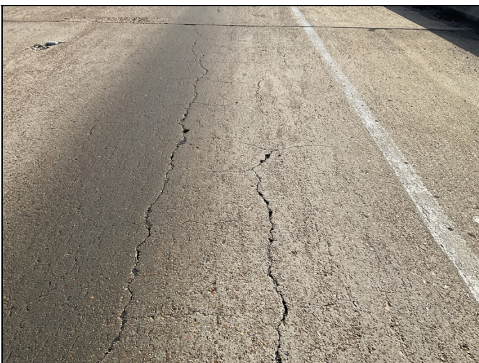
Deck cracking span 1 right lane
