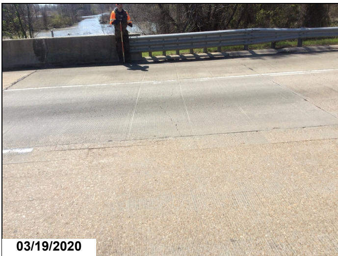
Typical transverse approach slab crack
