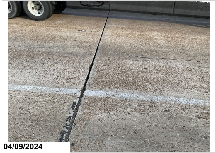
Bent 5 joint seal missing
