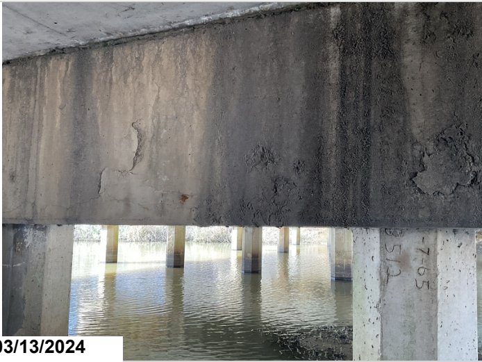
Bent #5 cap ahead face between piles 3 and 4 has one-foot delaminated area and three feet of longitudinal CS2 cracking.
