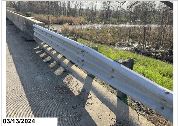
Abutment 1 right transition
