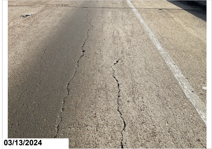
Deck cracking span 1 right lane
