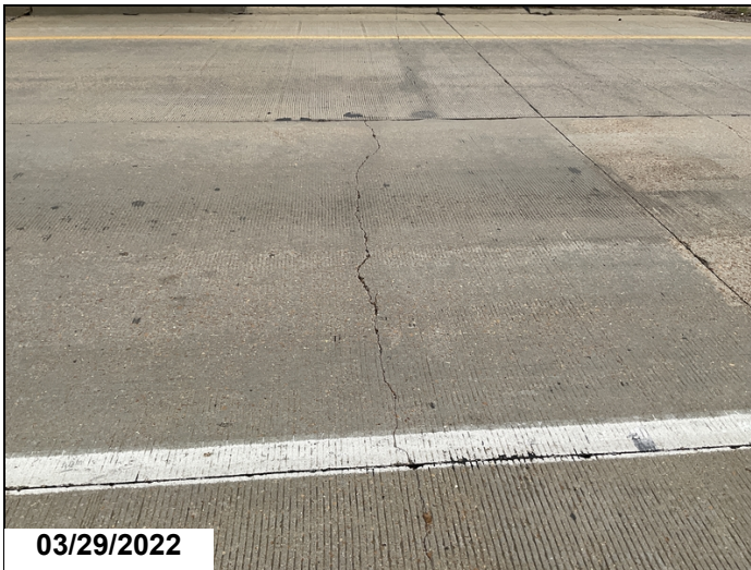
Typical transverse approach slab crack
