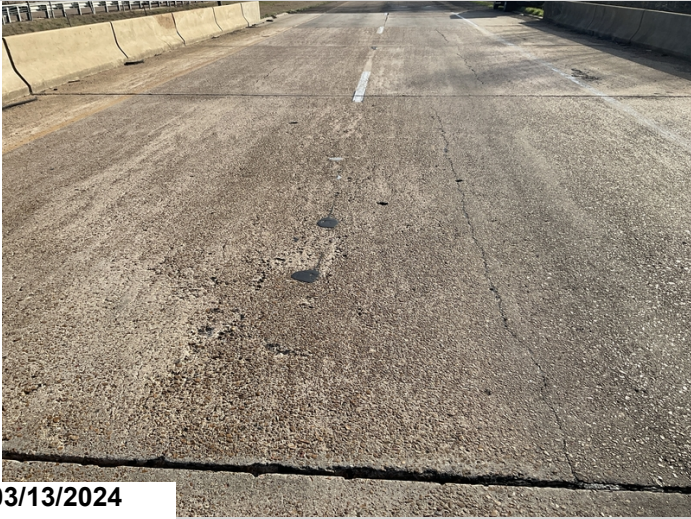
Deck, Span 3, Right Lane, Full Length: Sealed wide crack.
