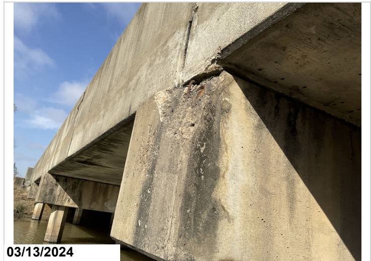
Bent 4 cap right end spalled with exposed rebar
