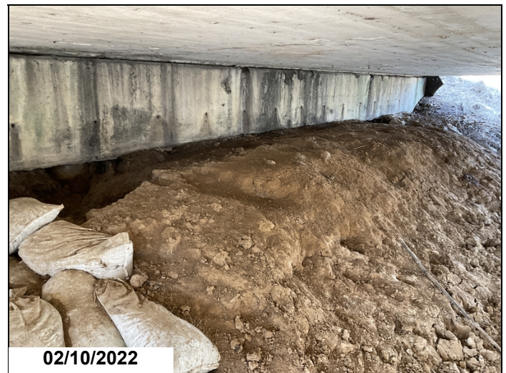
Abutment #1 has some erosion at cap exposing two piles.
