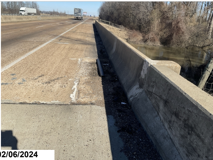
Dirt and debris in gutters
