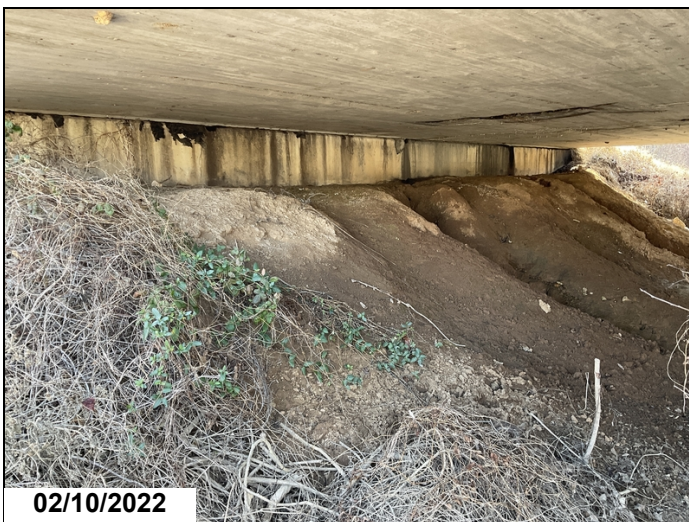
Abutment #2 slope is eroding to near vertical face within four feet of abutment with erosion veins running down slope.
