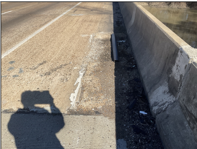
Span #1 right side patch in gutter scaling
