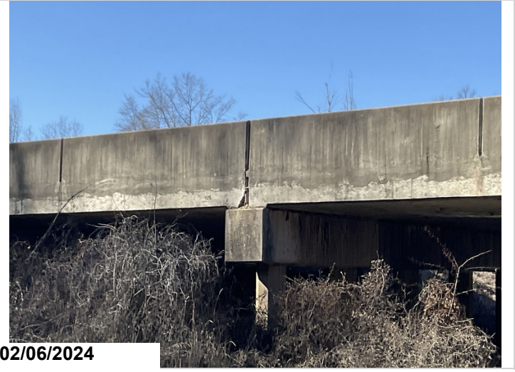
Span #2 right side at bent #2 end of slab spalled
