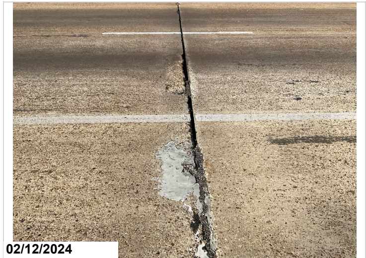
Typical missing joint material
