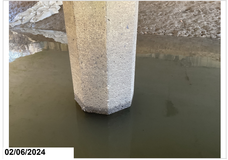
Typical light abrasion on piles
