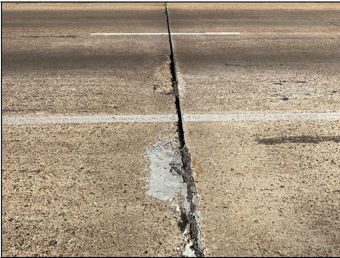
Typical missing joint material
