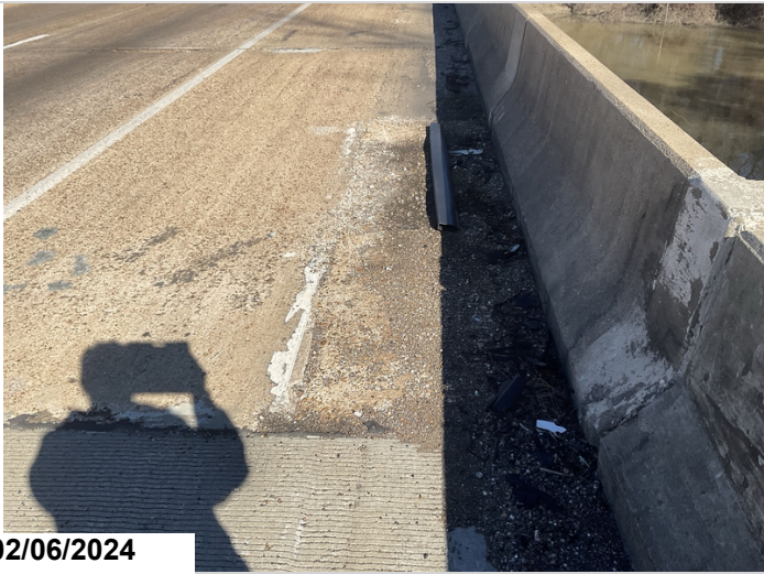
Span #1 right side patch in gutter scaling
