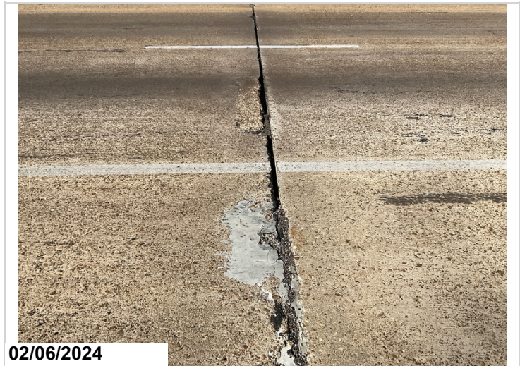
Typical missing joint material
