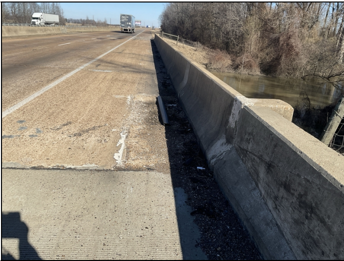
Dirt and debris in gutters
