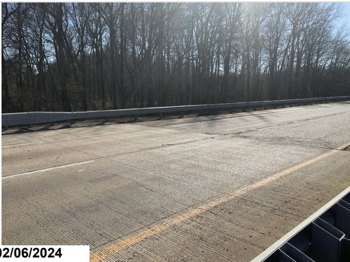
Abutment #1 right approach rail has 10 feet of moderate damage mid span
