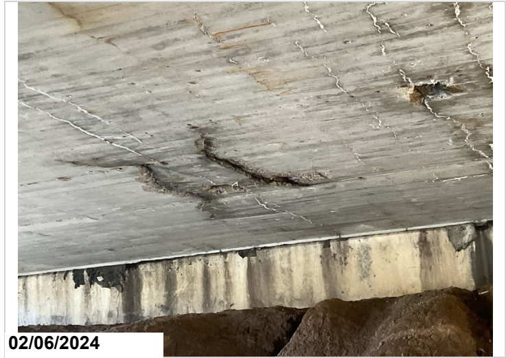
Large delaminated area span #5 soffit / underside of deck
