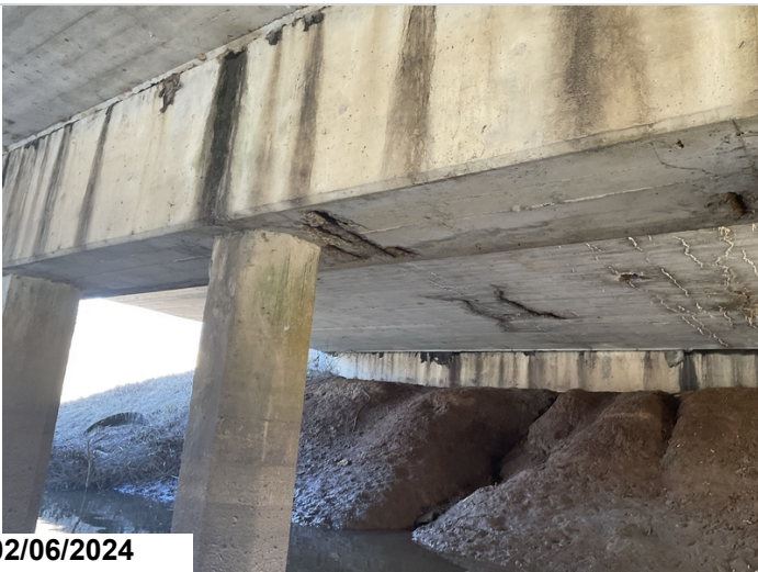
Exposed rebar bent #5 bottom face by pile #5
