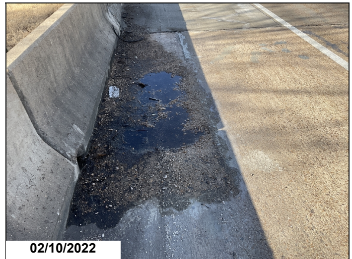
Span #1 has 15' of heavily scaled patches in right gutter.
