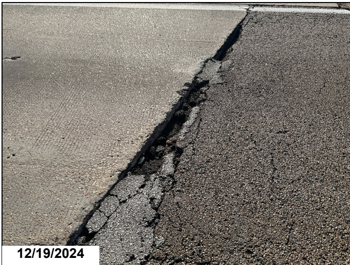
Abutment 1, approach roadway, right lane: spalled at joint with approach slab.
