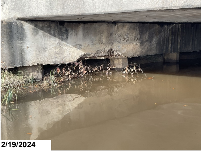
Abutment 1, pier cap, ahead, between piles 6 and 7: 4' spall with exposed reinforcing steel with moderate section loss.
