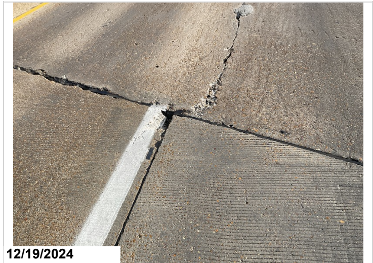
Abutment 1, approach slab, at centerline: small spall
