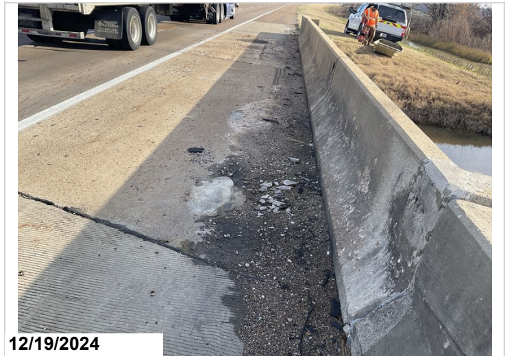
Dirt and debris in gutters
