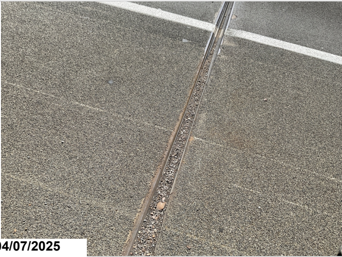
Typical dirt and debris in joint.
