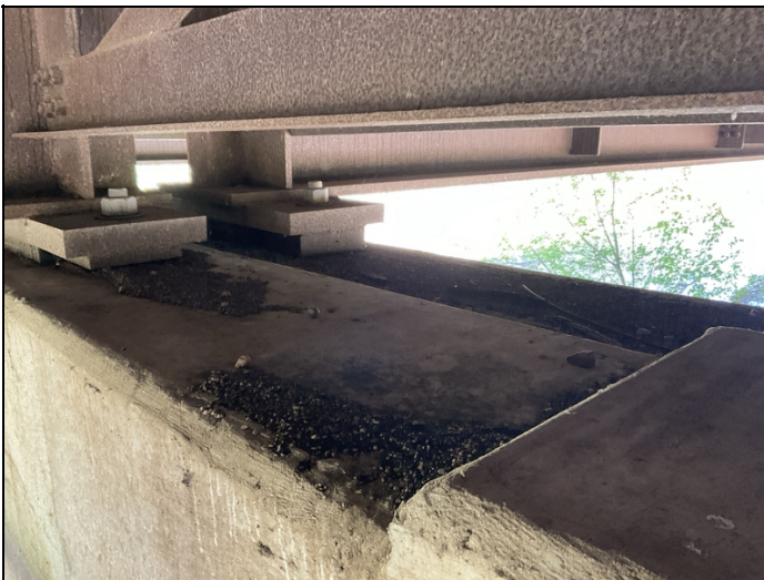
Typical dirt and debris on bent 3 pier cap.
