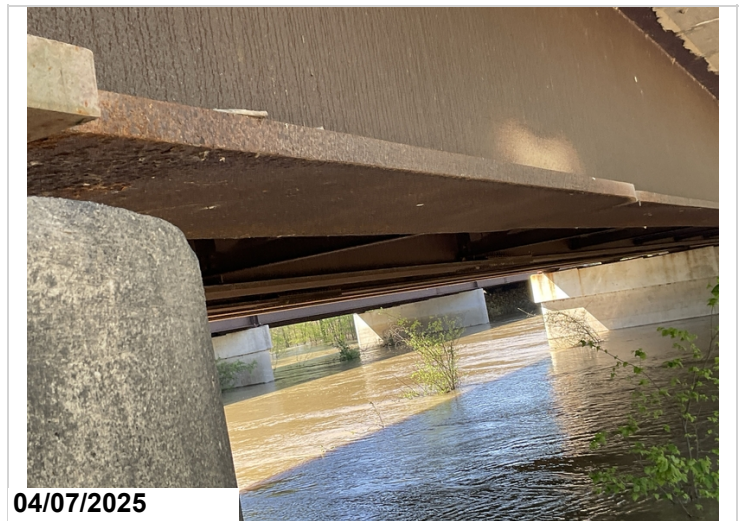
Span 3, girder 1, bent 4, last 10' on bottom of bottom flange and lower web: some scaling rust 1/4" or less flakes.
