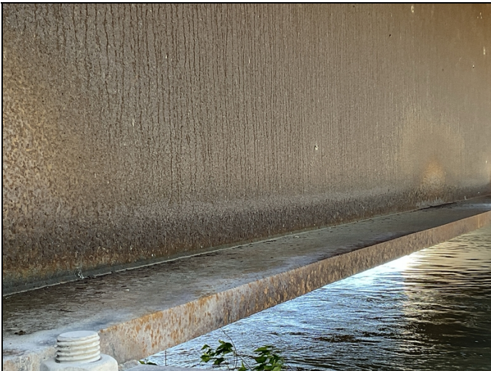
Span 4, girder 1, bent 5 last 10': minor scaling on outside web and bottom flange.
