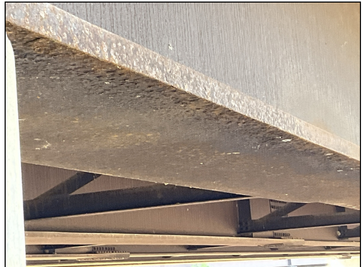
Span 4, girder 1, bent 5 last 10': minor scaling on bottom of bottom flange has minor scaling.
