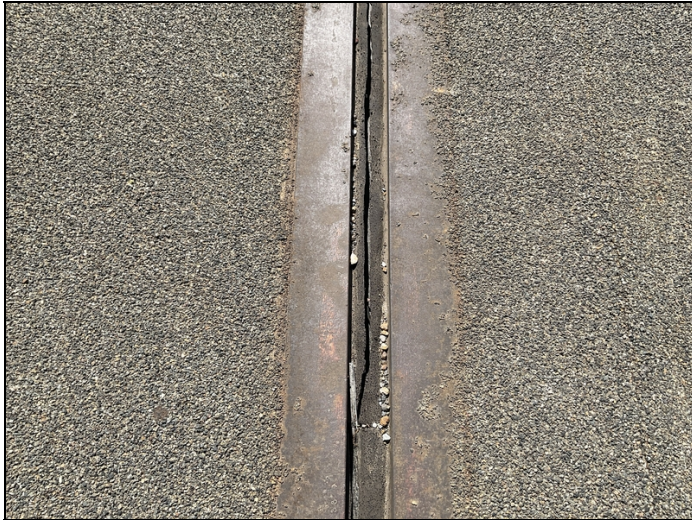
Abutment 1, pourable joint seal: split full width, typical split.
