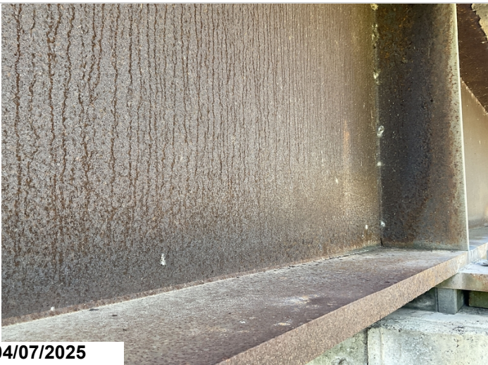
Span 5, girder 1, bent 5, first 3': minor scaling on outside web and bottom flange.
