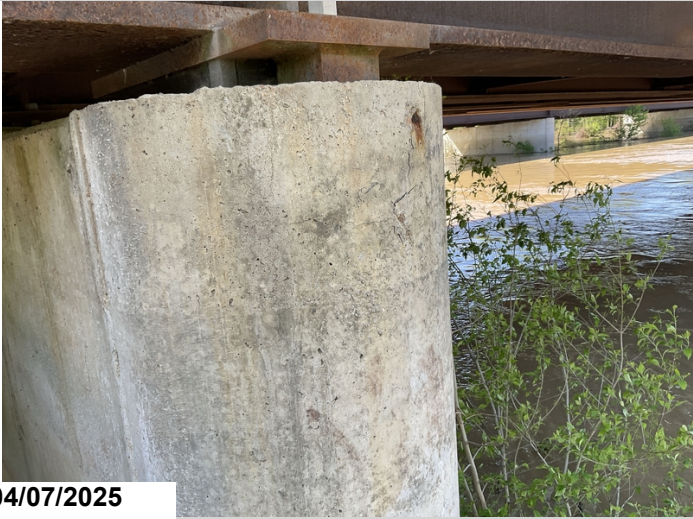
Bent 5, pier wall, left end: small, delaminated area with small piece of reinforcing steel exposed at top.
