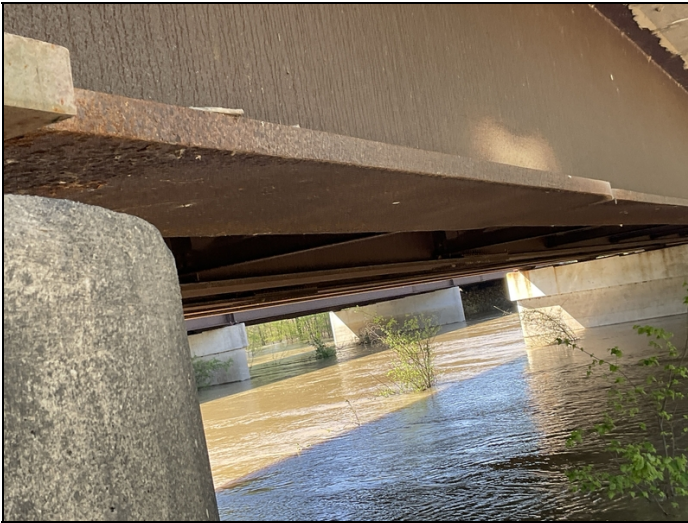
Span 3, girder 1, bent 4, last 10' on bottom of bottom flange and lower web: some scaling rust 1/4" or less flakes.
