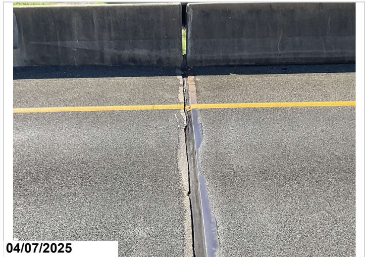
Abutment 2, pourable joint seal, right lane: split.
