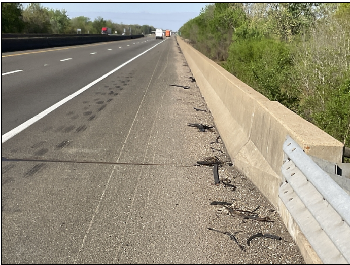
Dirt and debris in gutters.
