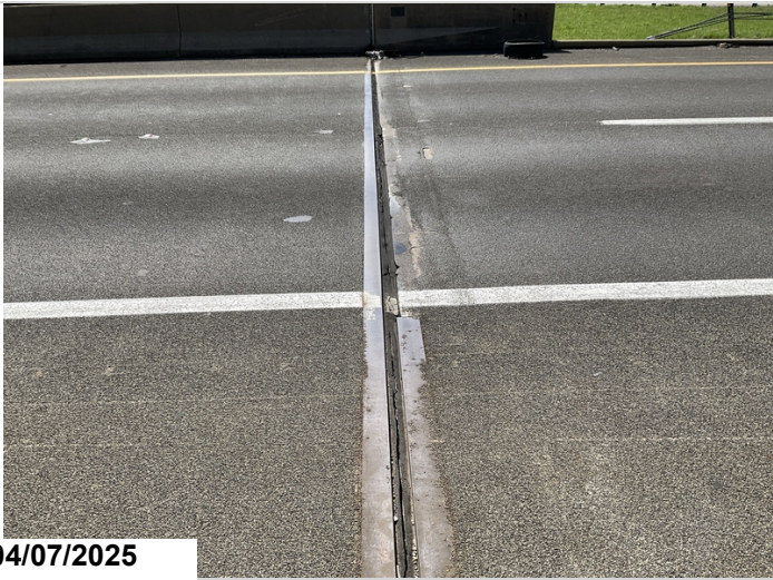
Abutment 1, pourable joint seal: split full width.
