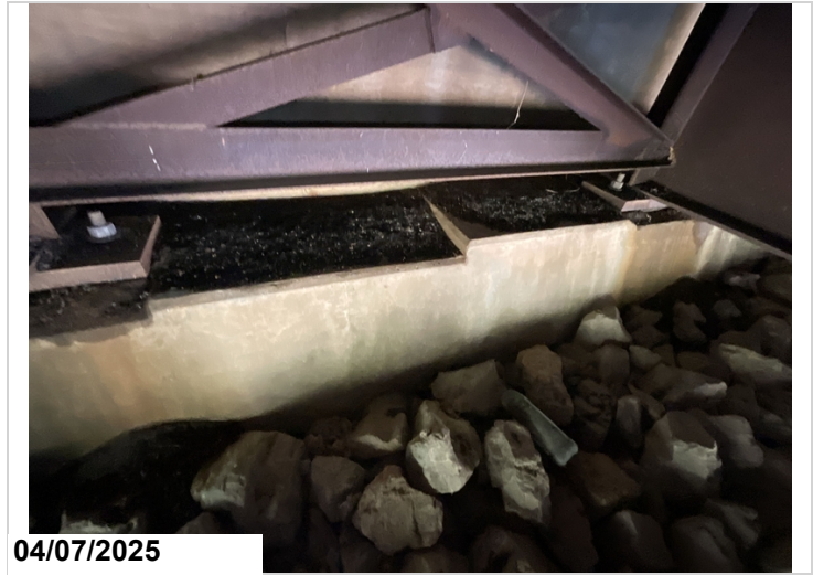
Dirt and debris on abutment caps.
