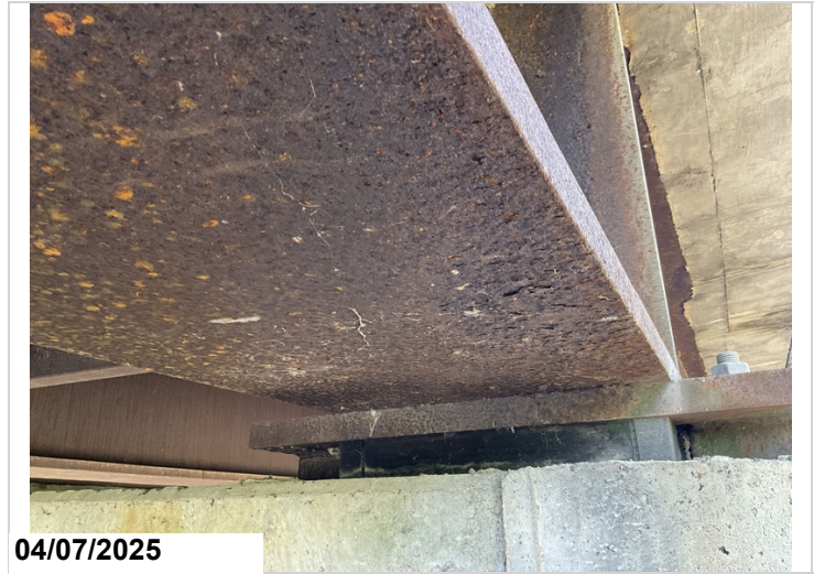
Span 5, girder 1, bent 5, first 3': minor scaling on bottom of bottom flange has minor scaling.
