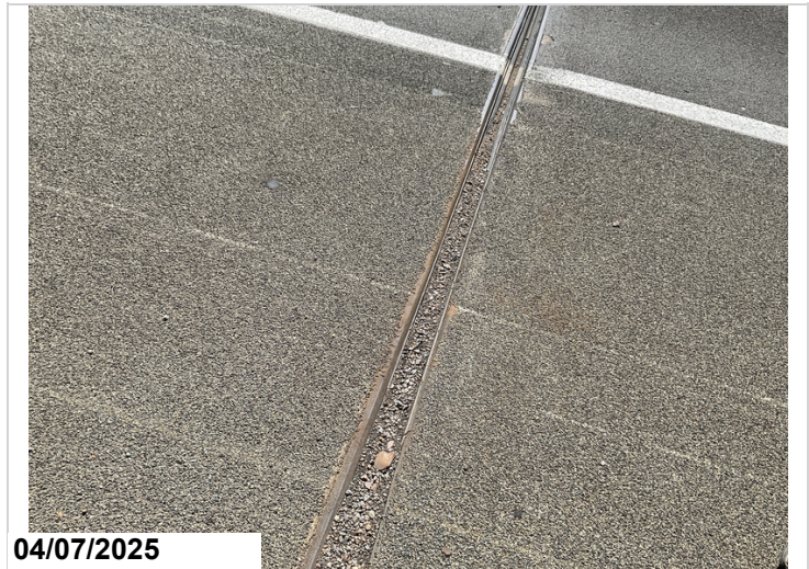
Typical dirt and debris in joint.
