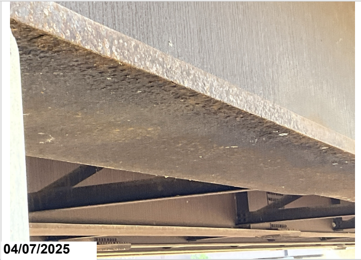
Span 4, girder 1, bent 5 last 10': minor scaling on bottom of bottom flange has minor scaling.
