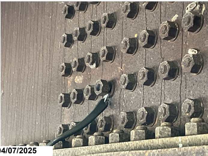
Span 3, girder 1, field splice: one loose nut on second row from bottom in center.
