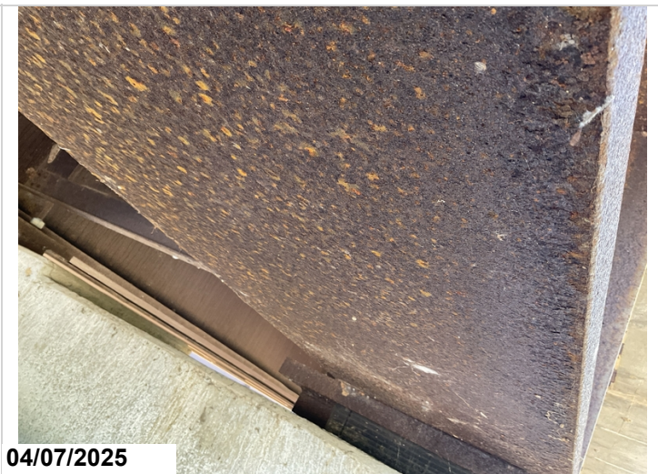
Span 4, girder 1, bent 4, first 10' of bottom flange and lower web has scaly rust 1/4" or less flakes.
