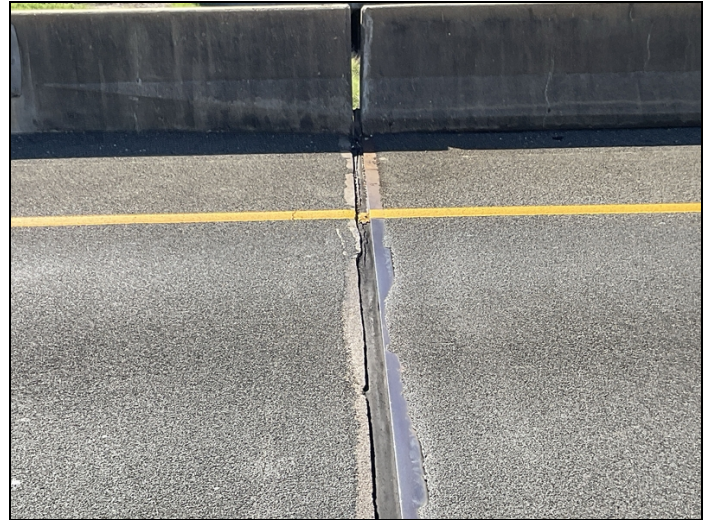
Abutment 2, pourable joint seal, right lane: split.
