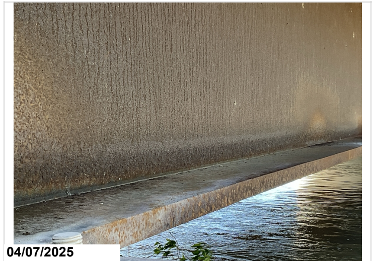
Span 4, girder 1, bent 5 last 10': minor scaling on outside web and bottom flange.
