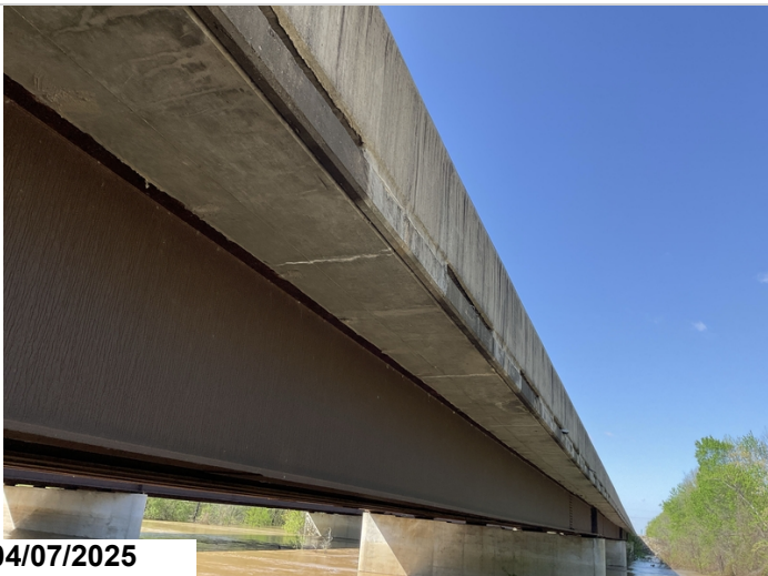
Typical transverse cracking in undersurface of overhang.
