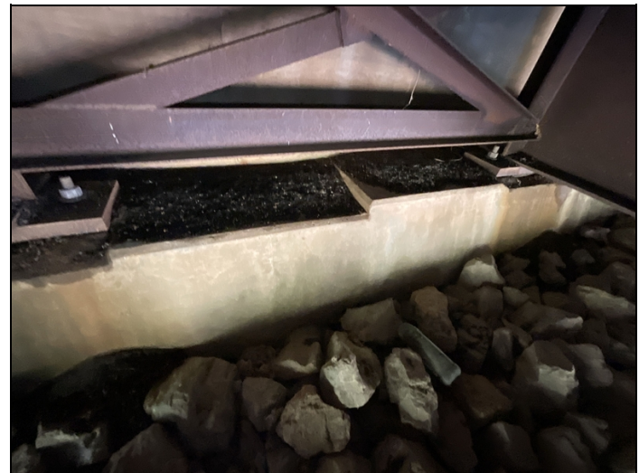
Dirt and debris on abutment caps.
