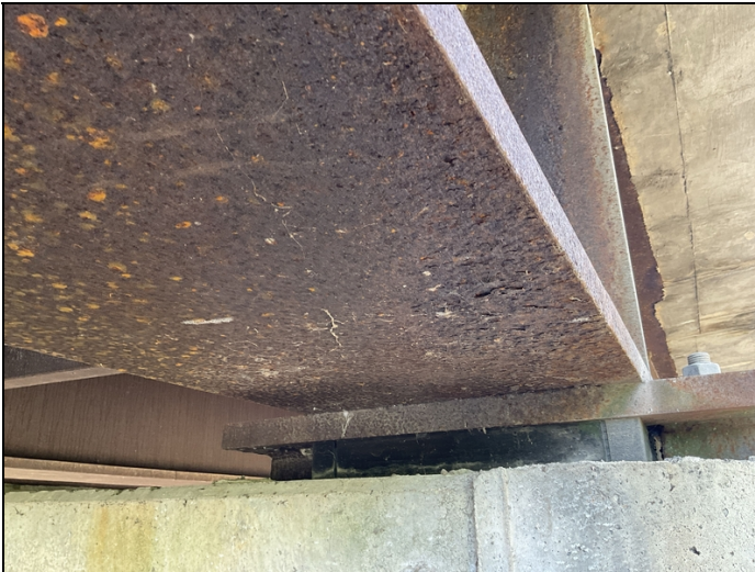
Span 5, girder 1, bent 5, first 3': minor scaling on bottom of bottom flange has minor scaling.
