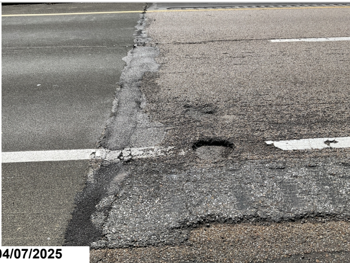
Abutment 1, approach roadway, left lane at white line: 1' spall 2" deep.
