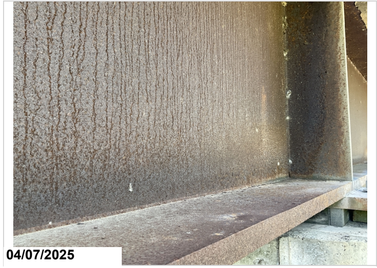
Span 5, girder 1, bent 5, first 3': minor scaling on outside web and bottom flange.
