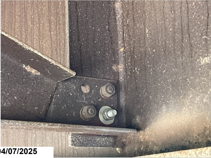
Span 3, bay 2, diaphragm 3: left lower connection bolts loose with one missing and one grade 5 bolt.
