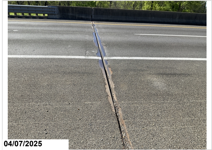
Abutment 2, pourable joint seal.
