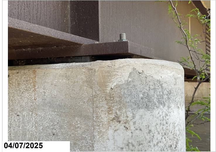
Bent 7, pier wall, left top corner: small area of repair with minor cracks.
