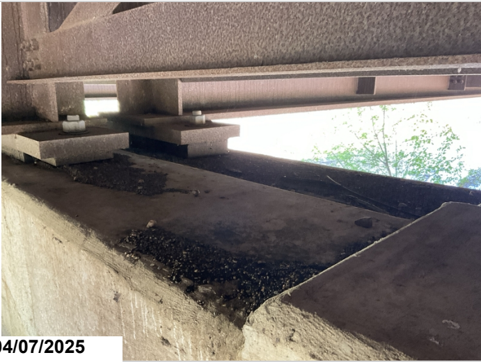
Typical dirt and debris on bent 3 pier cap.
