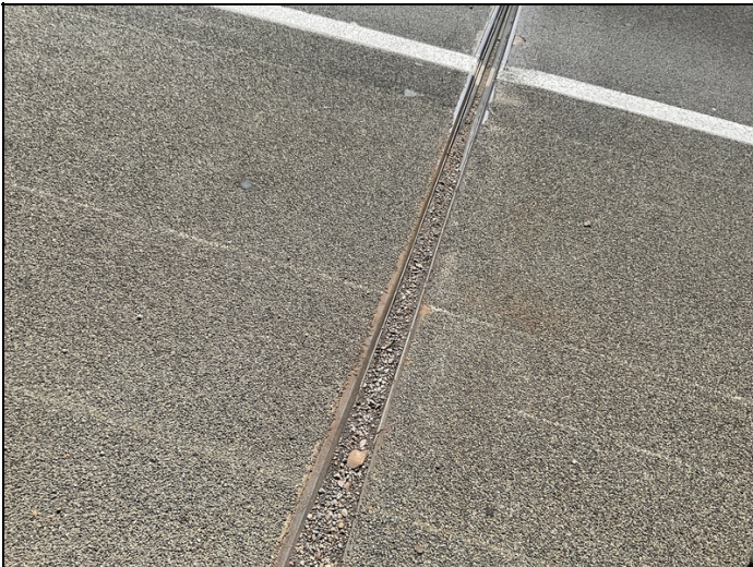
Typical dirt and debris in joint.
