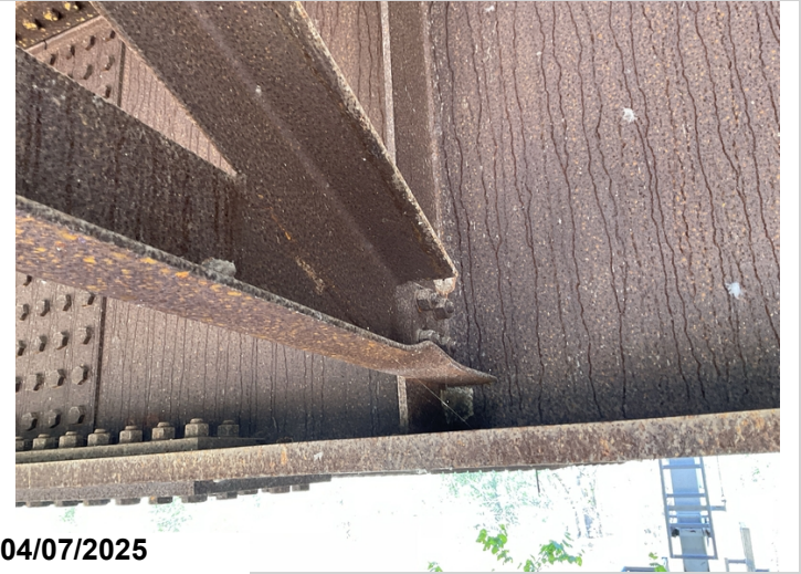
Span 3, right side of girder 3, diaphragm 8 at bottom: dented.
