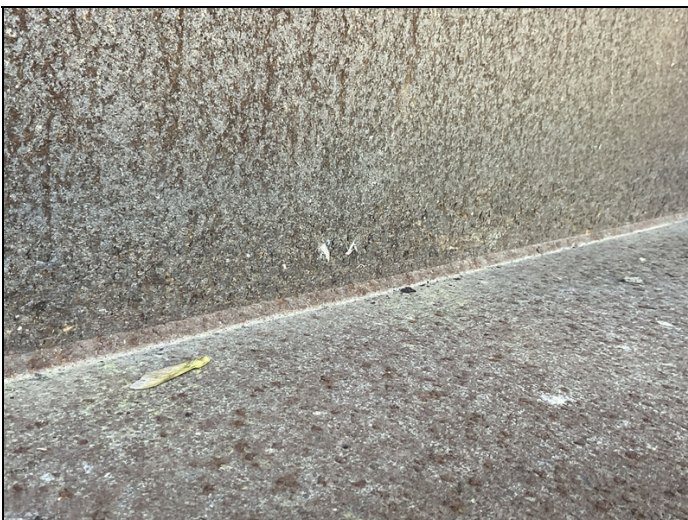
Span 4, girder 1, bent 4, first 10' of bottom flange and lower web has scaly rust 1/4" or less flakes.
