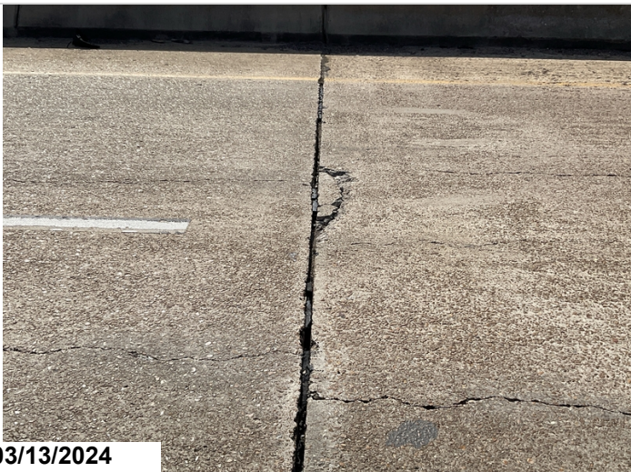
Deck, Span 3, Bent 4, Right Lane: 1' wide by 2' long spall / delaminated area. CS3
