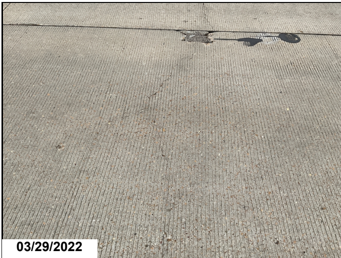
Typical approach slab crack
