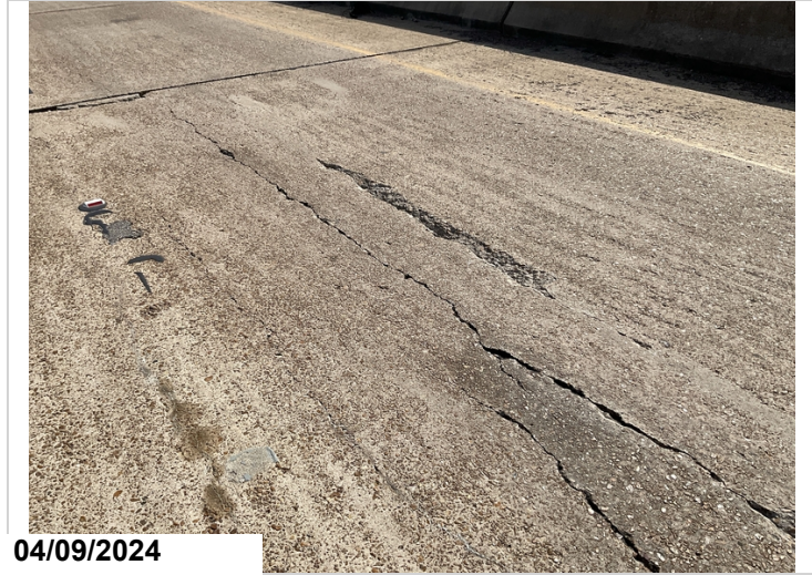
Deck, Span 3, right lane: spalled along crack, typical of left lane.
