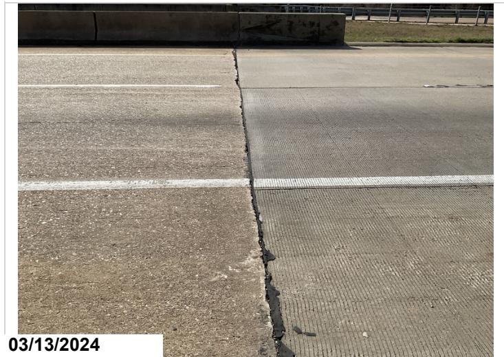
Abutment 1, pourable joint seal, across right travel lane: missing.
