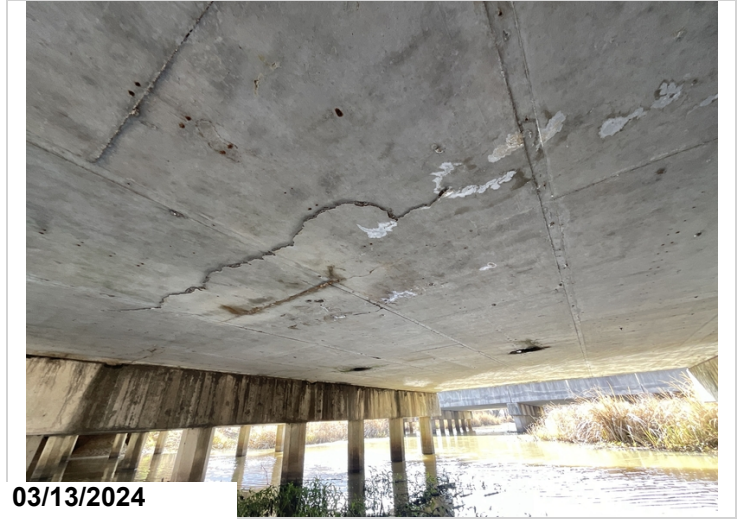
Span 2, soffit / under surface of deck, left side: has 4' wide by 6' long delaminated area
