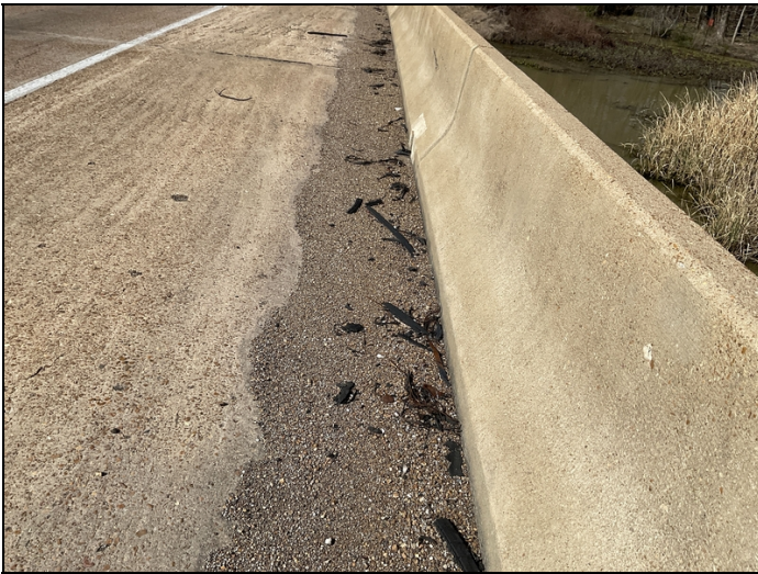
Dirt and debris in gutters
