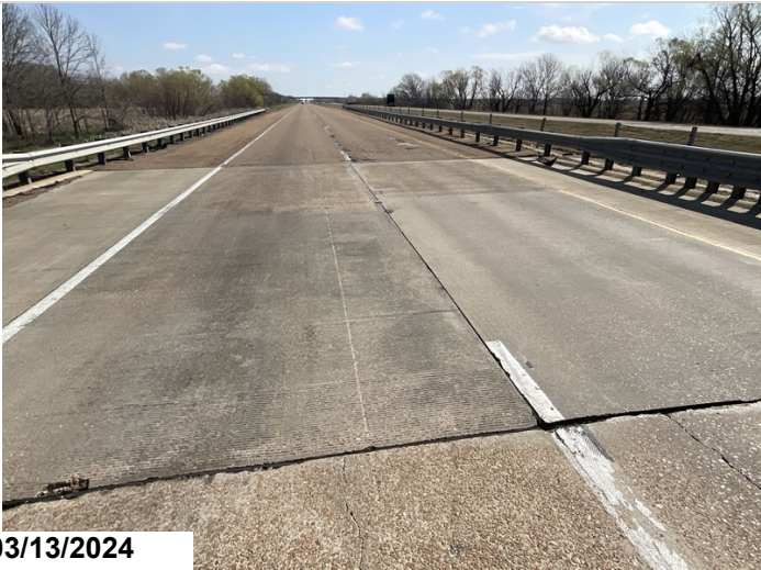
Abutment 2 approach slab
