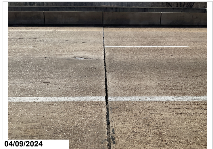
Bent 3, pourable joint seal: Pourable joint seal missing for 30'.
