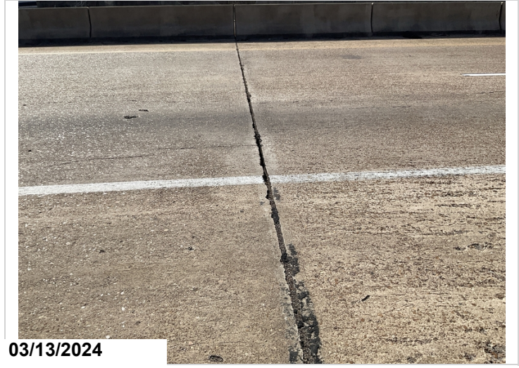
Pourable joint seal, bent 5: pourable joint seal missing across travel lanes.
