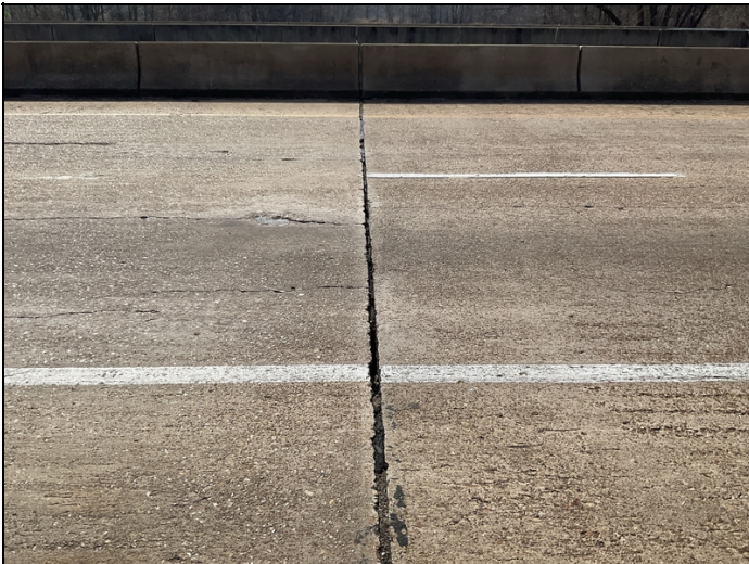
Bent 3, pourable joint seal: Pourable joint seal missing for 30'.
