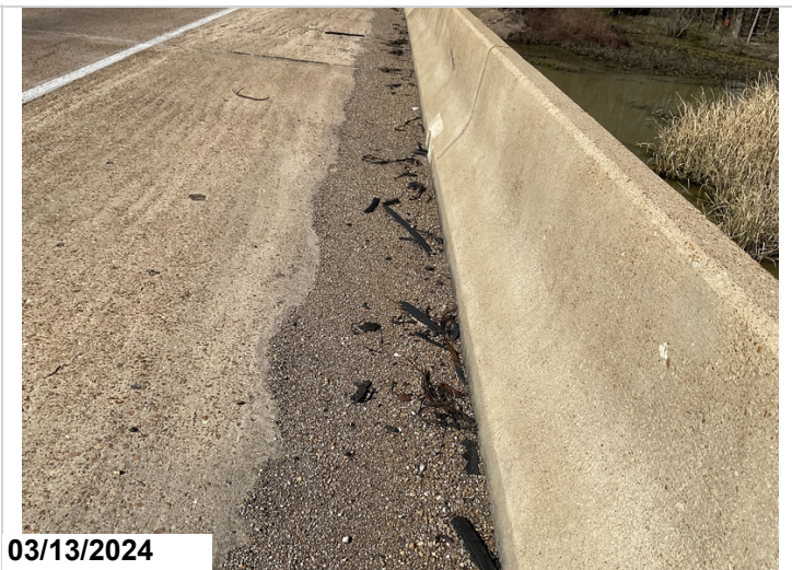
Dirt and debris in gutters
