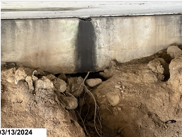
Abutment 1 slope eroded at centerline undermining cap for two feet up to one foot deep.
