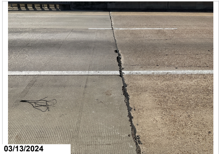
Pourable joint seal, Abutment 2: 16' missing
