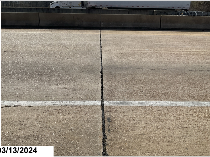
Bent 2, Pourable Joint seal: 15' missing.
