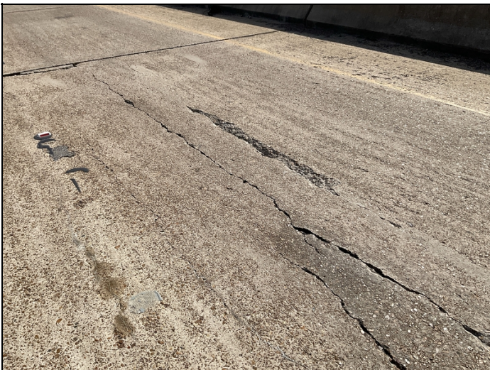
Deck, Span 3, right lane: spalled along crack, typical of left lane.
