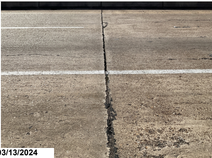
Pourable joint seal, bent 4: pourable joint seal missing across travel lanes.
