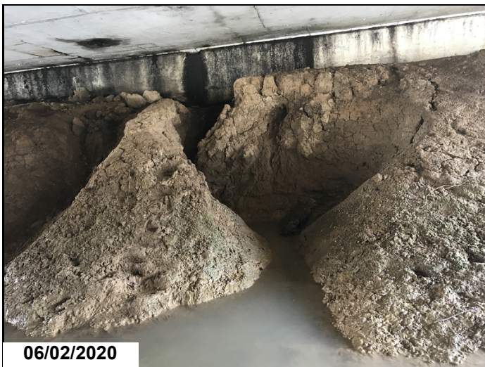
Erosion at abutment 2.
