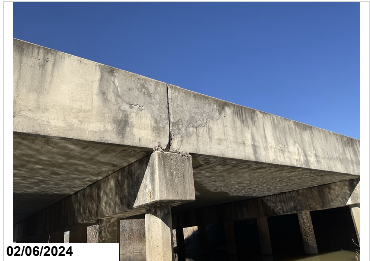
Spans #3 and 4 right bridge rail patched
