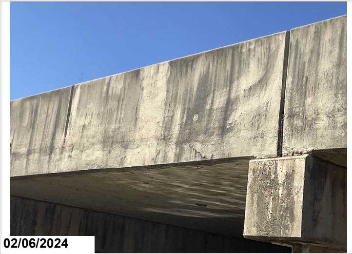
Span #2 right side of slab at bent #3 cracked
