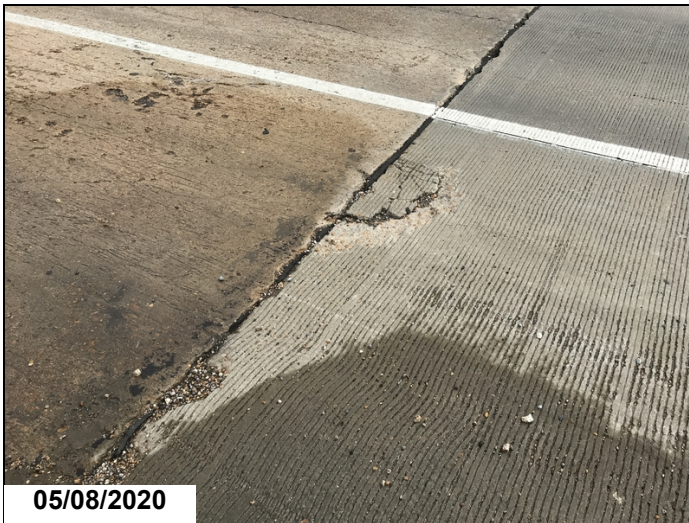
Abutment 1 left approach gutter 1' x 2' delamination and spall.
