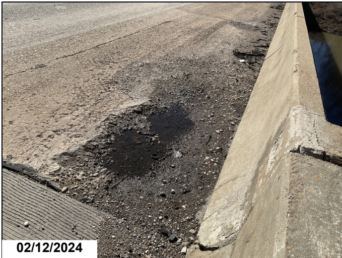
Heavy scaling in span #5 left gutter
