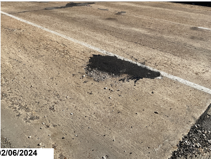
ACHM patch in span #1 left lane
