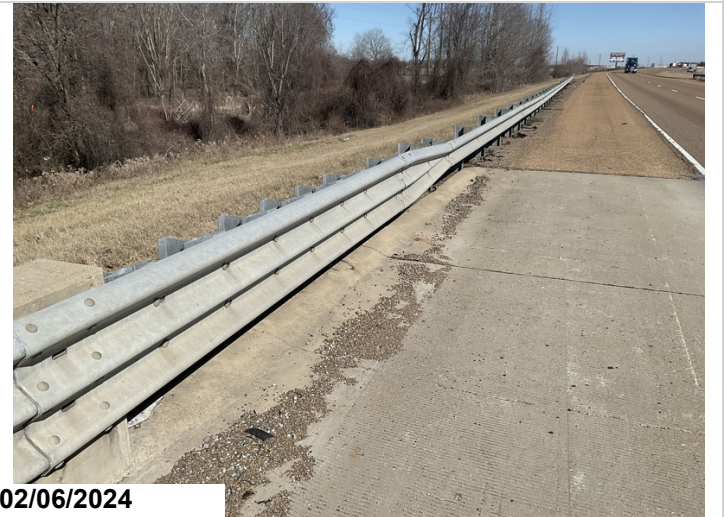
Abutment #2 left approach rail
