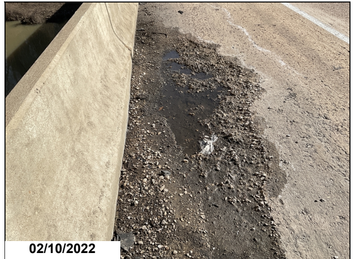
Span #2 left gutter has 36' of heavy scaling.
