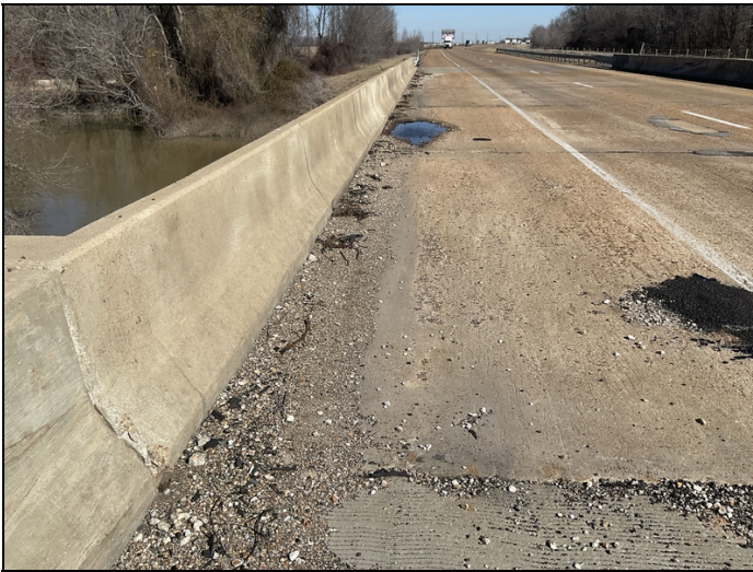
Dirt and debris in gutters
