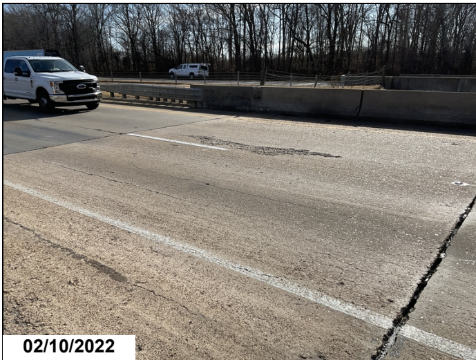
Span #5 right lane has a eight foot shallow spall with no exposed rebar.
