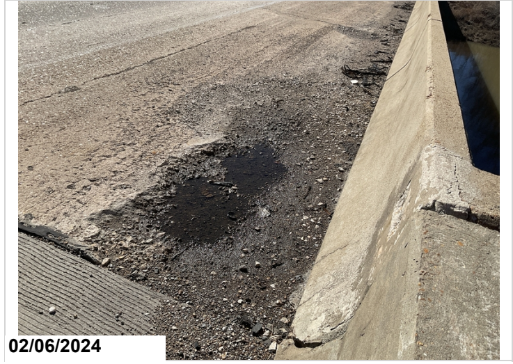
Heavy scaling in span #5 left gutter
