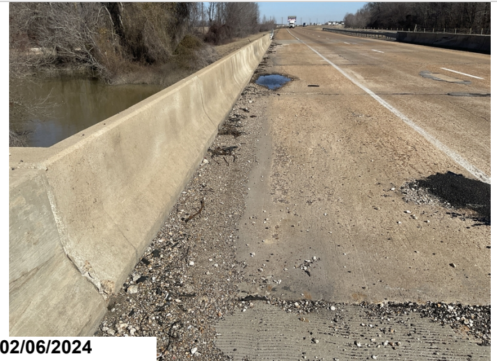
Dirt and debris in gutters
