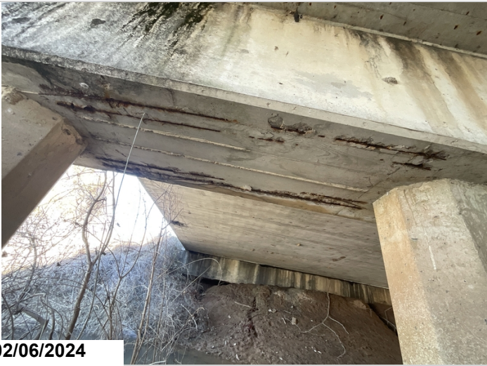
Typical exposed rebar on bottom face of caps
