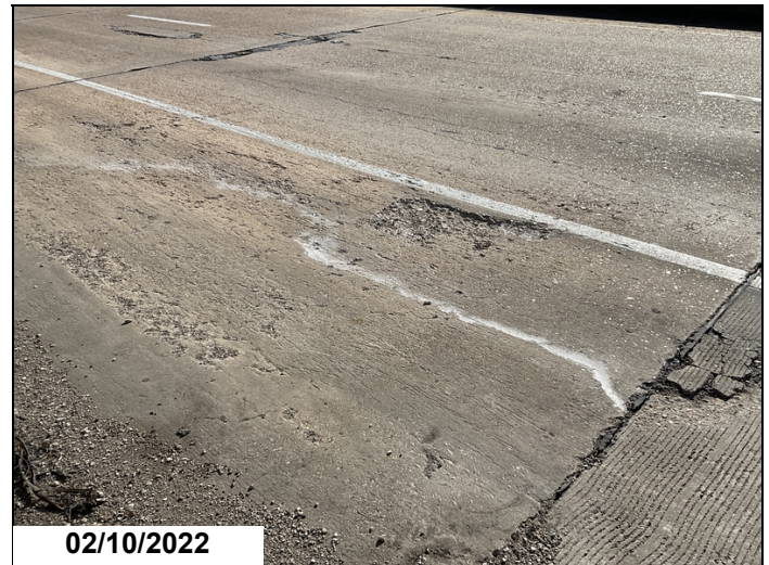
Span #1 left shoulder has two foot spall no rebar exposed.
