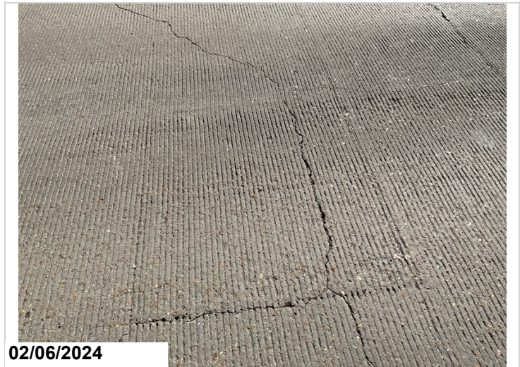
Typical approach slab cracks
