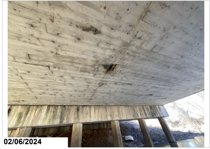
Typical soffit spall with exposed rebar
