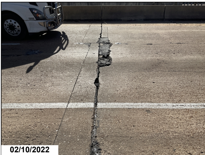
Span #1 has 4 square feet of asphalt repairs with spalling around edges, left lane and a 1'
