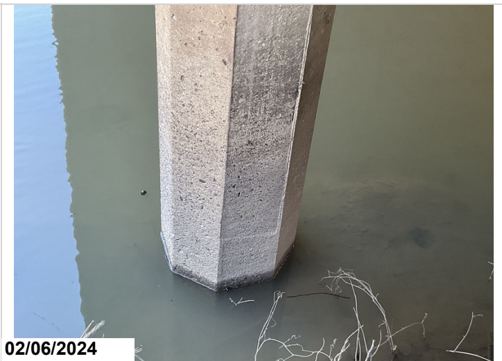
Typical light abrasion on piles
