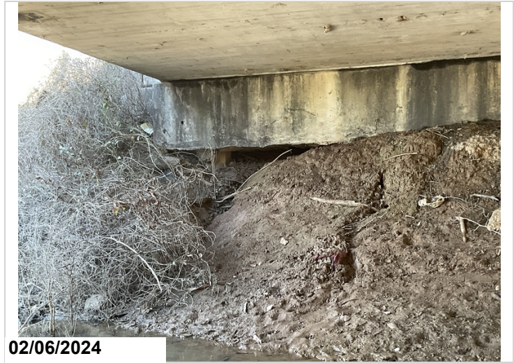
Abutment #2 left side undermined up to one foot for six feet exposing pile #2
