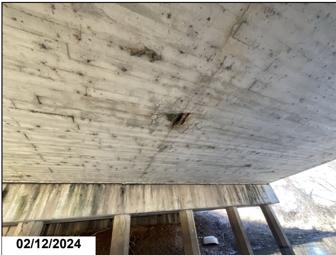
Typical soffit spall with exposed rebar
