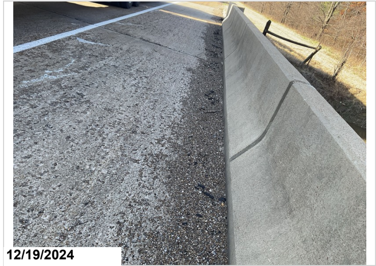
Dirt and debris in gutters
