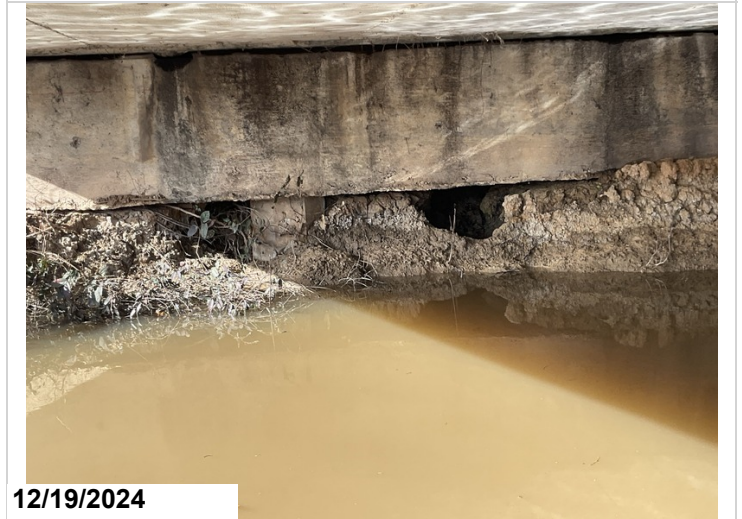
Abutment 1, right side: cap undermined 6' up to 2' deep exposing pile 6.
