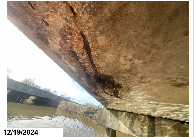
Span 2, undersurface of deck, at right deck drain: spalled at right deck drain with exposed reinforcing steel with moderate section loss, 1' by 3'.
