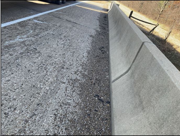
Dirt and debris in gutters
