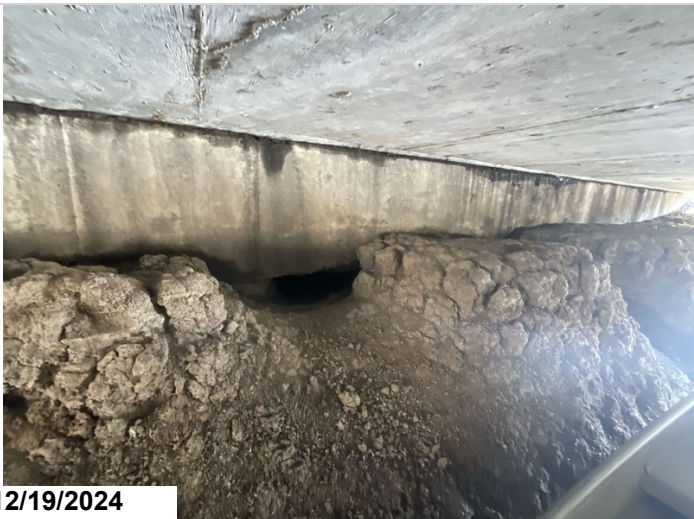
Abutment 2, by pile 3: large animal hole under cap exposing pile 3 up to 1'.
