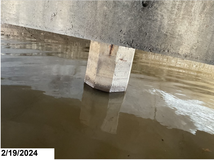
Bent 2, pile 4, at top: two small pieces of exposed reinforcing steel due to poor concrete coverage.
