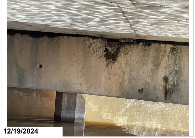
Bent 2, pier cap, back, between piles 6 and 7, at top: spalled with no exposed reinforcing steel.
