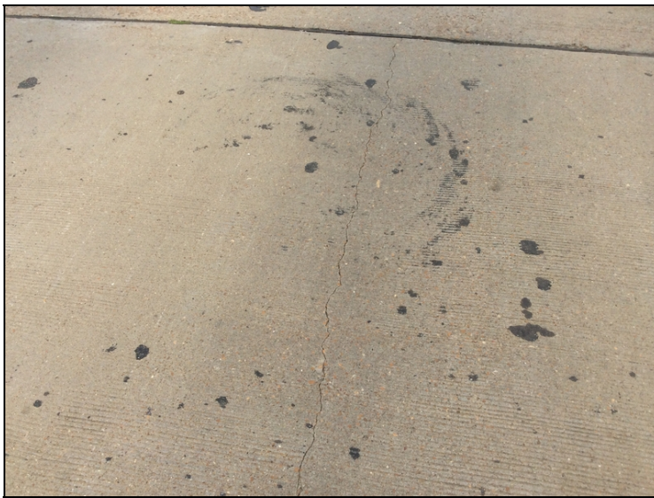
Typical longitudinal deck crack.
