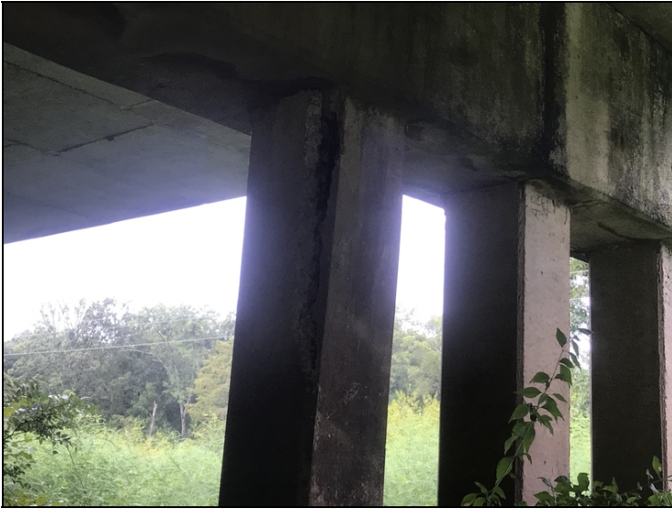
Bent #7 pile #3 is cracked, delaminated and spalled at top with exposed rebar with 5% section loss.
