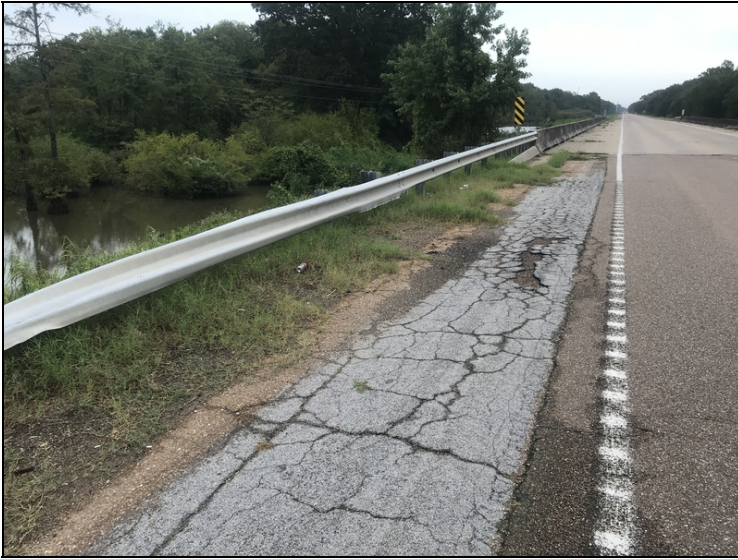
Abutment #1 left approach rail has minor collision damage first two rail posts are damaged and not connected.
