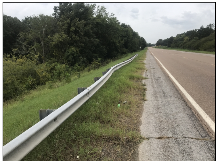
Abutment #1 right approach rail has 40'+- of collision damage 90' +- from bridge end.
