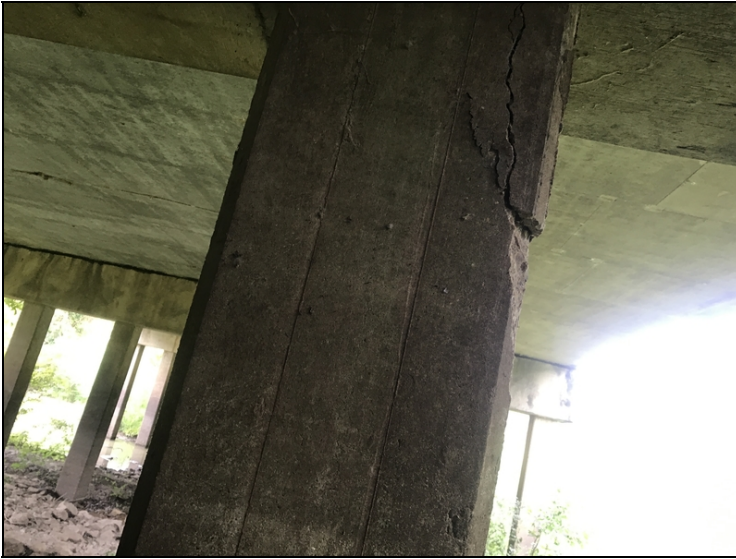
Bent #10 pile #3 is cracked, delaminated and spalled at top with exposed rebar with 5% section loss.
