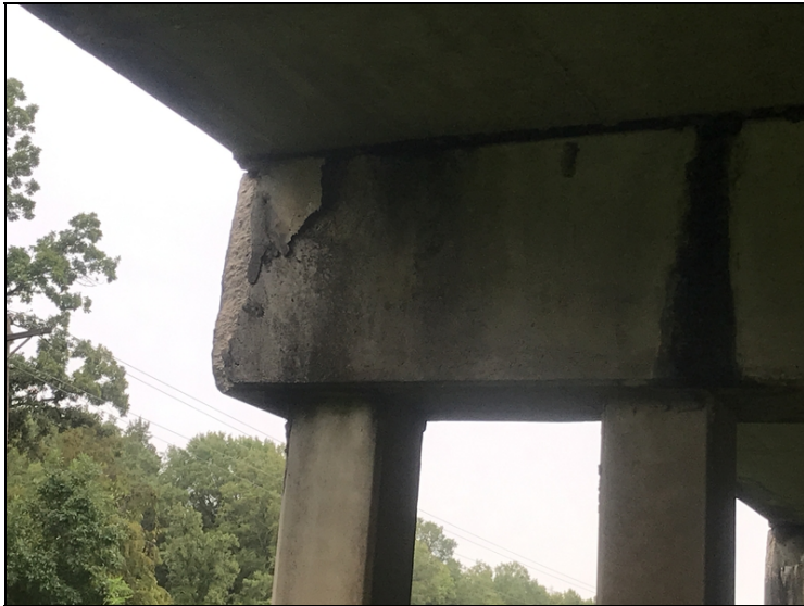
Span #7 cap left side back face spalled and delaminated.
