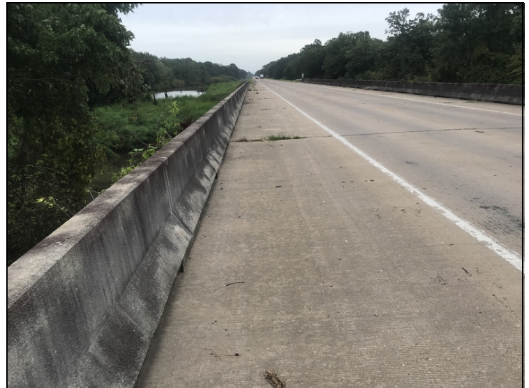
Vegetation growing in gutters at joints.
