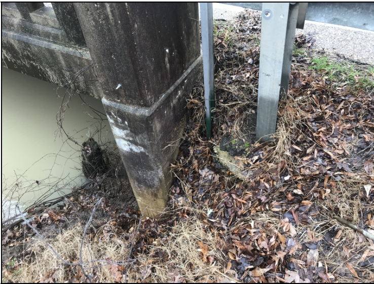
Erosion at abutment 1 left side.
