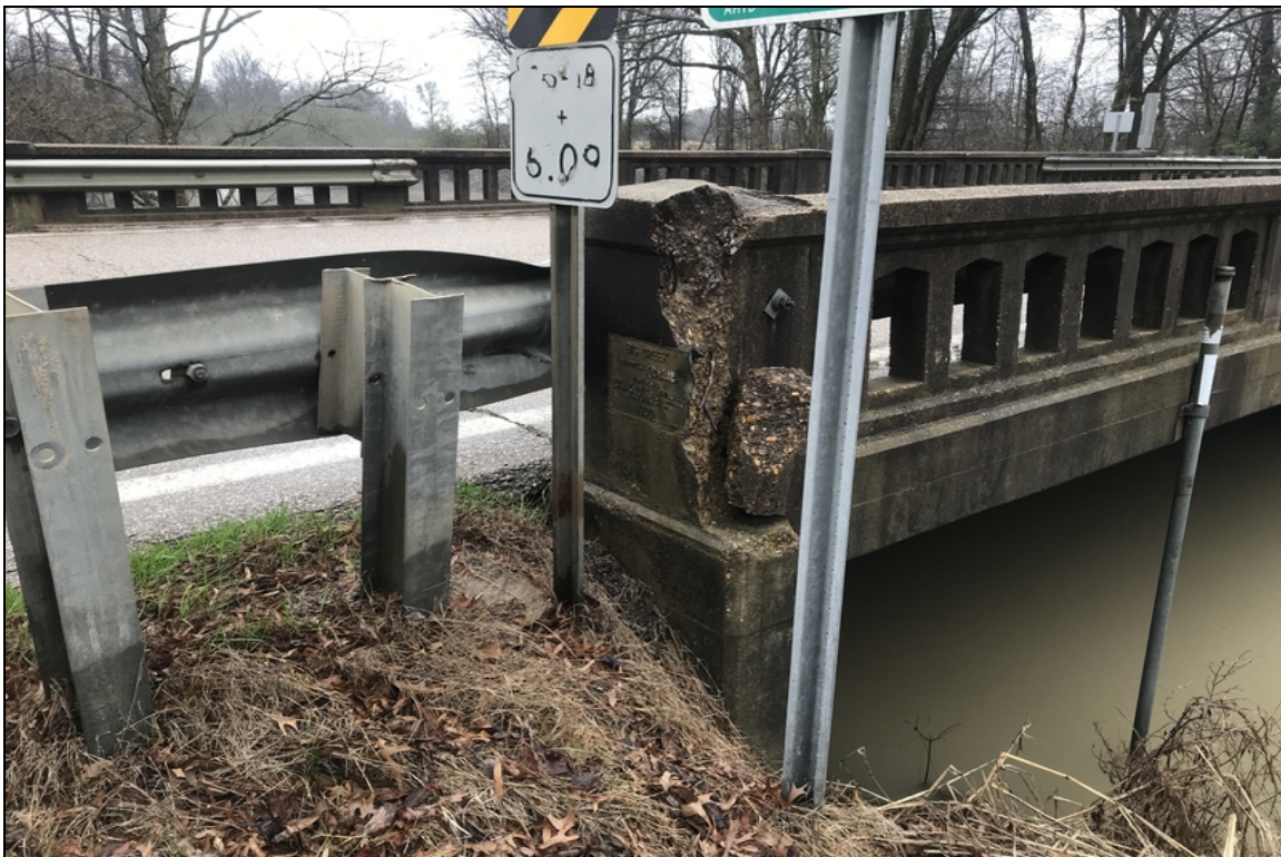
Abutment 1 right monument post damage.
