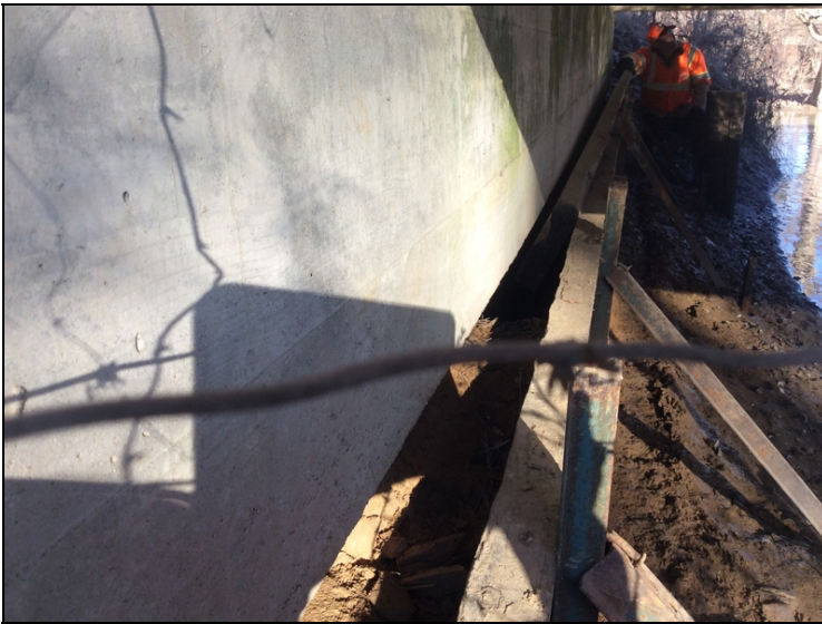
Abutment #1 is undermined behind wood abutment several feet.
