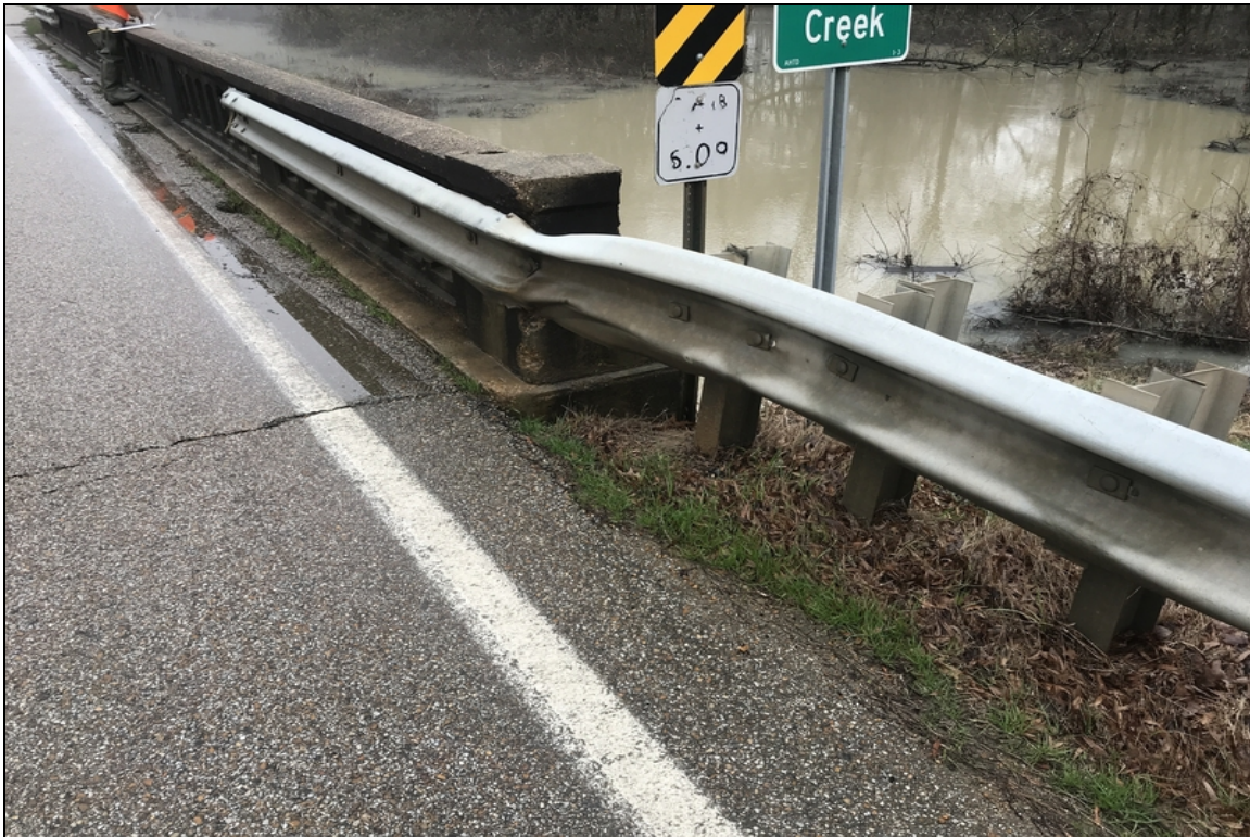
Right approach rail damage at abutment 1.
