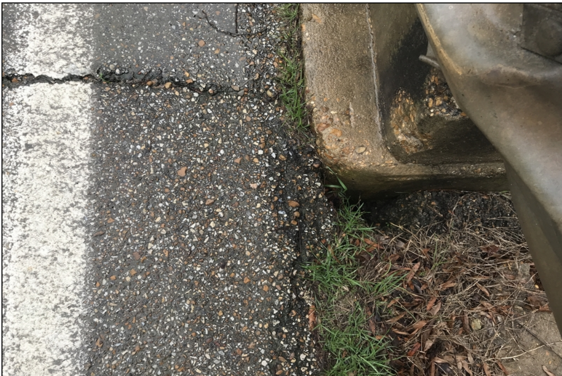
Hole in shoulder at abutment 1 right side.
