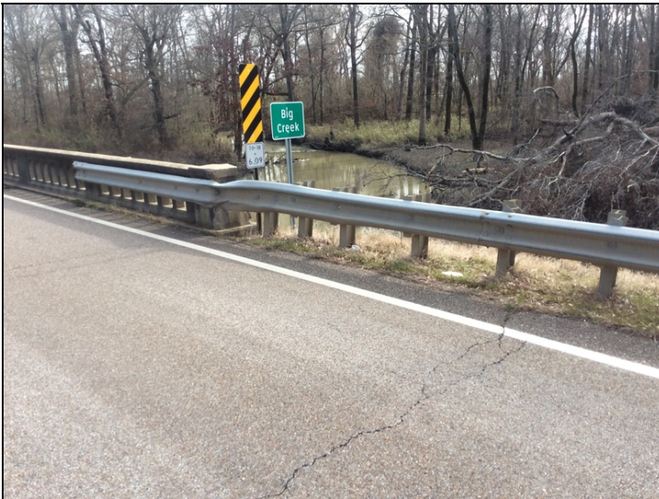
Abutment #1 right approach rail damage.
