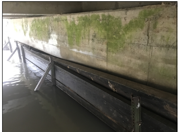
Top board of abutment 1 timber abutment has fallen down.
