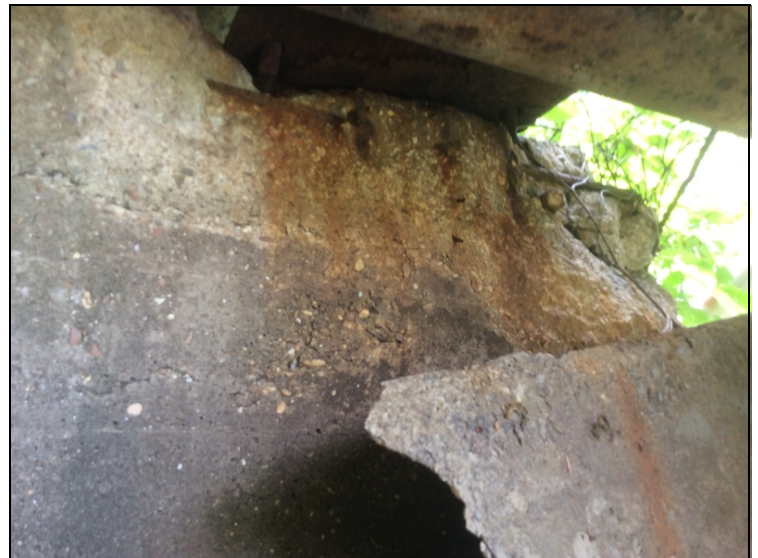
Bent #8 front face has a two foot spall at top right side under bearing of girder #6 with exposed rebar with 5% section loss and 50% loss of bearing.
