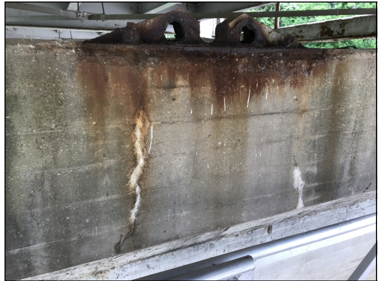
Bent #7 cap back face in center has two cs2 vertical cracks with light efflorescence.
