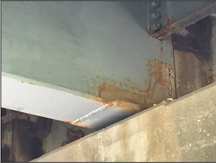
Span #2 girder #3 bent #2 has a L shape t-splice one foot long.
