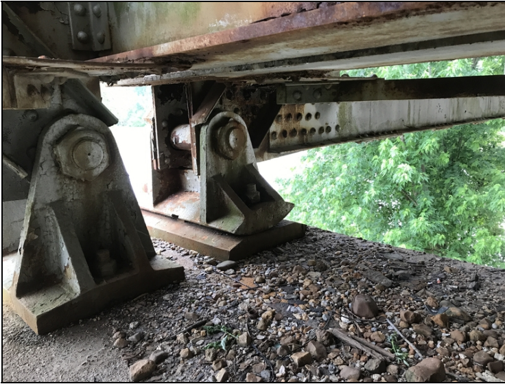
Typical movable bearing truss.
