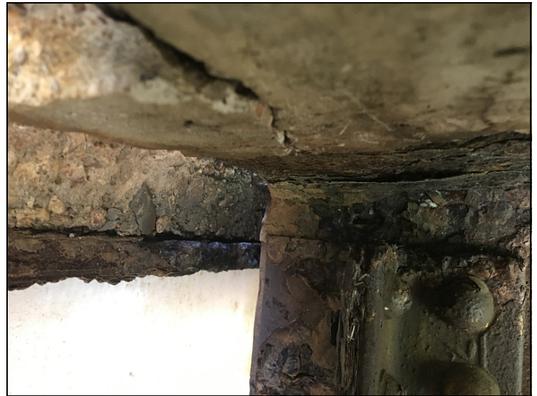
Span #2 girder #3 bent #3 has half inch hole above diaphragm connection and 60% section loss below diaphragm connection.
