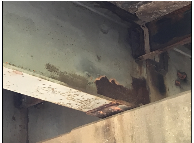
Span #2 girder #4 bent #2 has a L shape t-splice one foot long.
