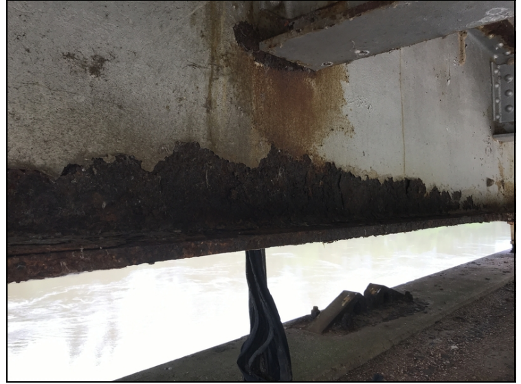
Span #4 at bent #5 floor beam #9 lower flange has corrosion with laminations full length leading into lower web with up to 20% section loss.
