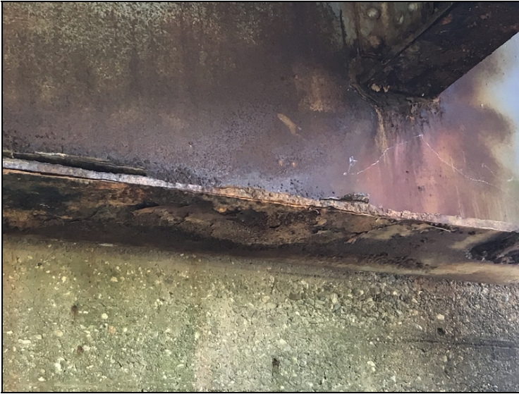
Span #3 at bent #3 floor beam #1 has heavy corrosion full length top and bottom flanges with areas of section loss up to 60%.
