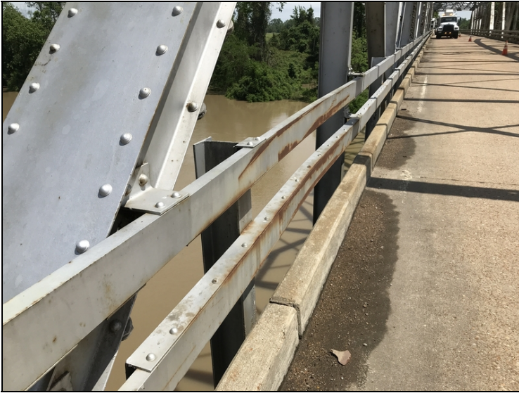
Span #5 left rail damage near bent #5.
