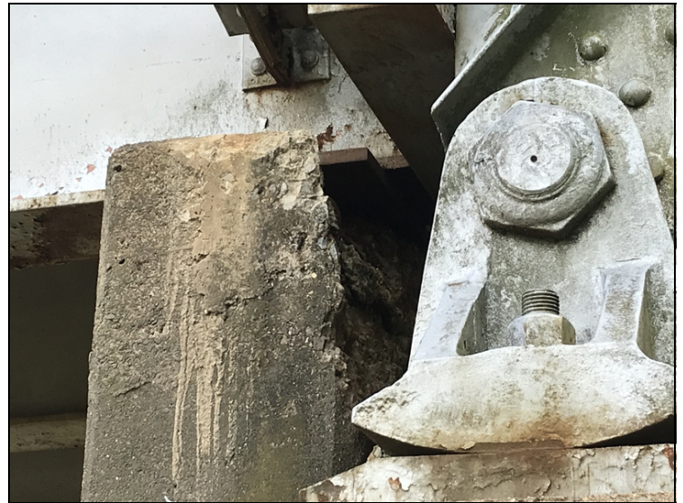
Bent #3 cap right side has large spall exposing bearing plate for span #2 girder #6.
