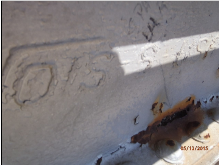
Span #5 right side of bridge at vertical location L4 lower outside web of bottom chord has area with a hole in web.
