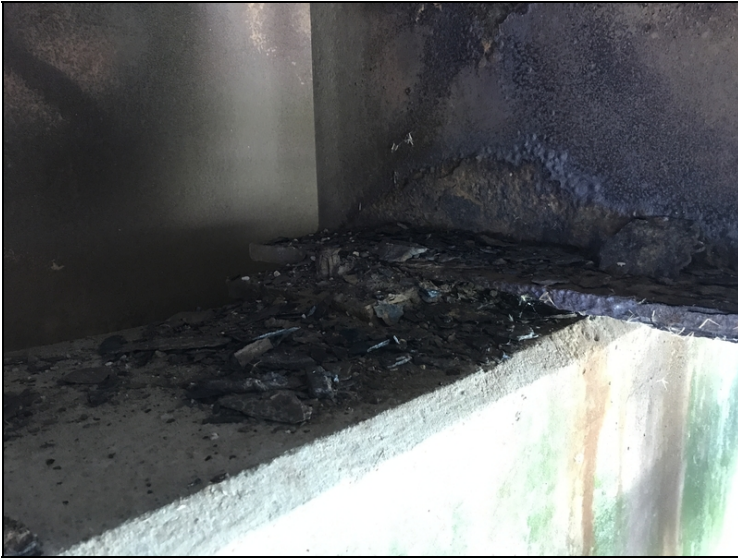
Span #8 girder #3 at bent #8 lower flange first two feet has areas of section loss up to a knife edge.
