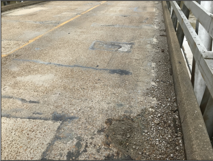
Span #4 right lane 3/4 span has four one foot spalls no rebar exposed.
