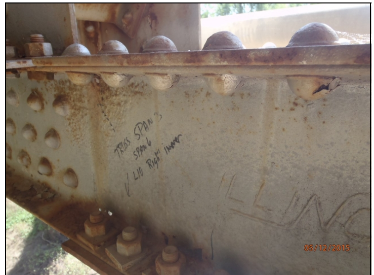
Span #6 right side of bridge at vertical L10 upper and lower inside web of bottom chord has areas of holes rusted through.
