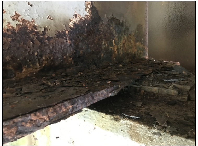
Span #8 girder #4 at bent #8 lower flange first two feet has areas of section loss up to a knife edge.
