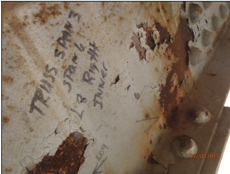
Span #6 right side of bridge at vertical L8 lower inside web of bottom chord has holes rusted through.
