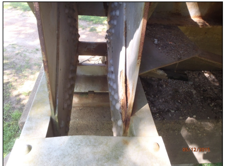
Gusset plate span #3 right L0 connection.
