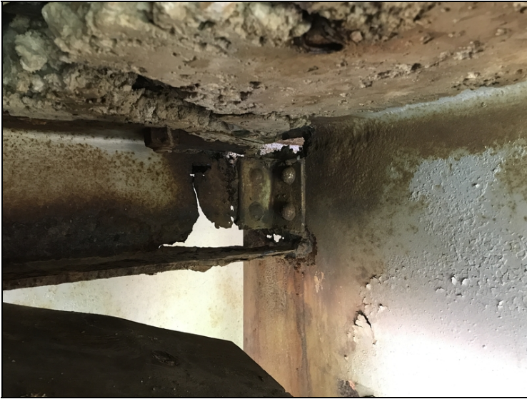
Span #2 girder #2 bent #3, girder has 6" long x 1 1/2" hole in web at top flange at end of girder and a 2" long x 1" tall hole in web below diaphragm connection.
