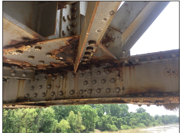
Span #5 right side of bridge at vertical L2 lower inside web of bottom chord has holes rusted through bottom hole is 7" long top hole is size of a dime.
