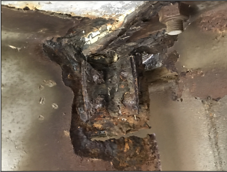
Span #8 girder #4 at bent #8 has a two inch long hole in web above diaphragm and a six inch hole below diaphragm.
