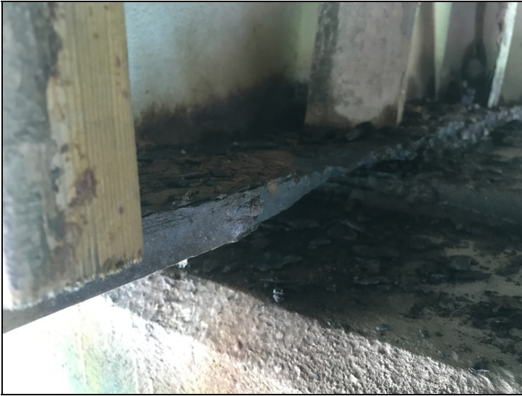
Span #2 girder #3 at bent #3, 1' from end of girder has 6" long area across bottom flange original thickness .850" remaining .260".
