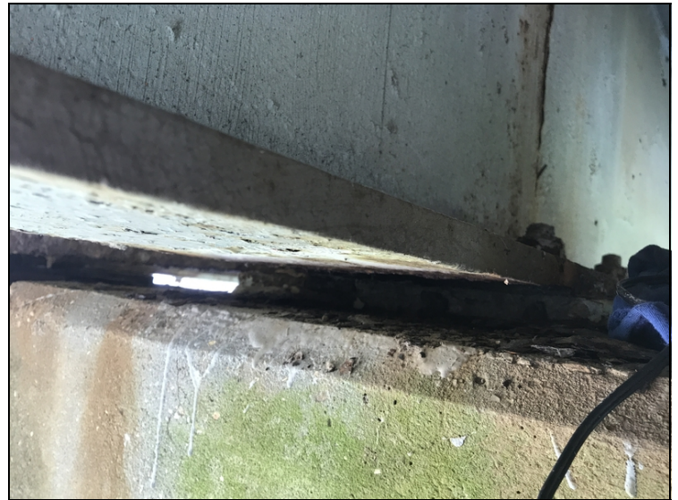
Span #2 girder #5 at bent #2, 1' from end of girder has a 4" long area across bottom flange original thickness .850" remaining .575".
