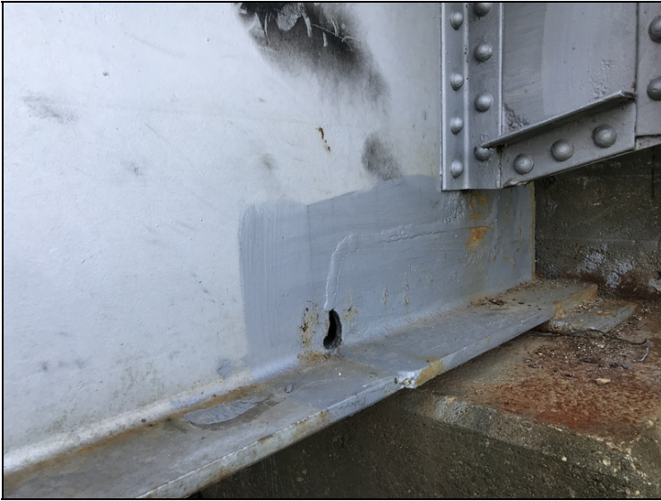
Span #1 girder #1 bent #1 has a t-splice first two feet by seven inches tall.
