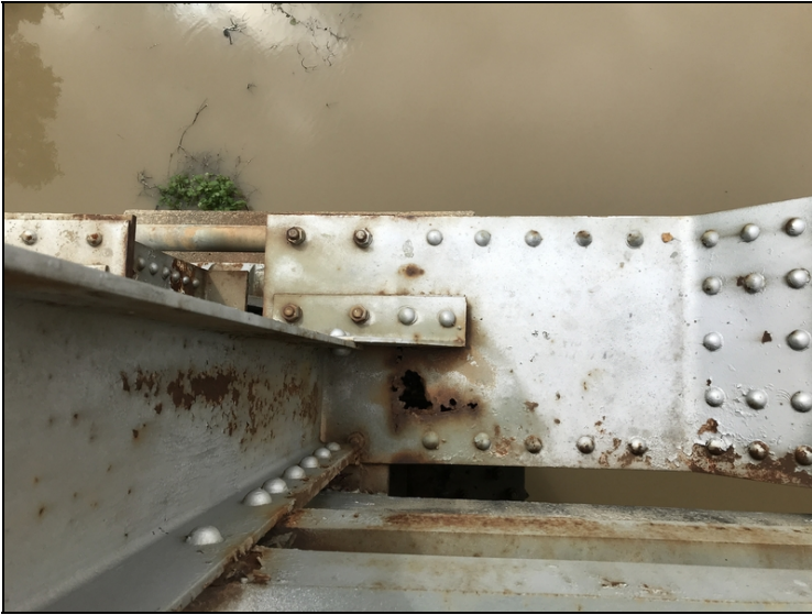
Span #6 right side cover plate at bent #7 L12 connection.
