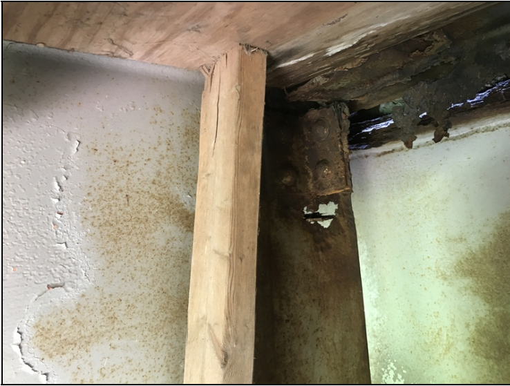
Span #2 girder #4 bent #3 has 3" long x 1 1/2" tall hole in flange below diaphragm connection.
