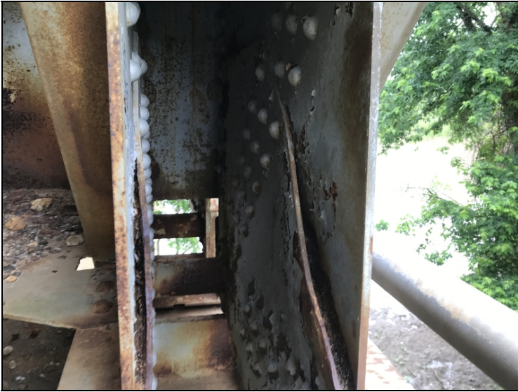
Gusset plate span #3 right side at bent #4 L8 connection
