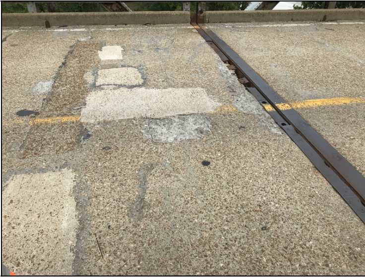
Span #3 both lanes at bent #4 has multiple spalls.
