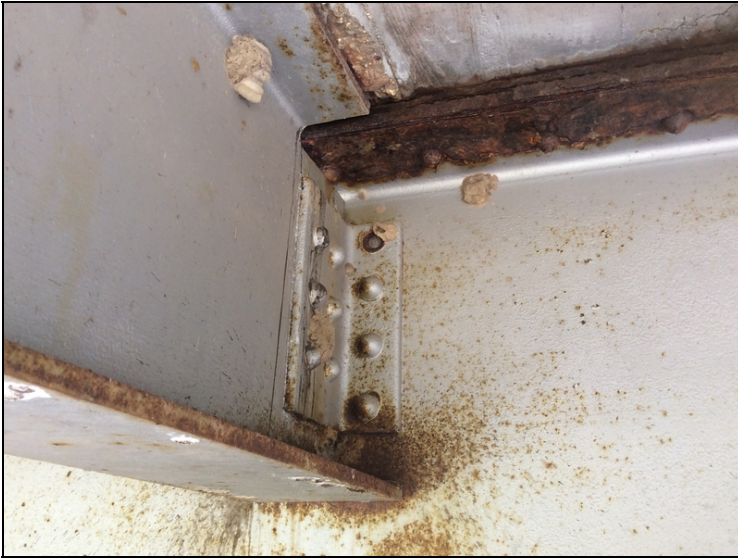
Bent #5 span #4 stringer #4 has right side top rivet sheared off.
