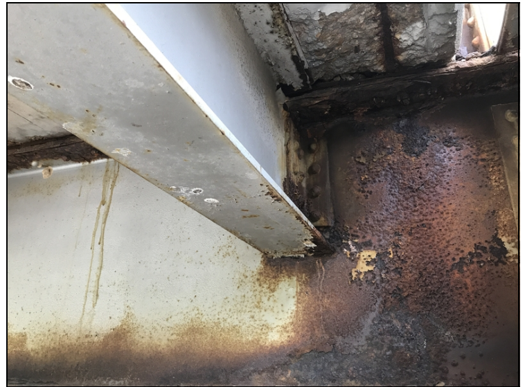
Span #4 at bent #5 floor beam #9 right side first two feet top flange has areas of section loss up to 70% leading into web with section loss up to 20%.
