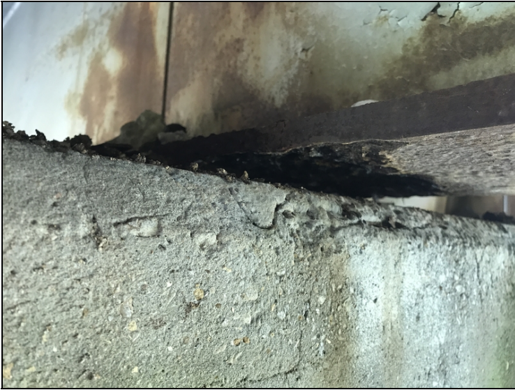
Span #1 girder #3 at bent #2 1' from end of girder has 5" long area across bottom flange original thickness .850" remaining .272".
