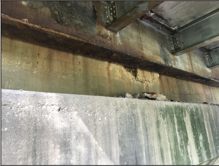
Bent #3 cap center ahead face has three foot delaminated area with two foot spall exposed rebar with 10% section loss.
