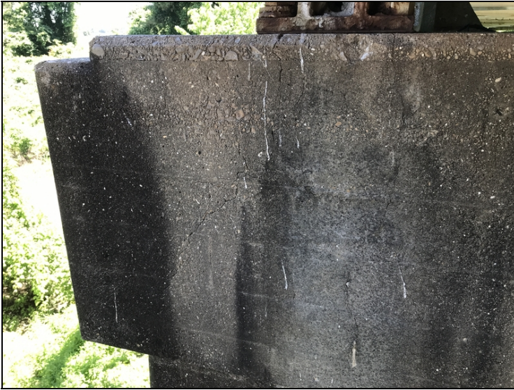
Bent #7 cap back face left side has some cs2 cracks under bearing.
