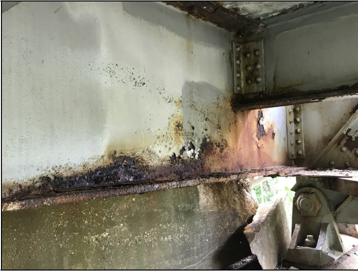
Span #7 floor beam #9 right end for three feet lower flange into web has corrosion with laminations and section loss up to 50%.
