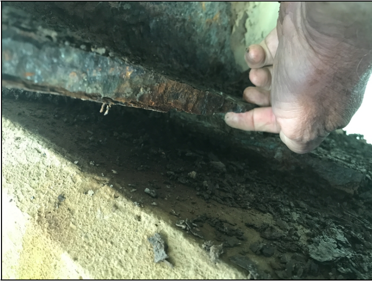
Span #2 girder #2 at bent #2 1' from end of girder has 5" long area across bottom flange original thickness .850" remaining .183", next 2' has .750" remaining
