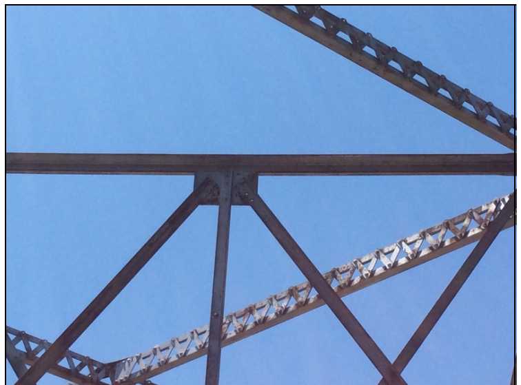
Span #5 3rd cross brace in upper truss top angle brace over left lane has two missing rivets.
