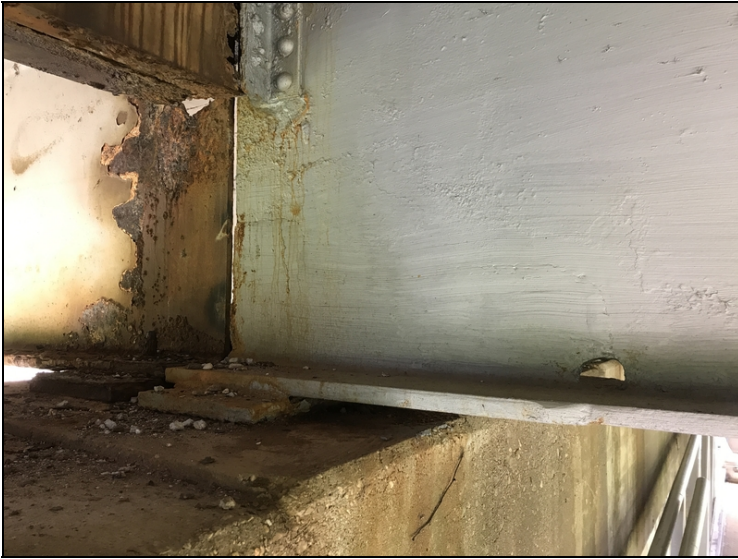
Span #8 bent #9 girder #2 has a t-splice that is two foot long by eight inches tall.
