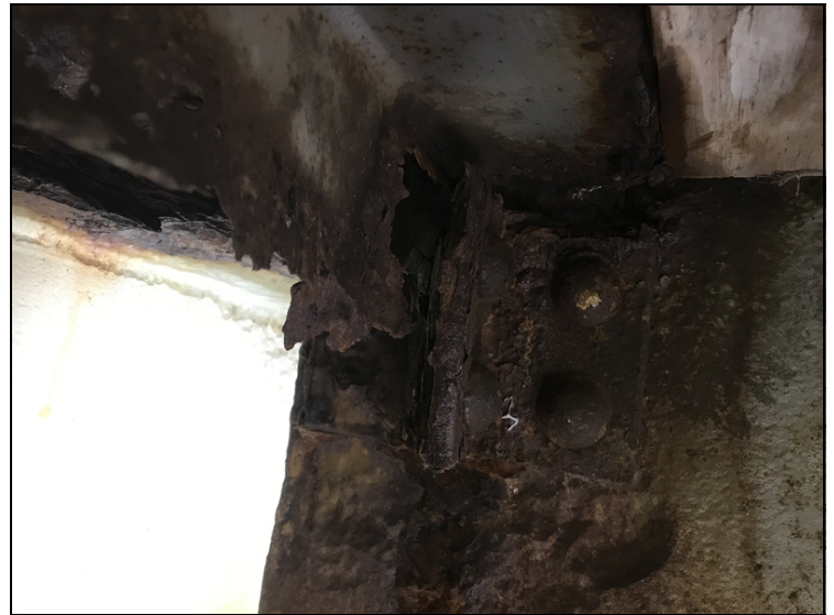
Span #2 girder #5 bent #2 has 1" hole in web above diaphragm connection and a pin hole below diaphragm connection.
