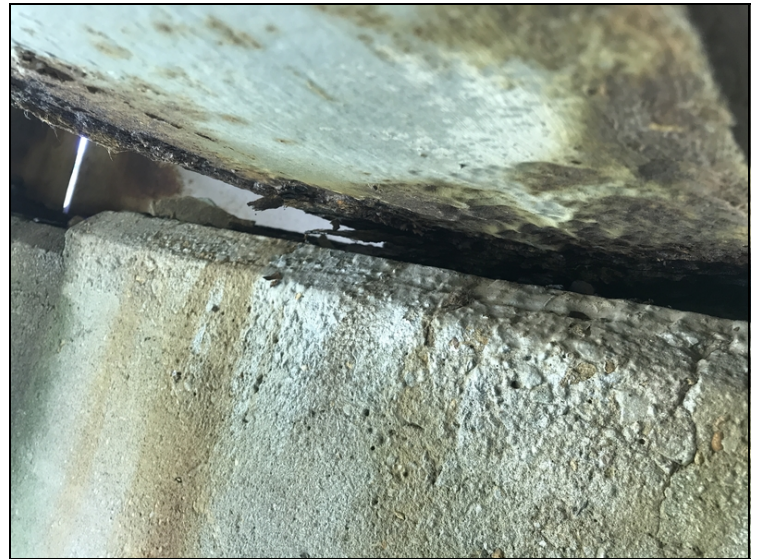
Span #1 girder #2 at bent #2 1' from end of girder has 5" long area across bottom flange original thickness .850" remaining .520".
