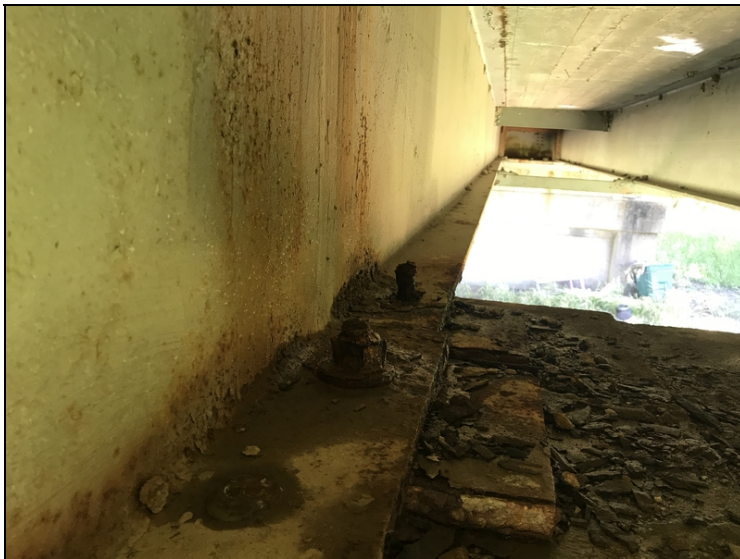
Span #2 girder #4 right anchor nut rusted off.
