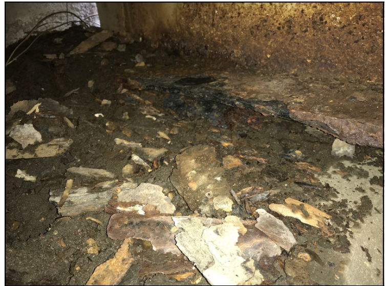
Span #1 girder #2 bent #1 first 1' bottom flange original thickness .850" remaining .309"
