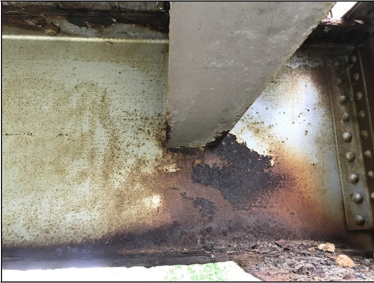
Span #3 at bent #4 floor beam #9 bottom flange right side of bridge at x bracing connection has section loss up to 50%.
