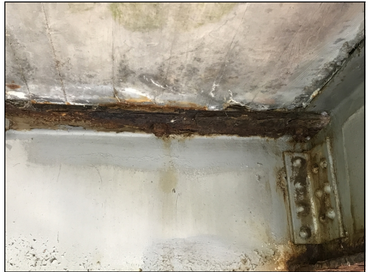
Span #7 floor beam #9 on ends for four feet top flange has corrosion laminations and section loss up to 50%.
