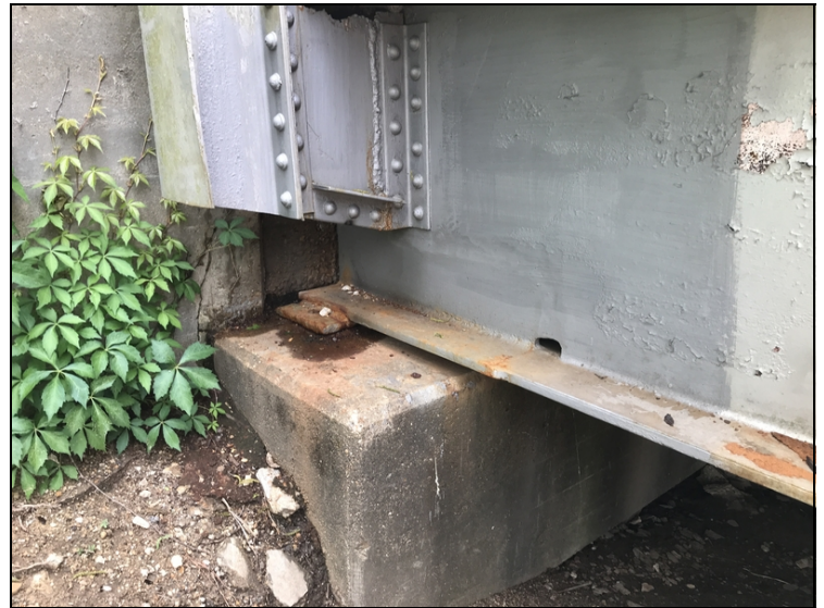
Span #9 girder #1 abutment #2 has been t-spliced two foot long eight inches tall.
