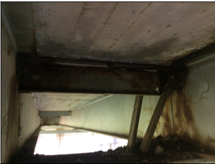
Typical approach spans diaphragms Spans #1,2,8,9
