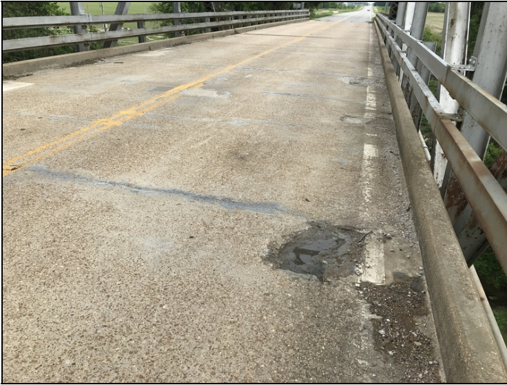
Span #7 right side at gutter spalls.
