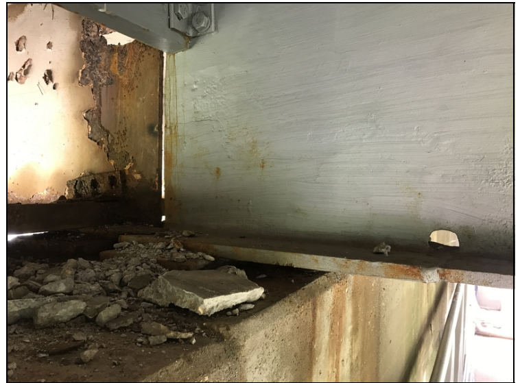
Span #8 bent #9 girder #3 has a t-splice that is two feet long by ten inches tall.
