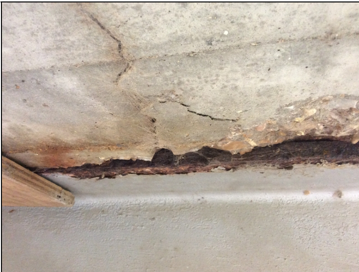
Top flanges of girders in approach spans last three feet of girder ends have corrosion with up to 30% section loss.
