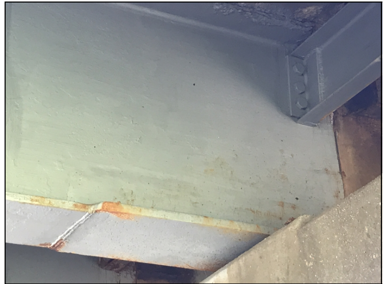
Span #2 bent #2 girder #2 has an L shape t-splice two foot long.
