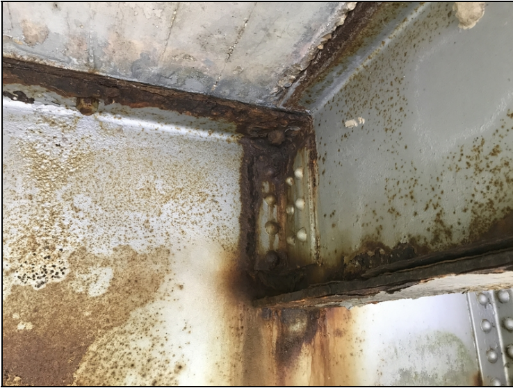
Bent #4 span #4 stringer #1 bottom flange last 3' has up to 20% section loss.
