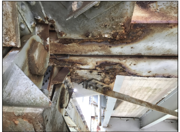
Typical bottoms of floor beam #1,9 spans #3,4,7 on ends at connections.
