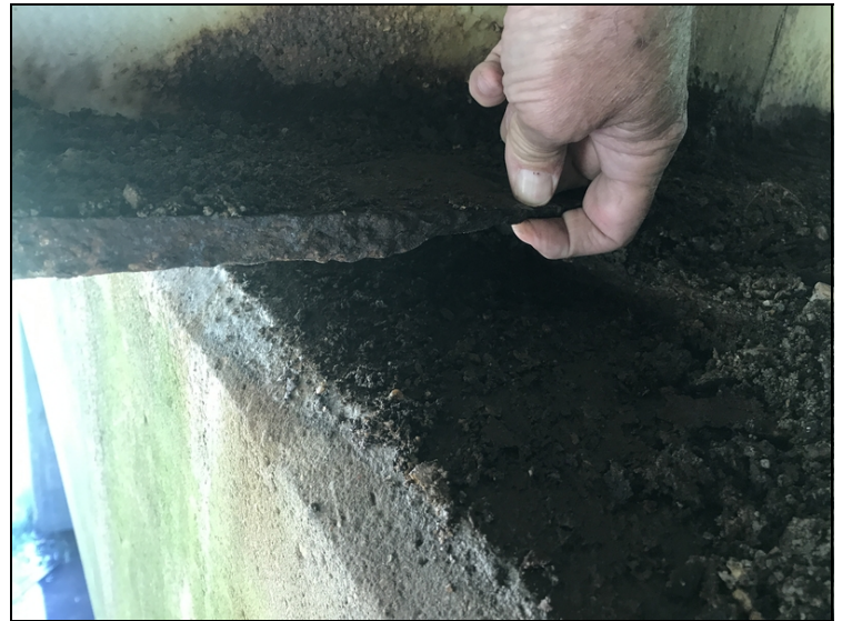
Span #2 girder #3 at bent #2 1' from end of girder has 5" long area across bottom flange original thickness .850" remaining .250".
