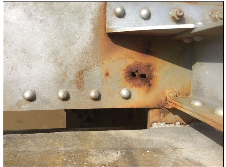
Span #5 cover plate on lower chord right side of bridge at L0 connection has holes rusted through with cracks staring to propagate.
