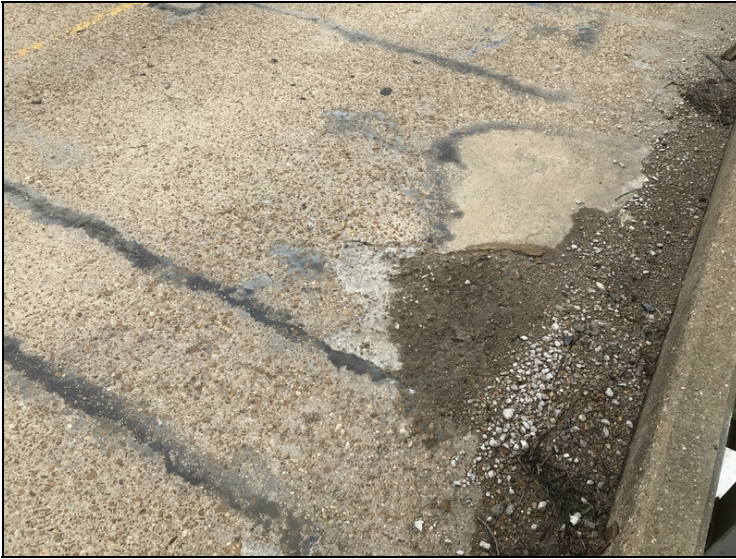
Span #3 right lane 1/2 span has two foot spall no rebar exposed.
