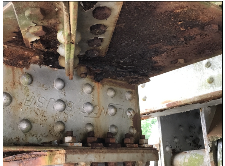
Span #6 left side end of truss at bent #7 lower cord and connection plate to floor beam and x brace has section loss up to 70% at connection of top flange of lower cord and connection plate.
