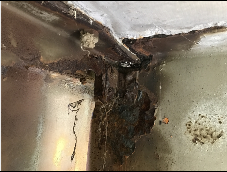
Span #8 bent #8 girder #5 has a three inch hole in web above diaphragm.
