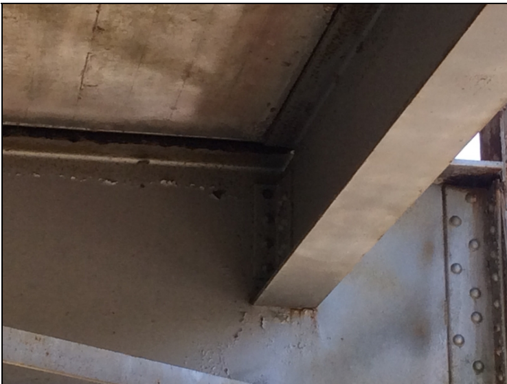
Span #7 floor beam #1 stringer #3 right ahead side top rivet sheared off.
