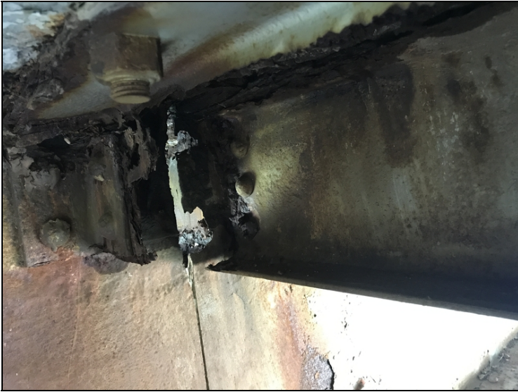
Span #2 bent #2 girder #2 has an 1 1/2" x 6" area of 100% section loss on the end at top.
