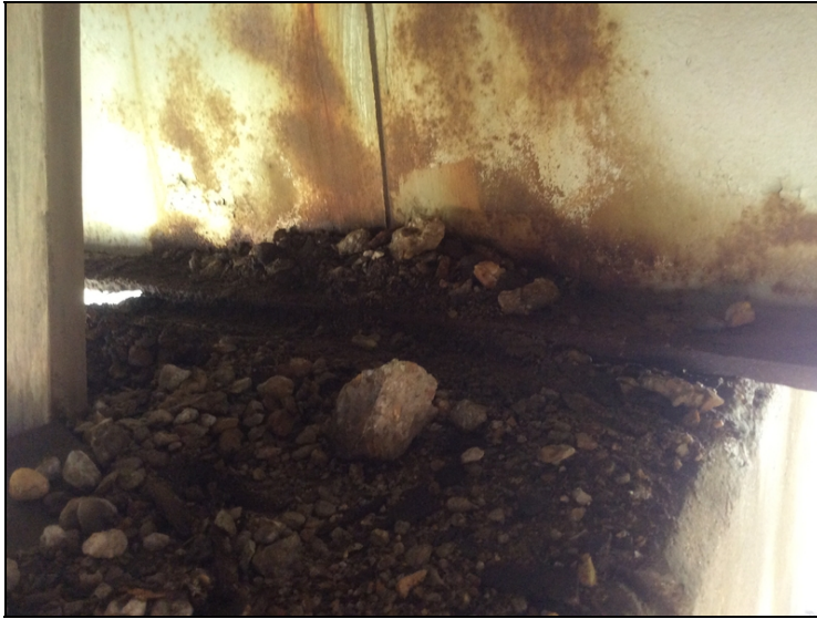
Bent #2 girder #3 span #1,2 lower flange for first foot has section loss up to 70%.
