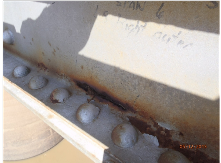
Span #6 right side of bridge at vertical location L8 lower outside web of bottom chord has area of hole in web.
