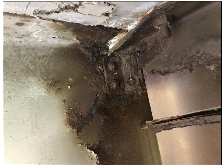
Span #8 girder #2 at bent #8 has a two inch hole in web above diaphragm.
