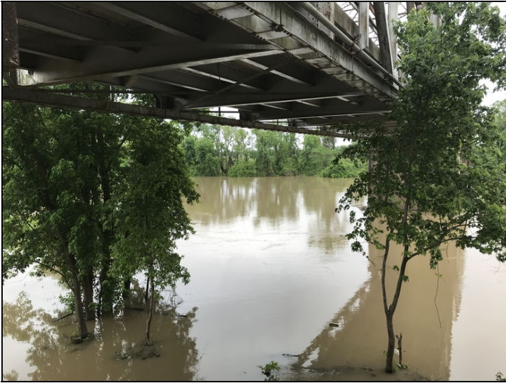
Typical vegetation growing beside and onto bridge hindering access to inspection.
