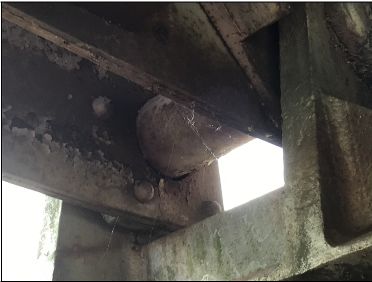
Typical wear in pins to bearing connection on truss.
