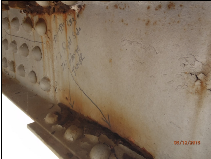
Span #5 right side of bridge at vertical location L2 lower inside web of bottom chord has area of hole in web.
