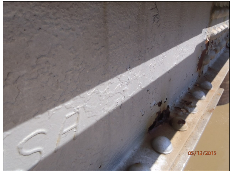
Span #5 right side of bridge at vertical location L2 lower outside web of bottom chord has area of hole in web.
