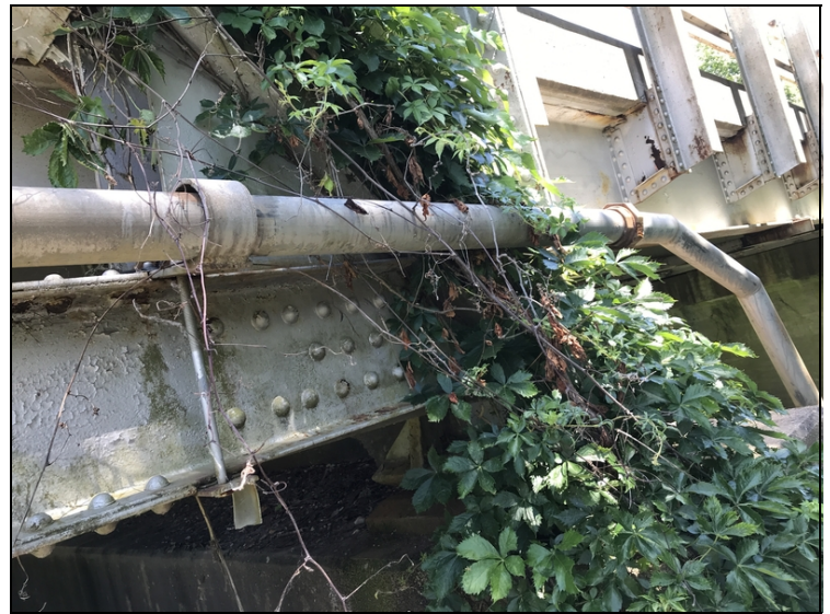
Bent #8 both sides have vines growing up bent onto truss and roadway.
