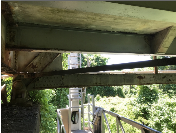
Span #7 stringer #5 at bent #7 is lifted up one inch breaking concrete stiffener.
