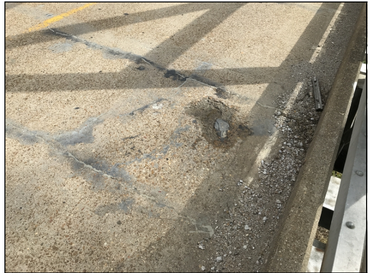
Span #3 right lane 1/4 span has one foot spall no rebar exposed.
