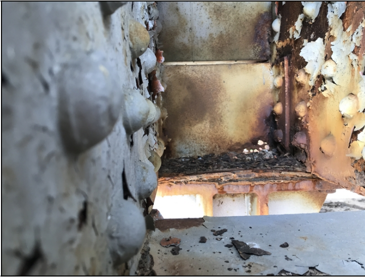
Span #5 at bent #5 right side lower cord inside at end above bearing has a transverse connection plate with section loss and holes.
