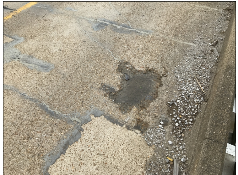
Span #3 right lane 3/4 span has two foot spall no rebar exposed.
