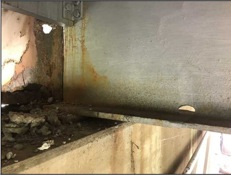
Span #8 bent #9 girder #4 has a t-splice that is two feet long by ten inches tall.
