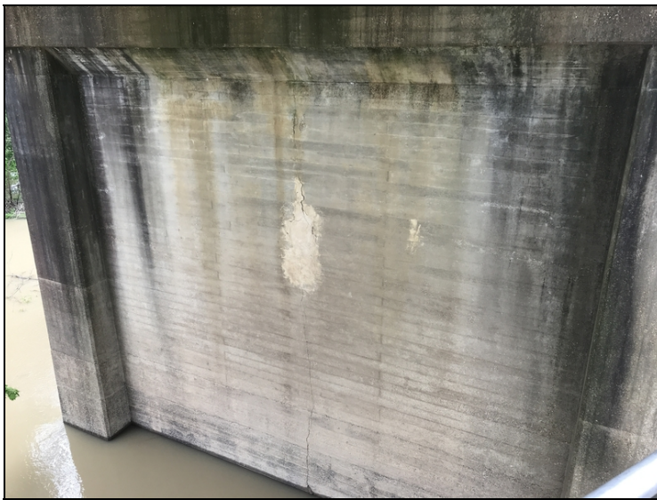
Bent #4 ahead face cs3 crack in center of pier wall.
