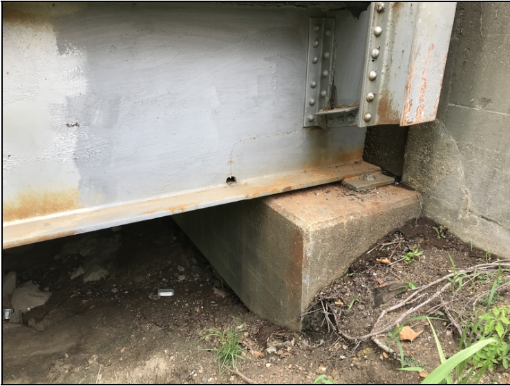
Span #9 girder #6 abutment #2 has been t-spliced two foot long eight inches tall.
