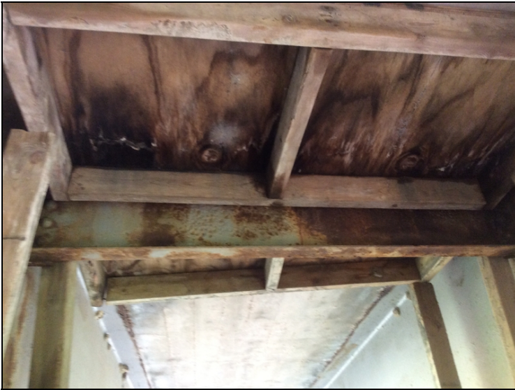
Bent #2 span #1,2 between girders #3,4 has forms left in place.
