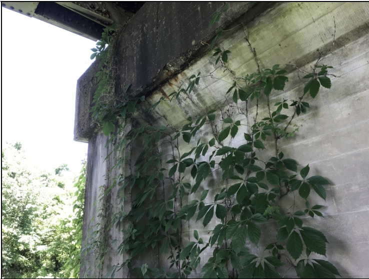
Bent #8 cap back face by column #1 has three foot long spall with exposed rebar to bottom where cap meets pier wall.
