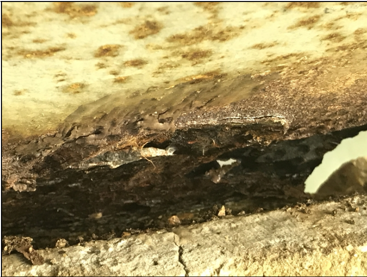
Span #2 girder #3 at bent #2 bottom flange has 3/4" hole rusted through ahead of bearing.
