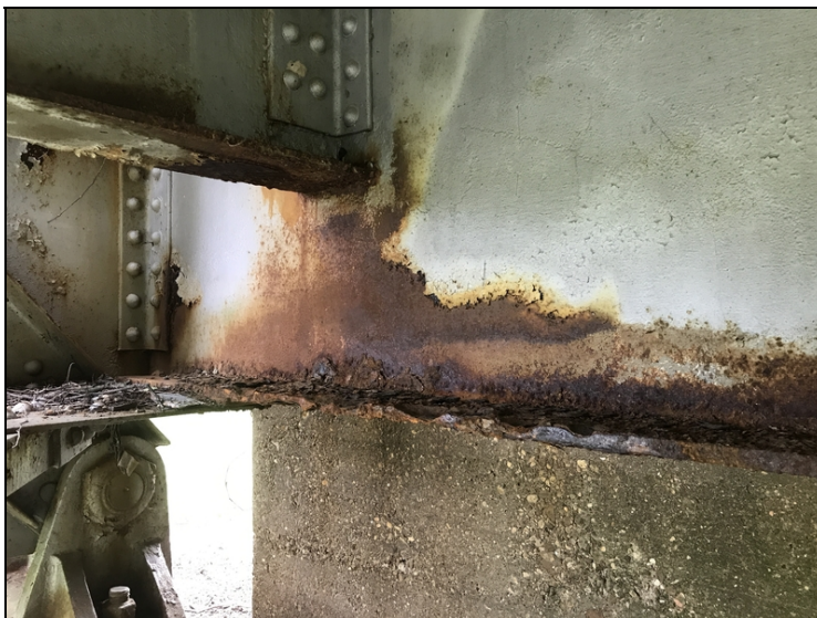
Span #7 floor beam #9 left end for three feet lower flange into web has corrosion with laminations and section loss up to 90%.
