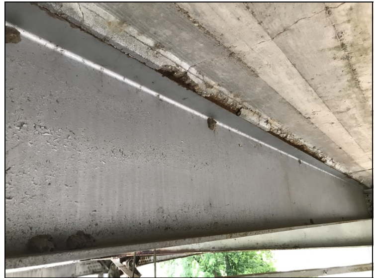
Typical areas beside stringers spalling due to pack rust on stringers top flange.
