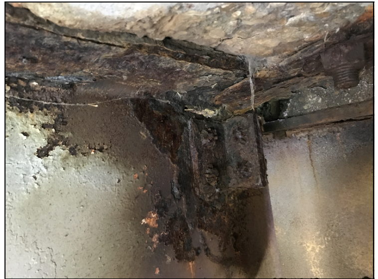
Span #8 girder #3 at bent #8 has a three inch hole in web above diaphragm.
