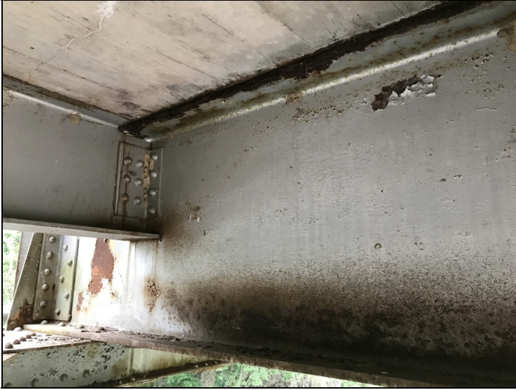
Typical ends of floor beams on all truss spans except those at bents.
