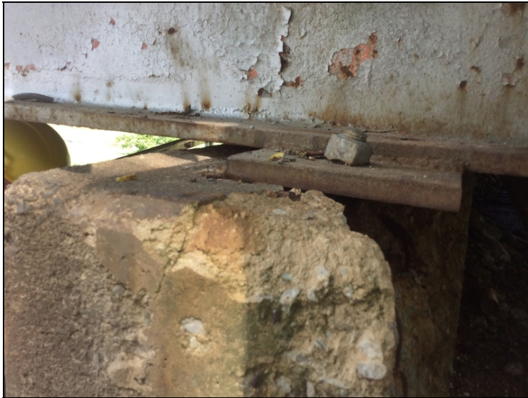
Bent #3 span # 2 cap spalled reduced bearing area to 50%.
