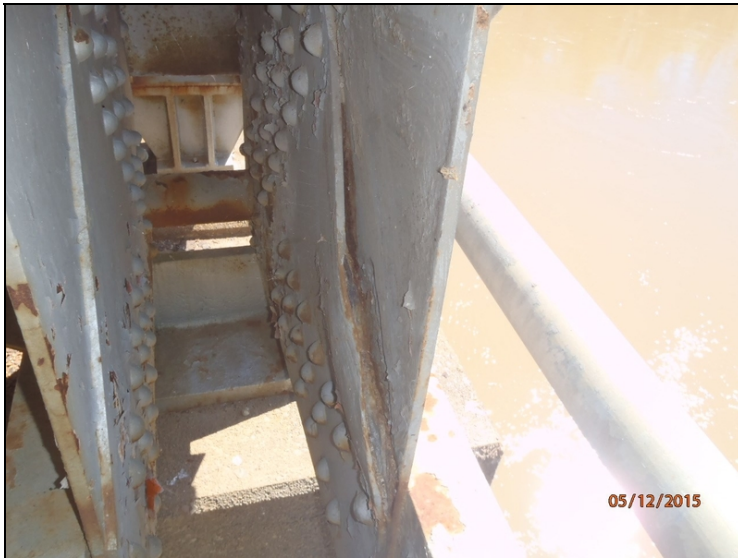
Gusset plate span #4 right side L0 connection.
