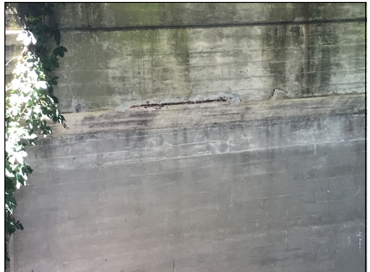
Bent #8 cap ahead face close to column #2 has a three foot piece of rebar exposed where cap meets pier wall with 10% section loss.
