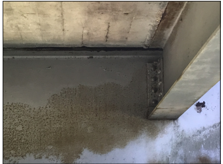
Typical corrosion on top flange of floor beam ends everywhere but ends of truss.
