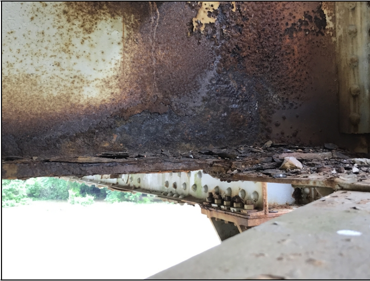
Span #4 at bent #5 floor beam #9 right side at connection to lower chord last 2' has up to 90% section loss on lower flange and 20% section loss in web.
