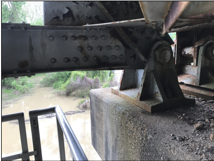
Typical fixed bearing truss.
