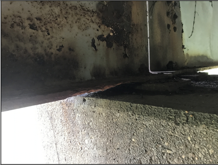
Span #8 bent #9 girder #1,5 first two feet of bottom flange has corrosion up to a knife edge.
