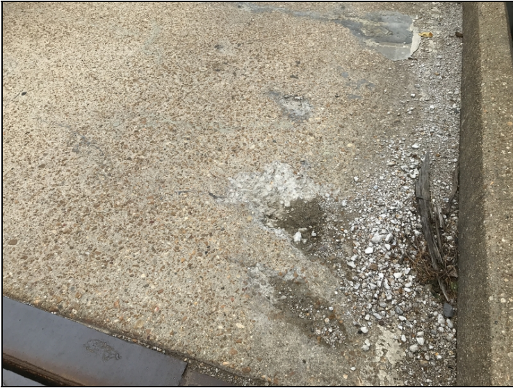
Span #4 right lane at bent #4 has one foot spall no rebar.
