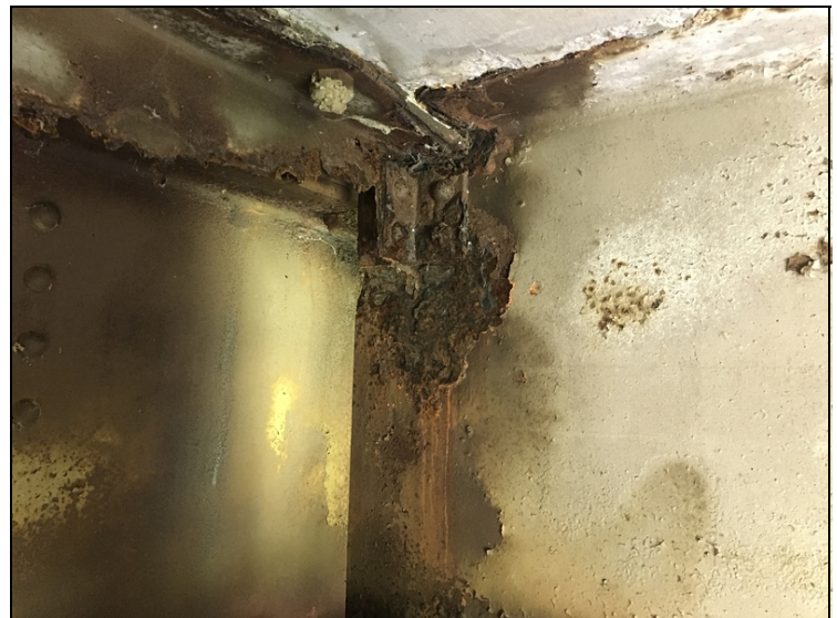
Span #8 bent #8 girder #2 web first foot at top at diaphragm connection has corrosion with laminations and section loss up to 50%.
