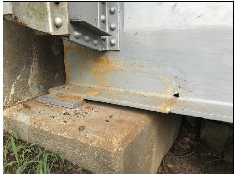
Span #1 girder #6 bent #1 has a t-splice first two feet six inches tall.
