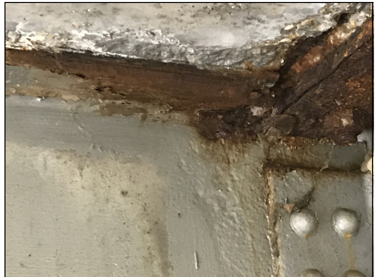
Span #7 stringer #1 at bent #8 web at top flange has a two inch hole on end.
