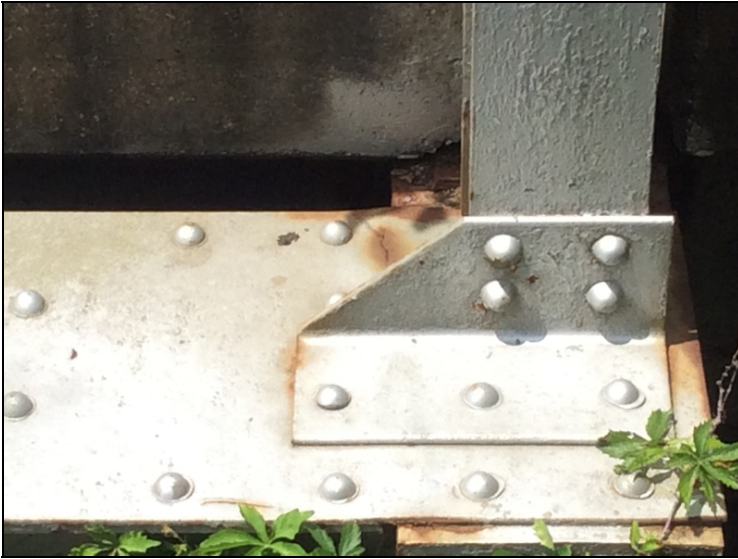
Span #7 lower chord cover plate at end of truss on right side L8 connection has two inch crack at floor beam connection.
