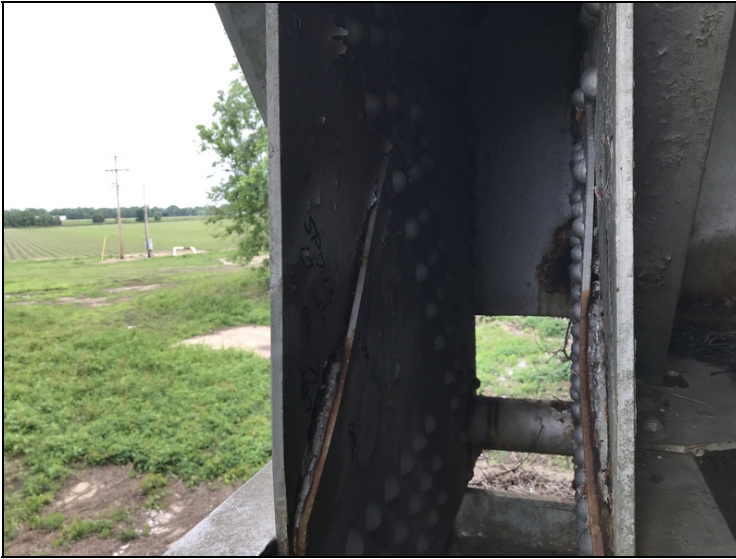
Gusset plate span #7 bent #8 left side L8 connection.
