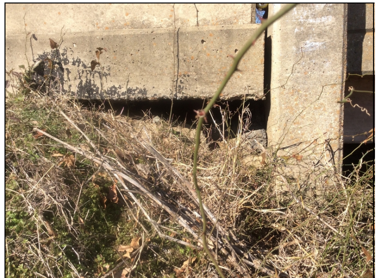
Large void under approach slab abutment #1 right side.
