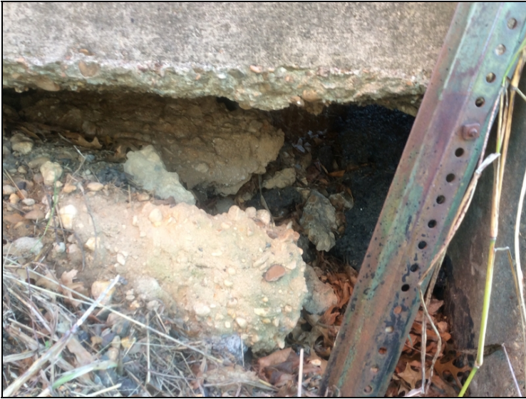
Large void under approach slab abutment #2 left side
