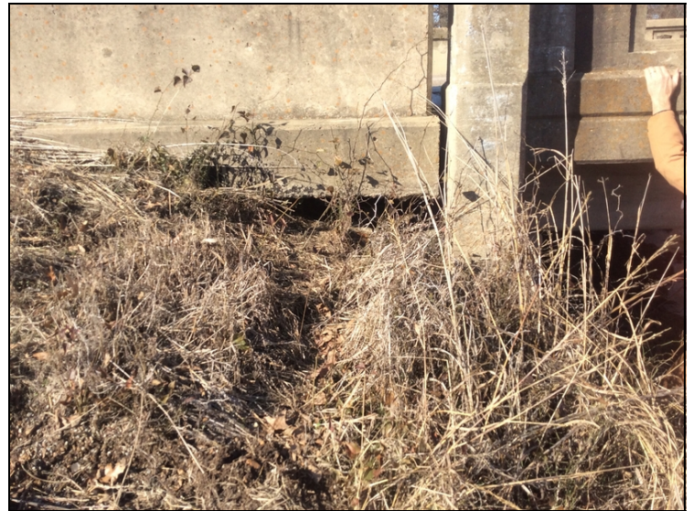
Ab #1. Right approach gutter undermined
