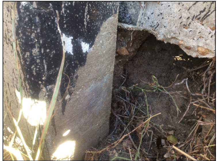
Monument post abutment #2 right side undermined
