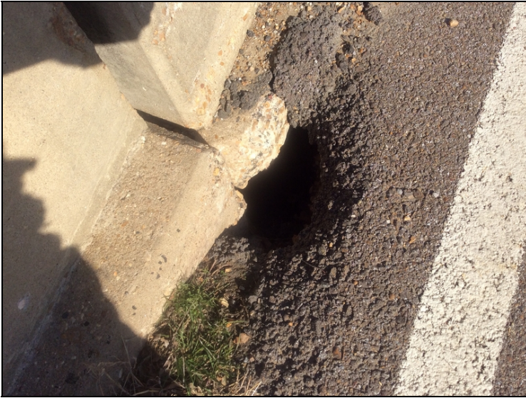
Void under approach slab abutment #2 left side.
