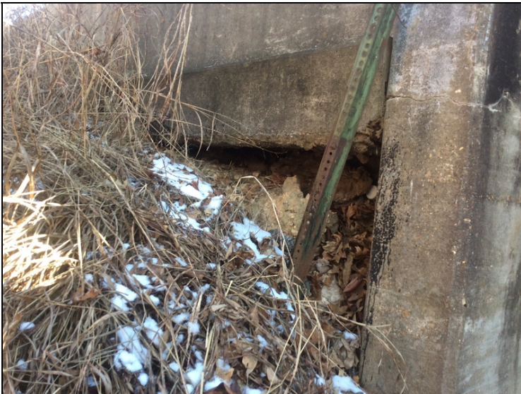
Erosion under abutment #2 left approach gutter
