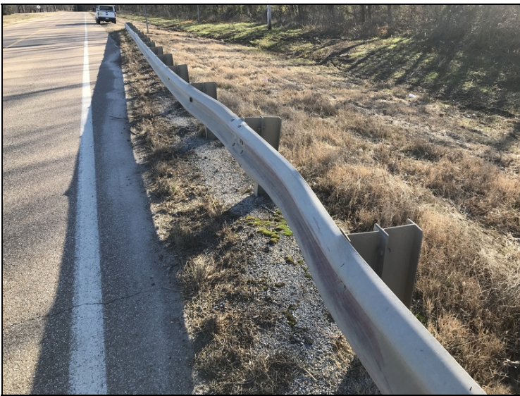
Abutment #2 right approach rail has collision damage twenty feet from bridge end.
