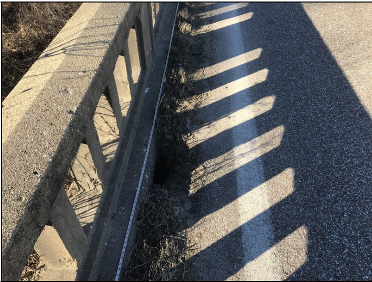
Gutters are full of dirt and debris with vegetation growing in them.
