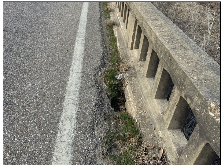
Dirt, debris and vegetation in gutters.
