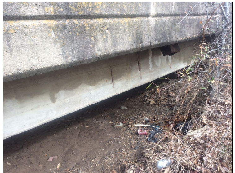
Typical sides of girders with exposed secondary rebar
