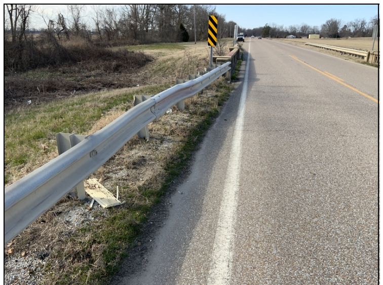
Abutment #2 right approach rail damage.
