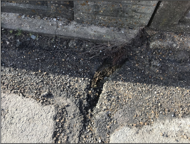
Hole in right gutter at bent 10.
