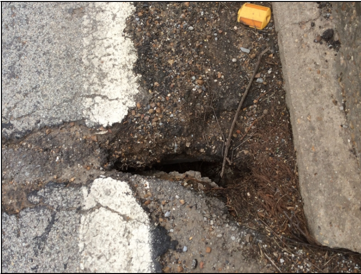
Bent#10 right shoulder hole in deck
