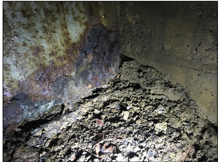
Girder #2 last 10" has 1" tall area of 100% section loss in web near bottom flange at girder end. Bottom flange has up to 80% section loss last 3'.
