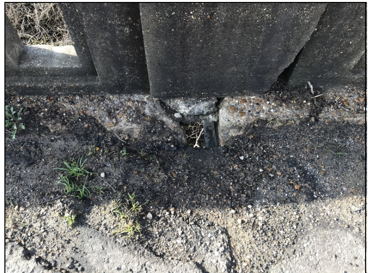
Hole in right gutter of bent 9.
