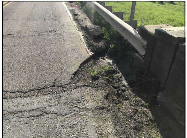
Abutment 2 right shoulder overlay spalled 3' x 4' x 4" deep.
