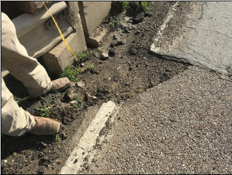
Abutment 1 left shoulder overlay spalled.
