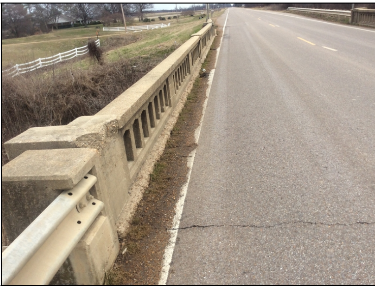
Gutters full of dirt and vegetation
