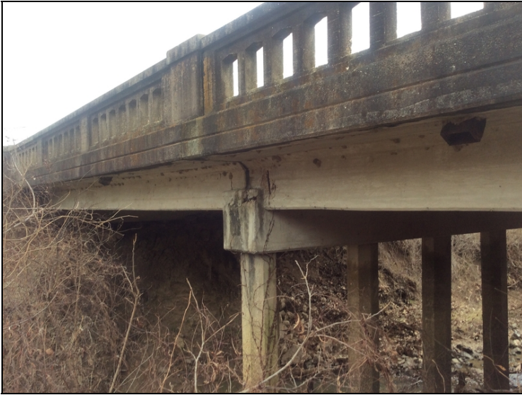
Left end cap at bent #2 and side of concrete t beam span #1 bent #2
