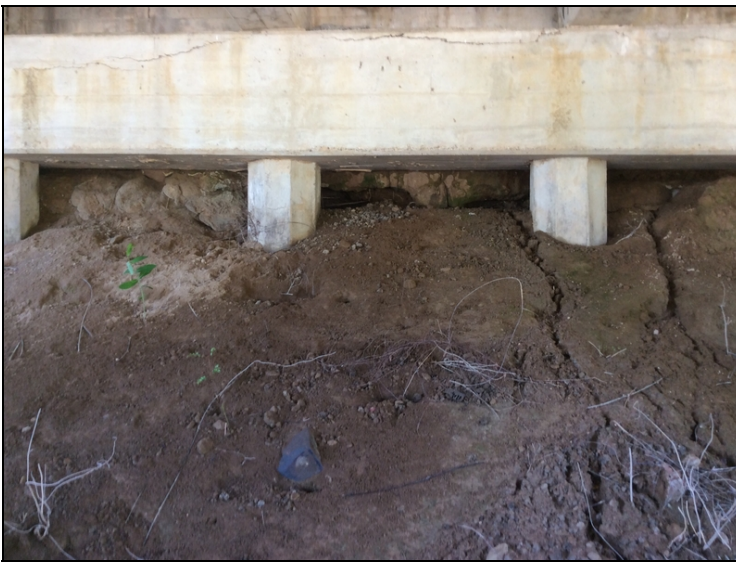
Abutment #2 is undermined 2'.
