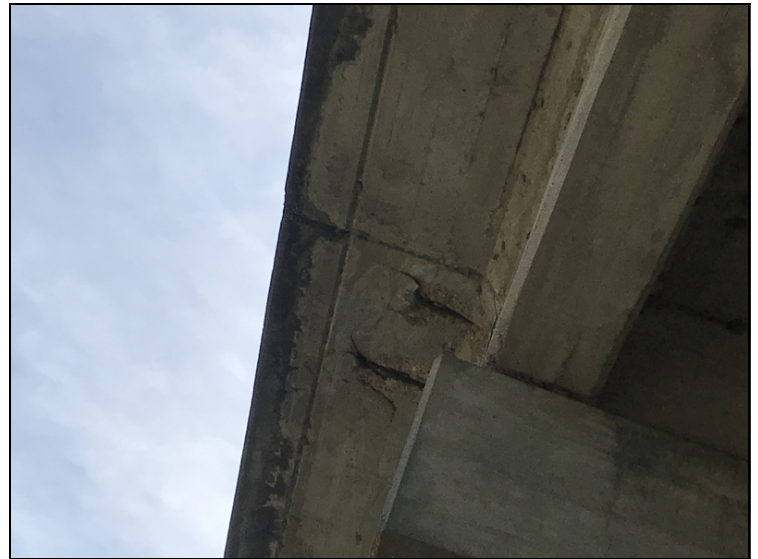
Typical spalls on soffit-under surface overhang.
