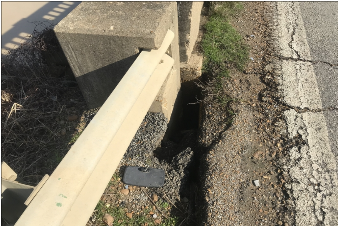
Hole in abutment 1 left approach shoulder.
