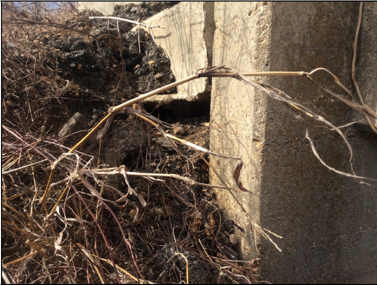
Abutment #1 right approach gutter undermined with hole in roadway
