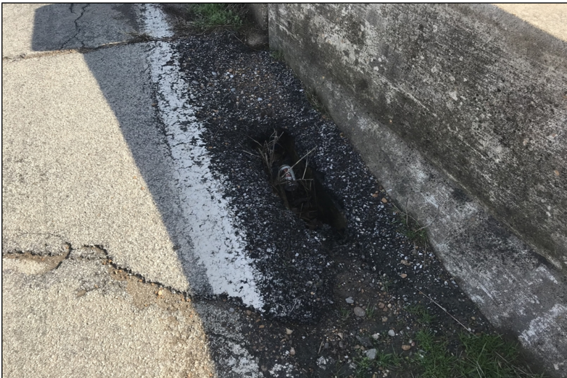
Hole in abutment 1 right approach shoulder.
