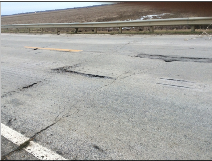
Abutment #2 right approach rail minor damage
