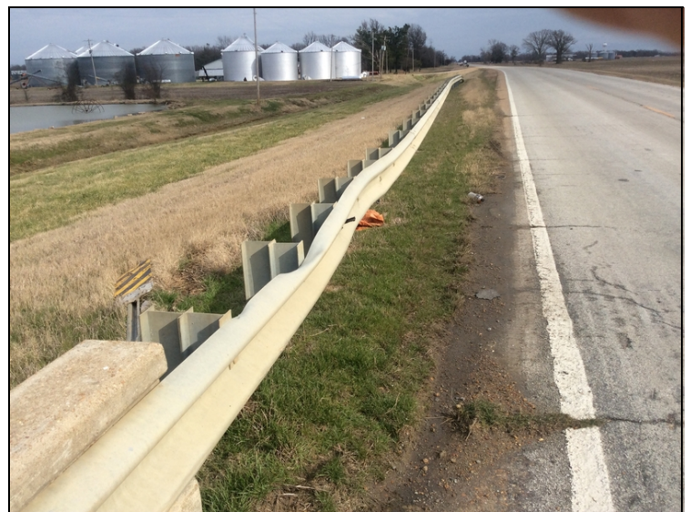
Abutment #2 left approach rail minor damage
