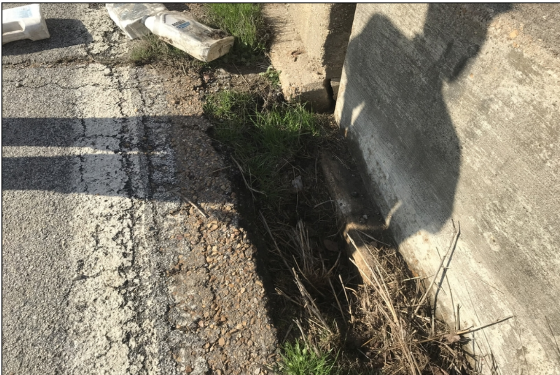
Hole in abutment 2 approach gutter left side.
