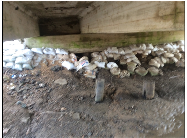
Abutment #2 bags falling down
