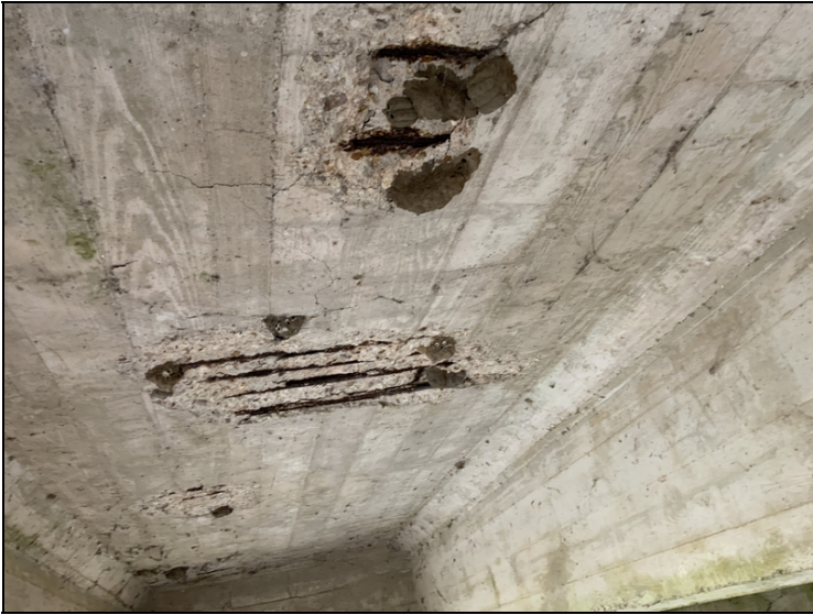
Bay #1 soffit spalls.
