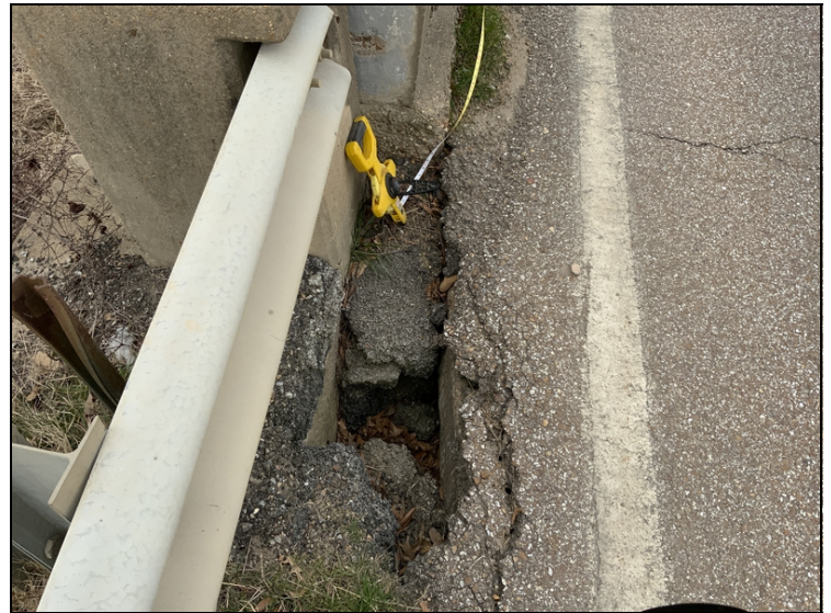
Abutment #2 right side hole in approach shoulder and void underneath slab.
