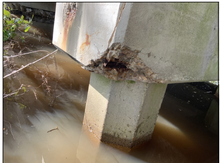
Bent #2 cap ahead face bottom right end has a one foot spall with exposed rebar with 5% section loss.
