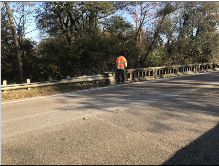
Abutment #1 left side monument post has been broken off and approach rail has collision damage.
