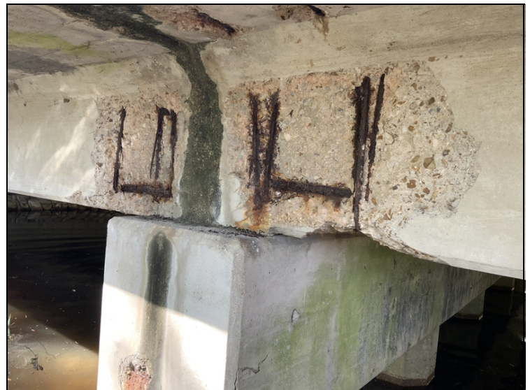
Spans #1 and 2 girder #5 spalled with exposed rebar at bent #2.
