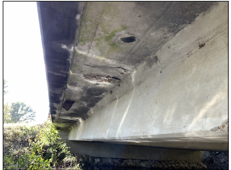
Typical soffit overhang spall with exposed rebar.
