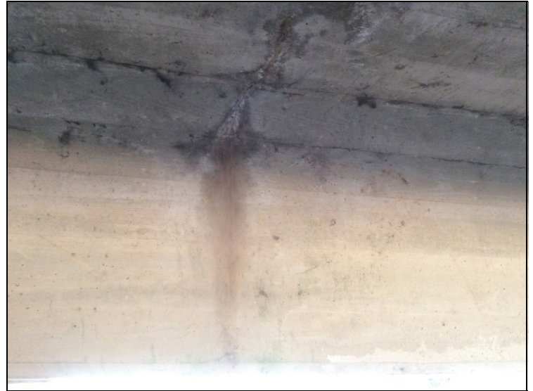
Soffit crack with efflorescence extending into girder.
