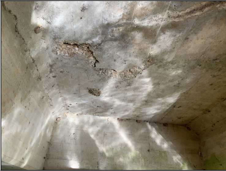
Soffit span #1 bay #4 at bent #2 has 1' delamination and 6' of exposed rebar.
