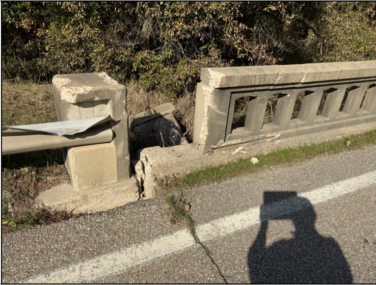
Abutment #1 left monument post broken off.
