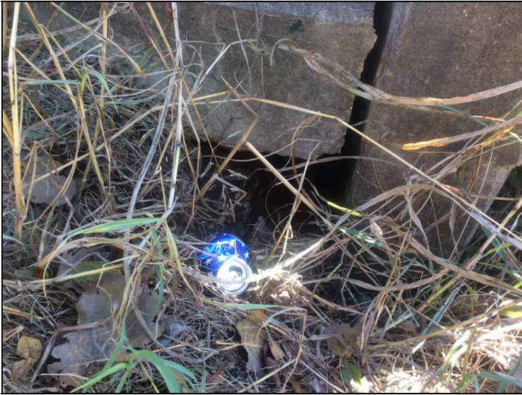
Erosion under abutment #2 left approach gutter.
