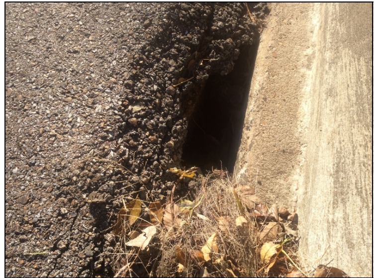
Hole at abutment #2 left approach shoulder.
