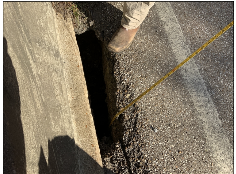
3' long by 2 1/2' deep hole in abutment #2 left approach gutter.
