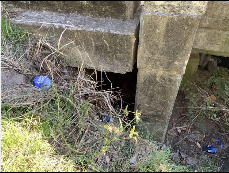
Void under abutment #2 approach slab left side.
