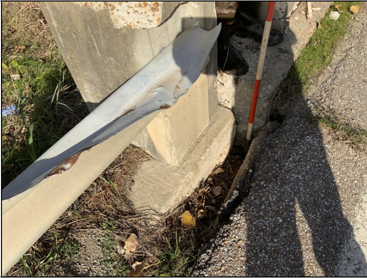
Hole in abutment #1 left approach gutter.
