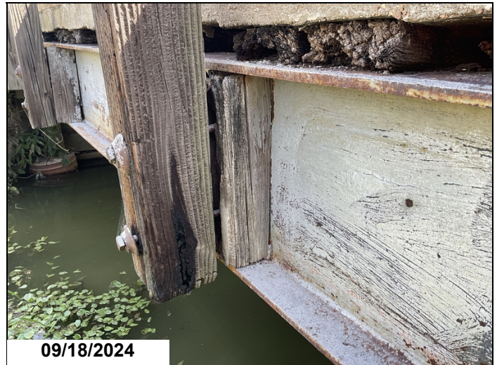
Typical, decayed rail post spacers, left side.
