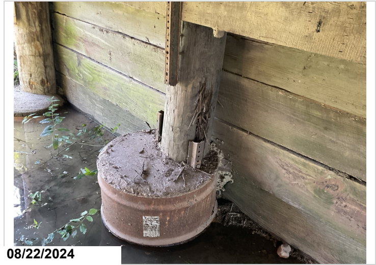
Abutment 1, pile 4: minor outer shell decay on upper section of spliced pile. 1EA CS3
