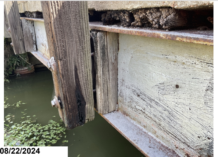
Typical, decayed rail post spacers, left side.
