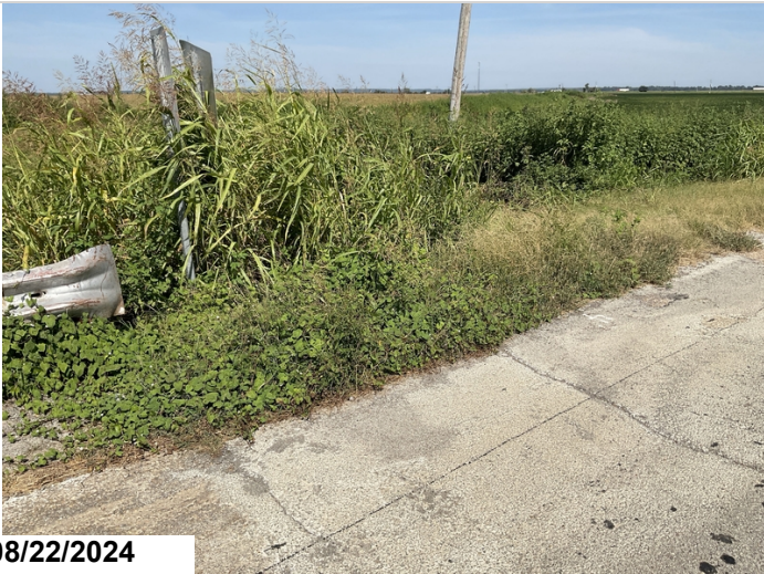
Abutment 2, approach rail, left side: missing.
