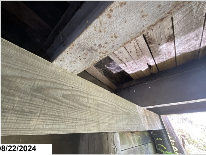
Typical missing timber sub deck at abutment 2
