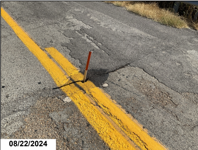
Small hole in abutment 2, approach roadway with 2' deep void underneath.
