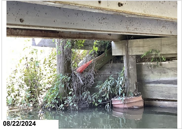
Abutment 2, timber back wall, left side: decayed with missing and broken boards , timber pile is leaning in.
