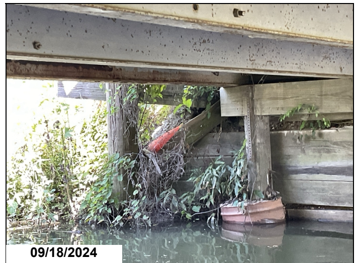
Abutment 2, timber back wall, left, side: decayed with missing and broken boards , timber pile is leaning in
