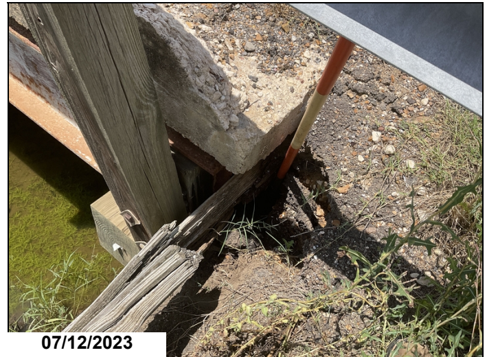
Abutment #2 right approach shoulder has two foot deep void
