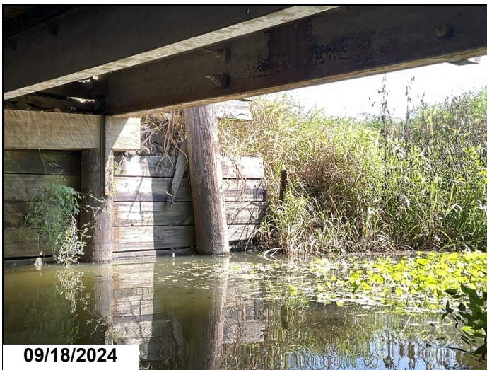
Abutment 2, timber back wall, right side: decayed with missing and broken boards
