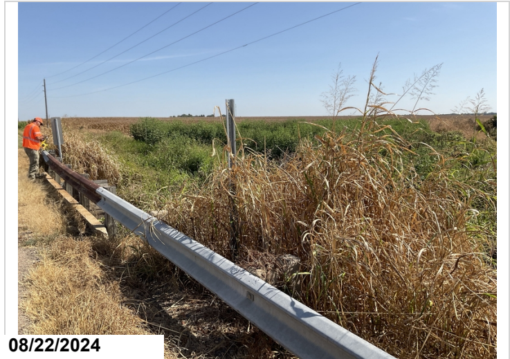
Abutment 1, right flair board and log mile sign missing
