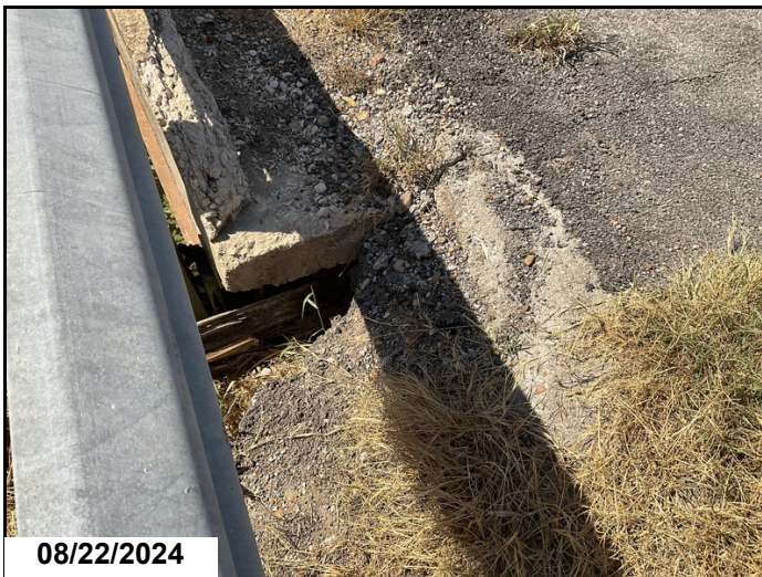
Abutment 2, right shoulder: eroded at bridge end.
