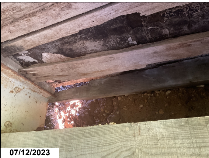
Void behind girder #4 at abutment #2
