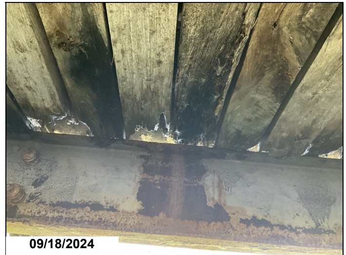
Typical missing timber slab deck over exterior girders
