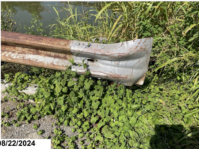
Bridge rail, left side: not connected to last rail post. Connection 1LF CS3
