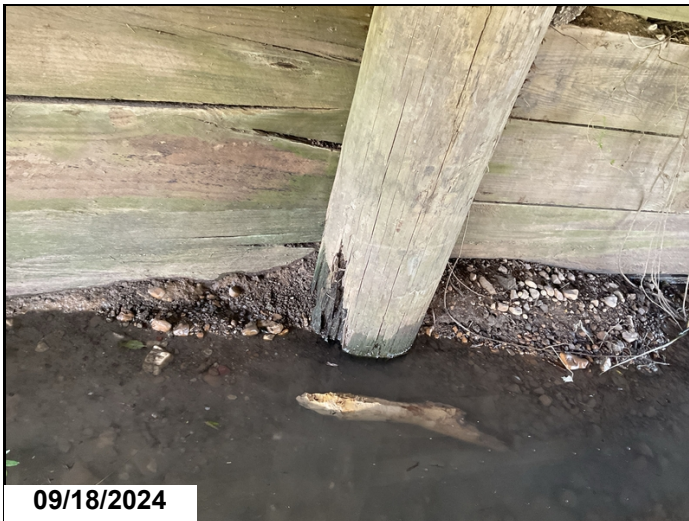
Abutment 1, pile 3: moderate decay at ground line. 1EA CS3
