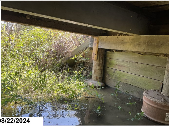
Abutment 1, timber back wall, right side decayed with broken and missing boards.
