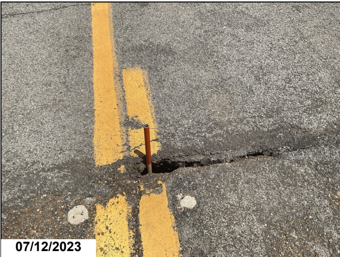
3' deep hole in abutment #2 approach roadway at centerline
