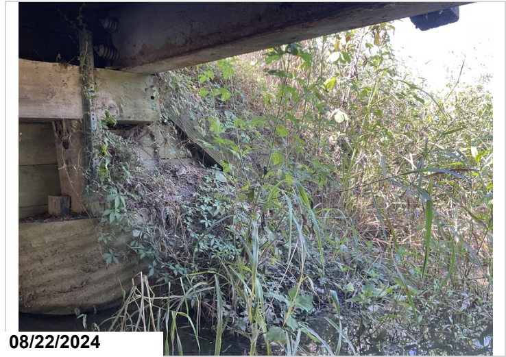
Abutment 1, timber back wall, left side decayed with broken and missing boards.
