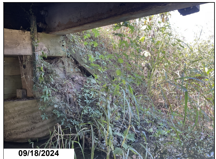
Abutment 1, timber back wall, left side decayed with broken and missing boards.
