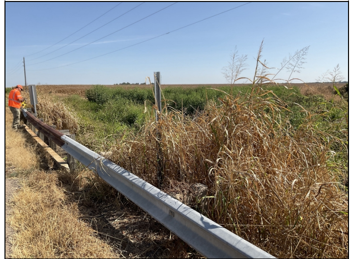
Abutment 1, right flair board and log mile sign missing
