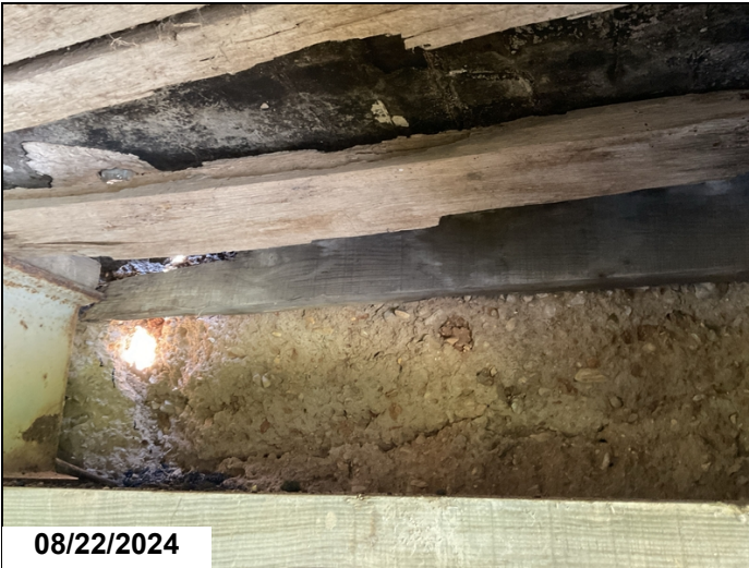
Abutment 2, void at centerline above cap where timber back wall is missing
