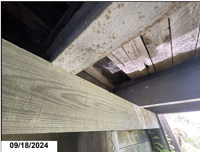
Typical missing timber sub deck at abutment 2
