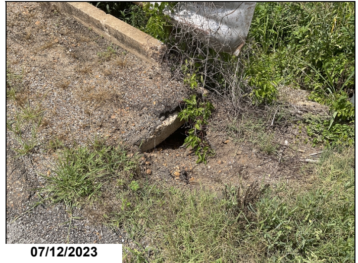
Abutment #2 left approach shoulder has two foot by two foot by one foot deep hole at bridge end
