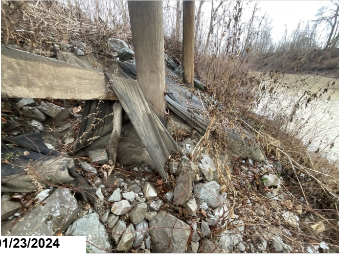
Displaced riprap and filter fabric east slope
