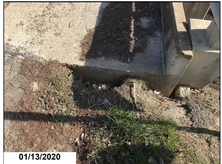
Abutment #1 right approach shoulder is eroded with two holes at bridge end.
