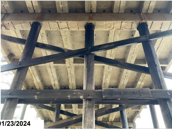
Span #7 soffit / underside of deck
