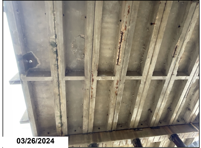
Span #3 soffit / underside of deck
