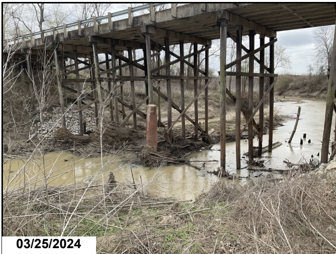
Silt and debris in channel
