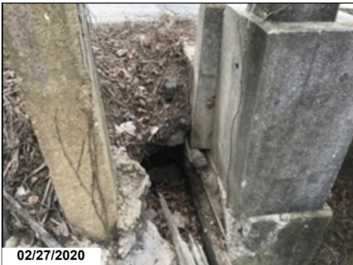
Abutment 2 left side, runoff has eroded shoulder at bridge end exposing bridge end and causing a 2' deep void under left shoulder.
