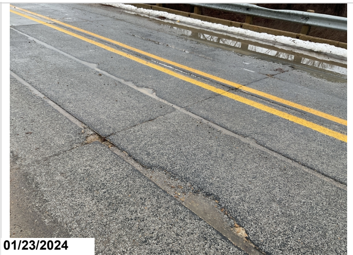
Typical deck spalling
