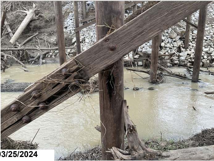
Bent #6 pile #4 has outer shell decay with moderate section loss.
