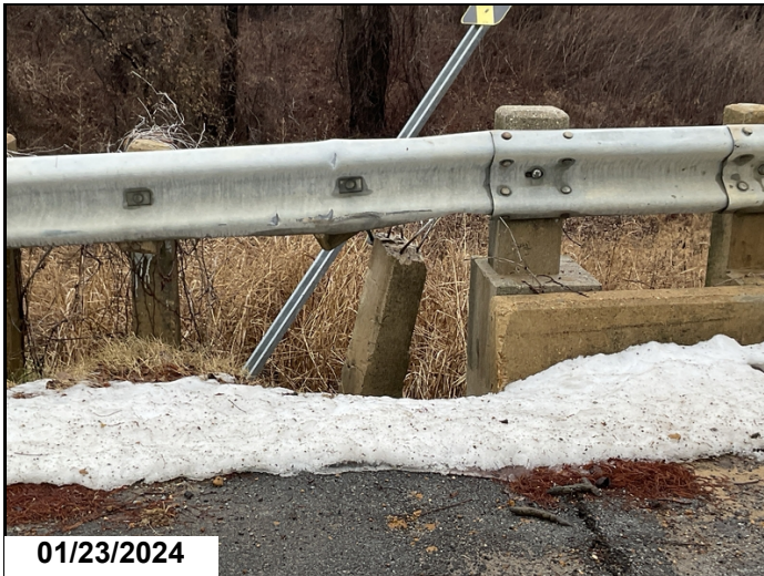
Abutment #1 left side last approach rail post spalled with exposed rebar
