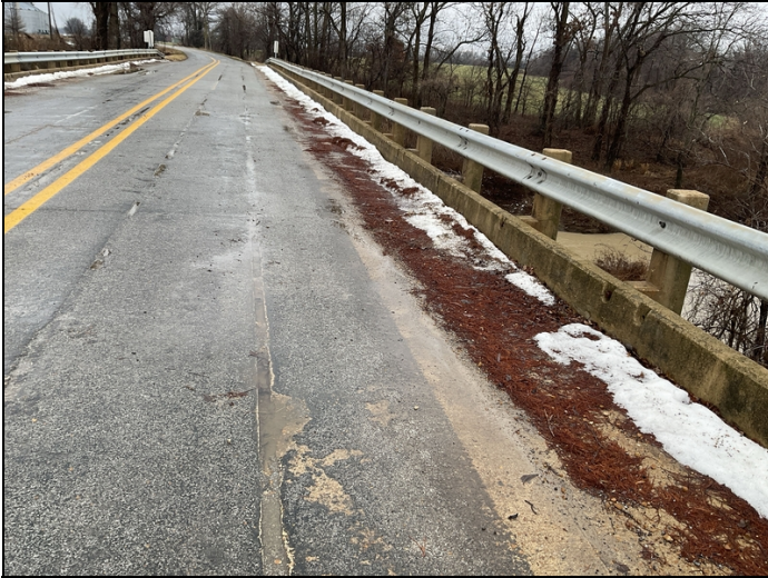
Dirt and debris in gutters
