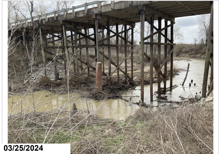
Silt and debris in channel
