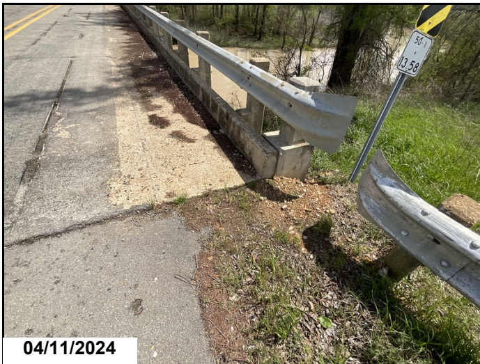
Erosion at abutment #1 right approach shoulder has been repaired at time of inspection.
