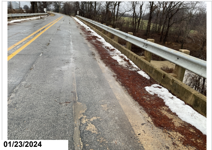
Dirt and debris in gutters
