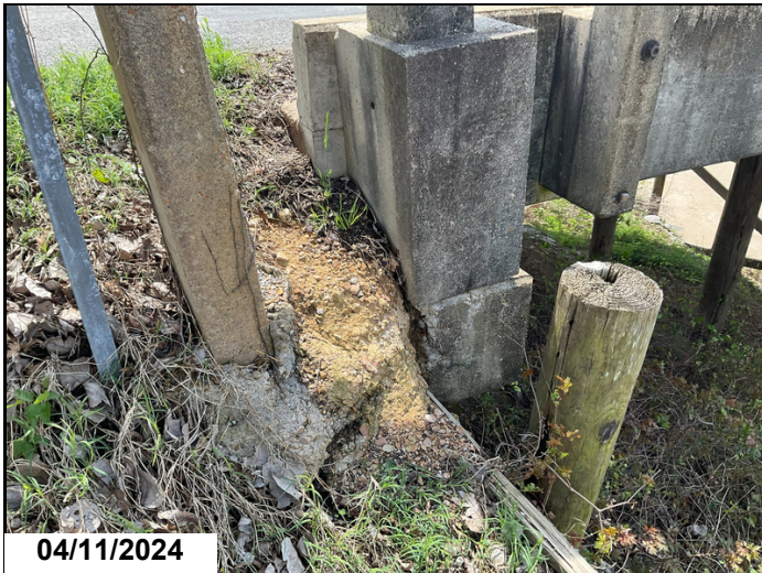
Void at abutment 2 left approach shoulder has been repaired at time of inspection.
