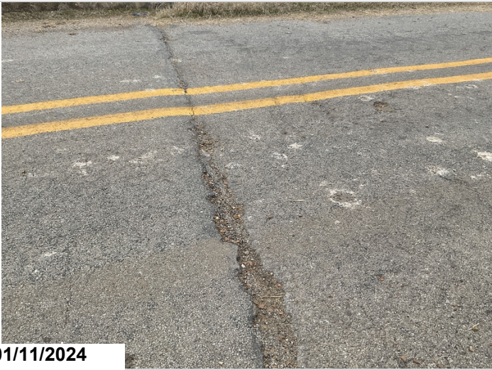
Abutment #2 approach roadway settlement
