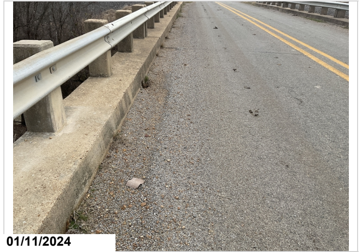
Dirt and debris in gutters
