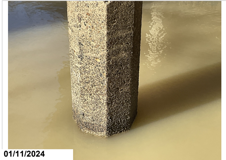
Typical abrasion on bent #3 piles
