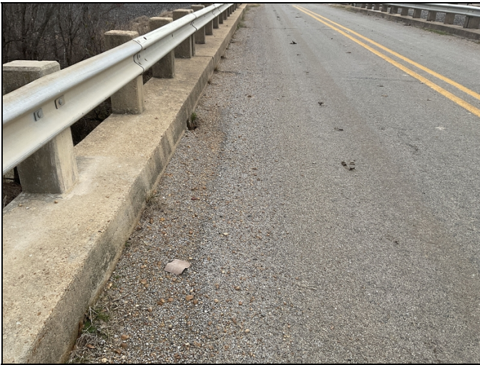
Dirt and debris in gutters
