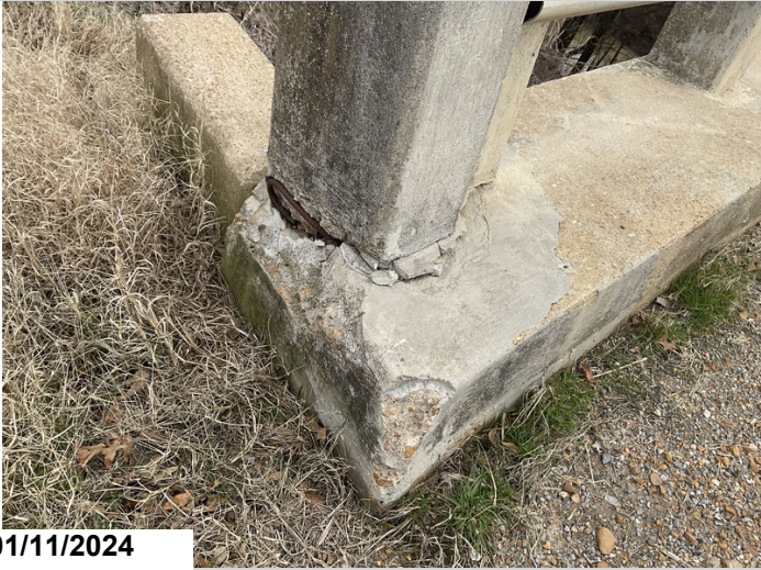
Abutment #2 right end post broken at bottom with exposed rebar and curb spalled
