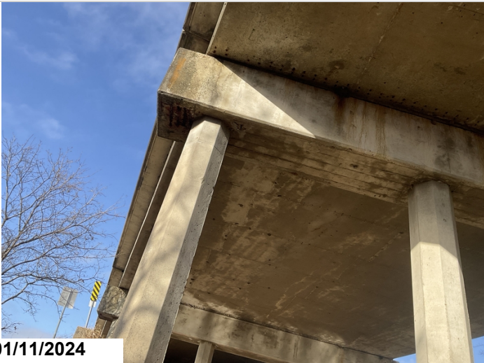
Typical exposed rebar on caps
