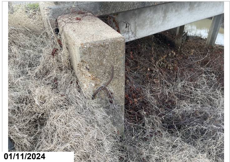
Abutment #1 right wing spalled with exposed rebar
