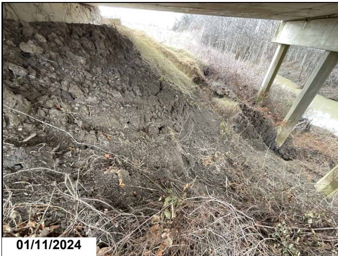
Abutment #1 slope erosion
