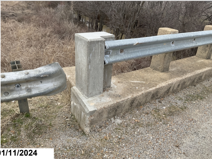
Abutment #1 left side first rail post has been replaced.
