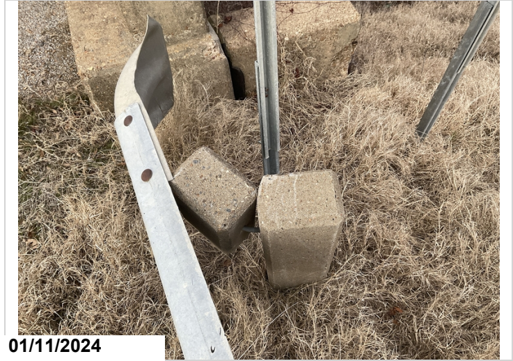
Last approach rail post misaligned and loose alignment abutment #1 right side
