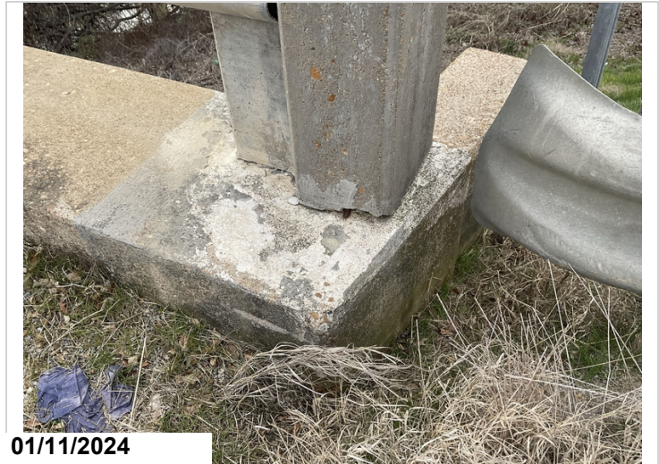
Attached #2 left end post broken loose at bottom with exposed
