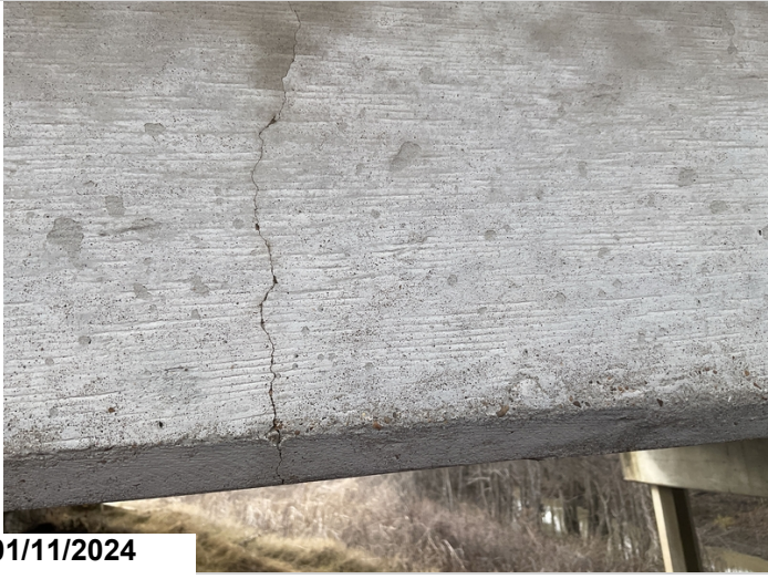
Typical vertical crack in side of slab
