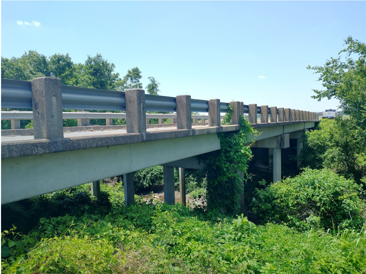
Site 3, Ditch 20 (June 2022) Looking north from the south
