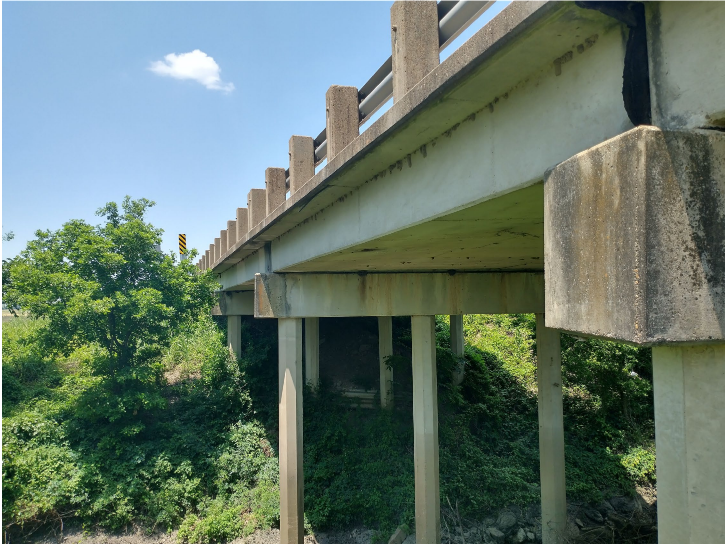
Site 3, Ditch 20 (June 2022) Looking south from the north
