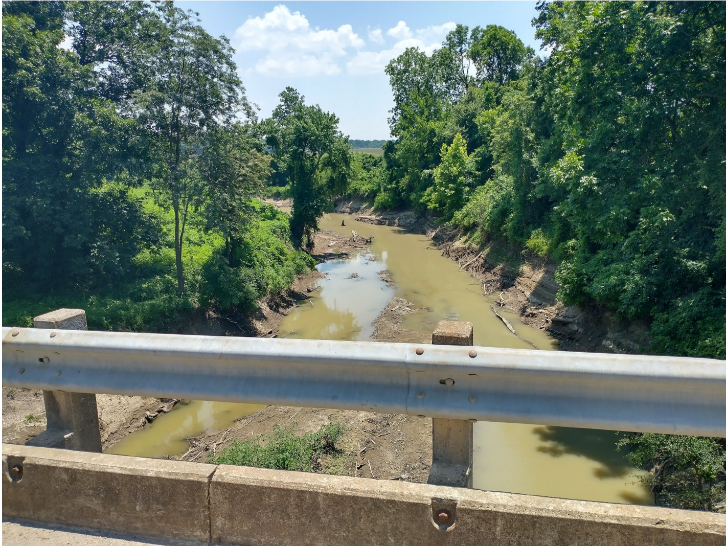
Site 2, Blackfish Bayou (March 2022) Looking down river to the south
