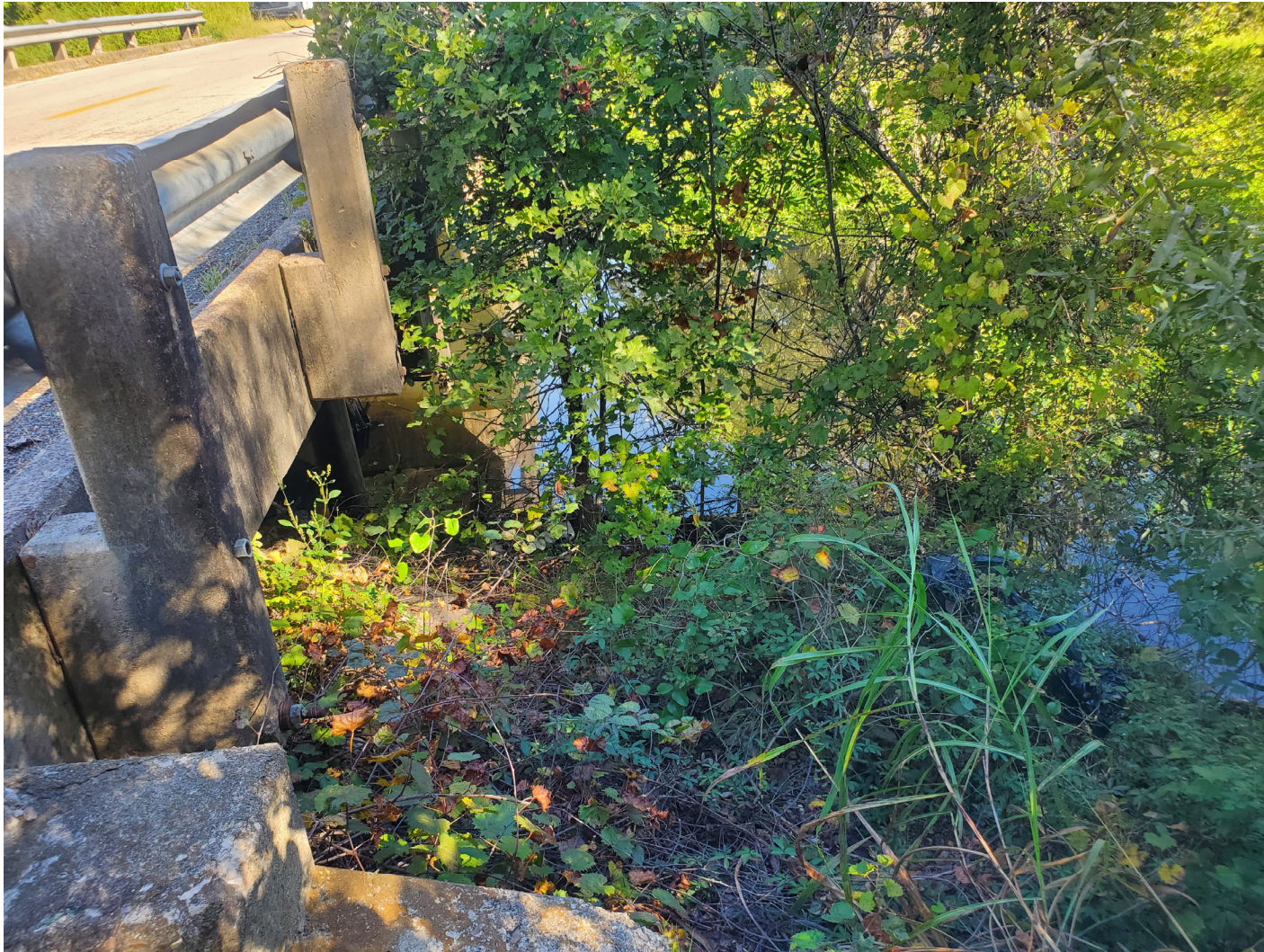
East Side of Bridge (September 2022) Looking North from the South
