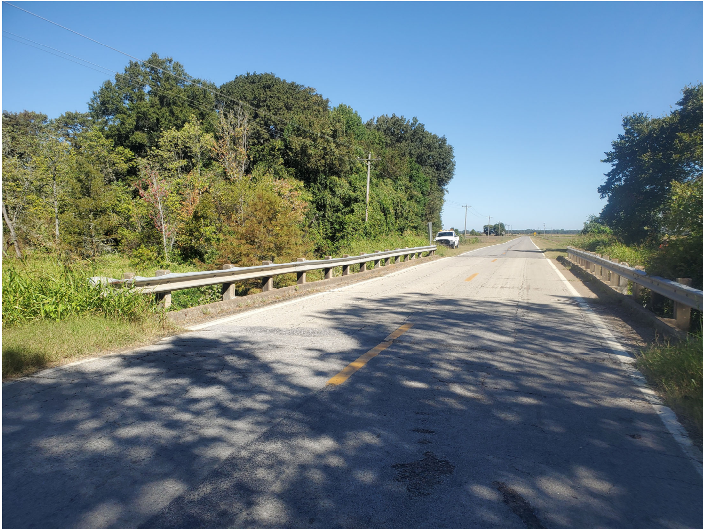
Bridge Deck (September 2022) Looking North from the South
