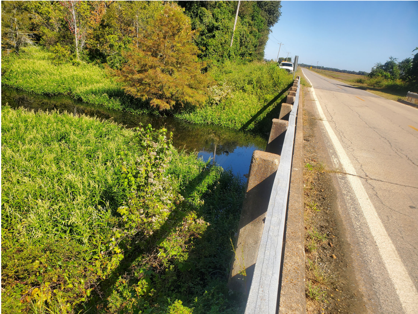
West Side of Bridge (September 2022) Looking North from the South
