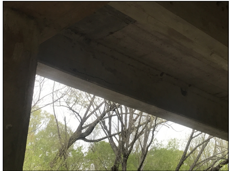
Span #12 girder #1 first ten feet from bent #12 has delamination.
