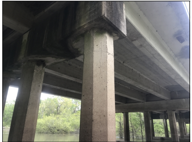
Bent #7 pile #5 has 3' of cracking near top.
