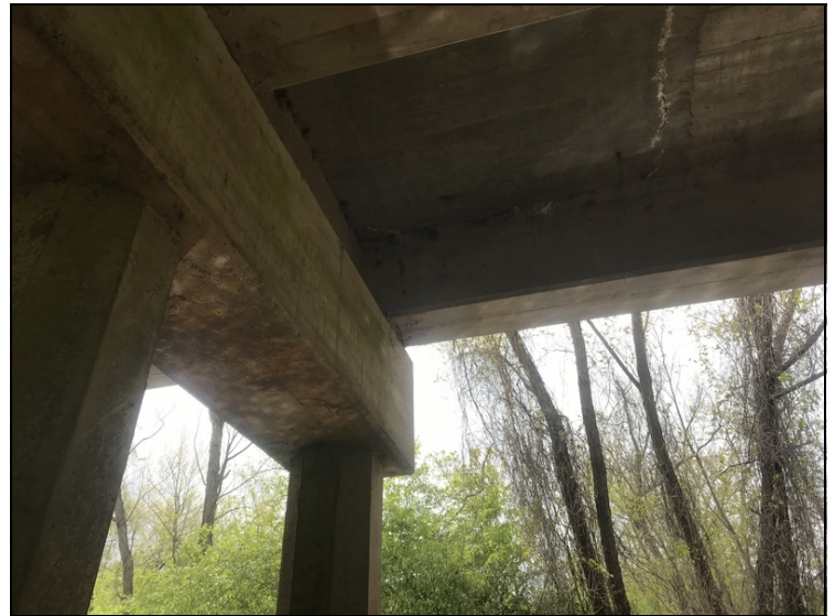
Span #13 girder #5 at bent #14 has 1' exposed rebar with 5% section loss.
