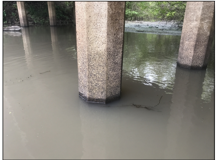
Typical abrasion on piles.
