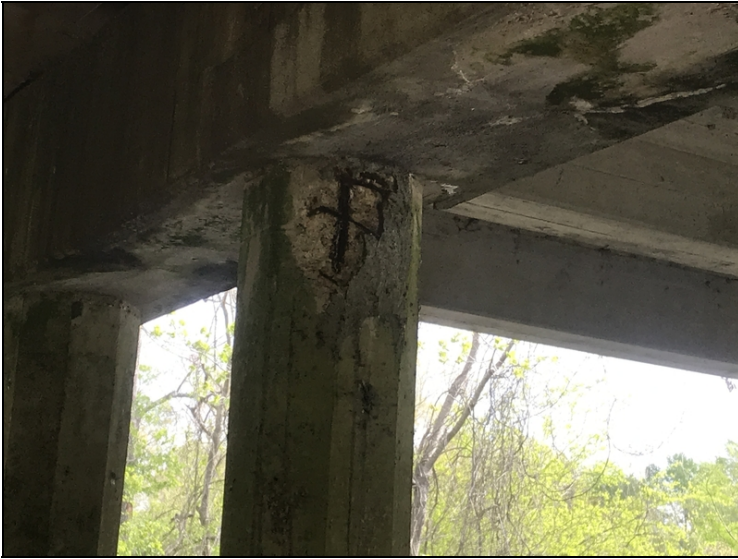
Bent #5 pile #3 1' spall at top with exposed rebar with 10% section loss.
