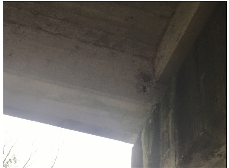
Span #5 girder #5 at bent #5 has a 1' spall on left side with exposed rebar no section loss.
