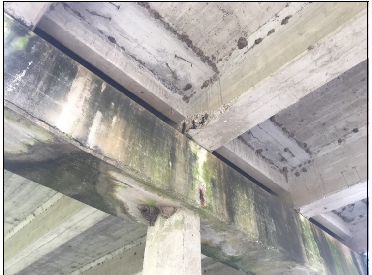
Span #7 girder #4 at bent #7 has a two foot spall with 1' exposed rebar with 20% section loss on right side.
