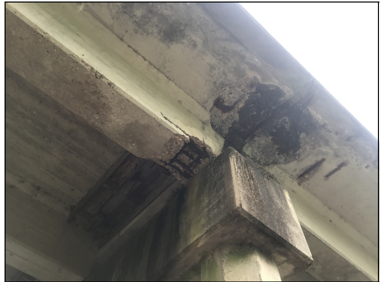
Span #6 girder #5 at bent #7 last one foot bottom of girder is spalled with exposed rebar with 20% section loss.
