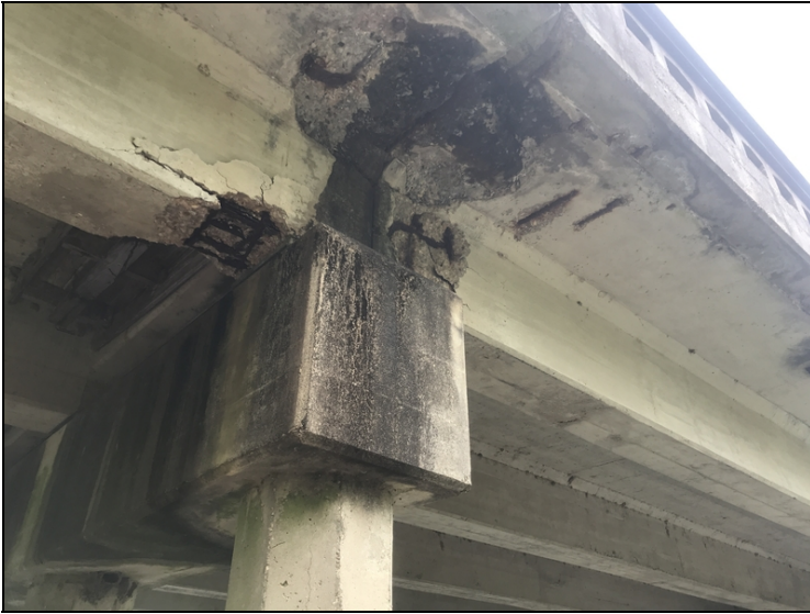
Span #7 girder #5 at bent #7 has a 2' spall on right side at bearing with rebar exposed with 20% section loss.
