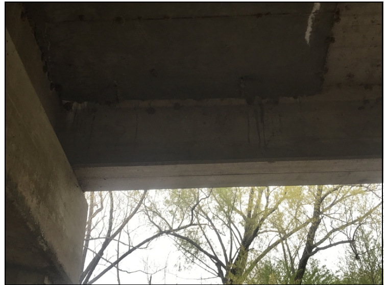
Span #14 girder #1 has a two foot delamination three feet ahead of bent# 14 on right side.
