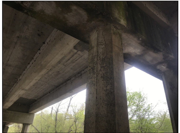
Bent #9 pile #4 cracked 3' near top.
