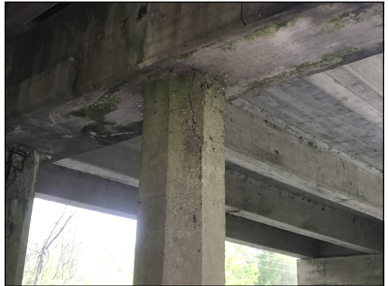
Bent #5 pile #4 1' delamination at top.
