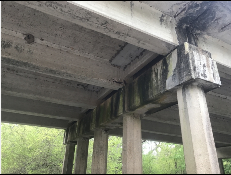
Span #7 bent #7 girder #2 has 3' of spalling with 1' exposed rebar with 20% section loss.
