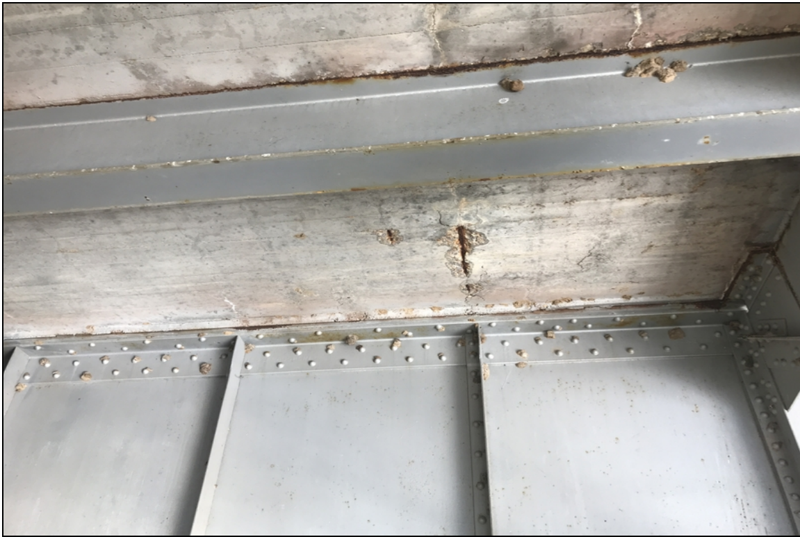
Exposed rebar on soffit span 3
