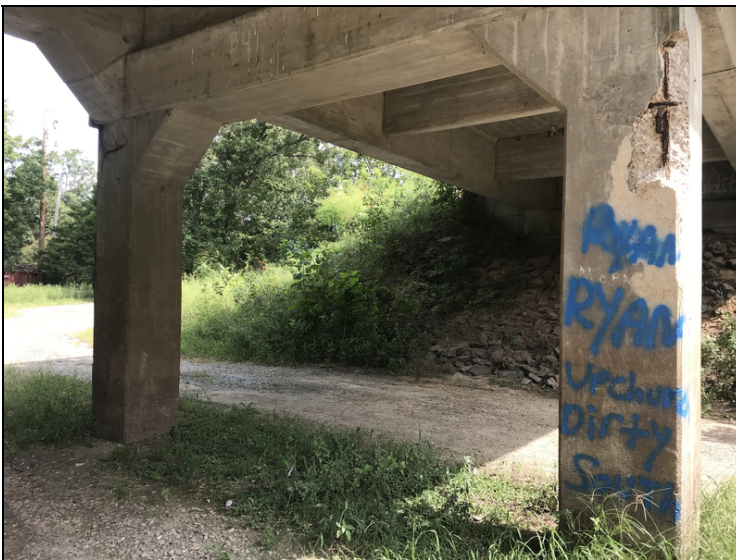
Bent 8 column 1 & 2 large spalls with exposed rebar
