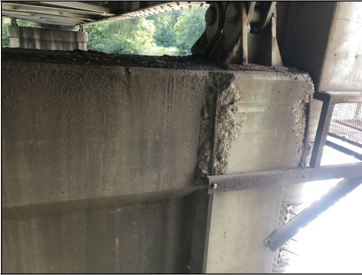
Back side pier 2, under girder 2: spalls with exposed rebar that has section loss. USGS river gauge is bolted to the cap and the bolts are loose.
