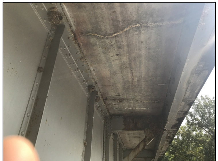
Span 5 right of girder 2: spalls with exposed rebar and transverse cracks with heavy efflorescence build up. Common deficiency at this span
