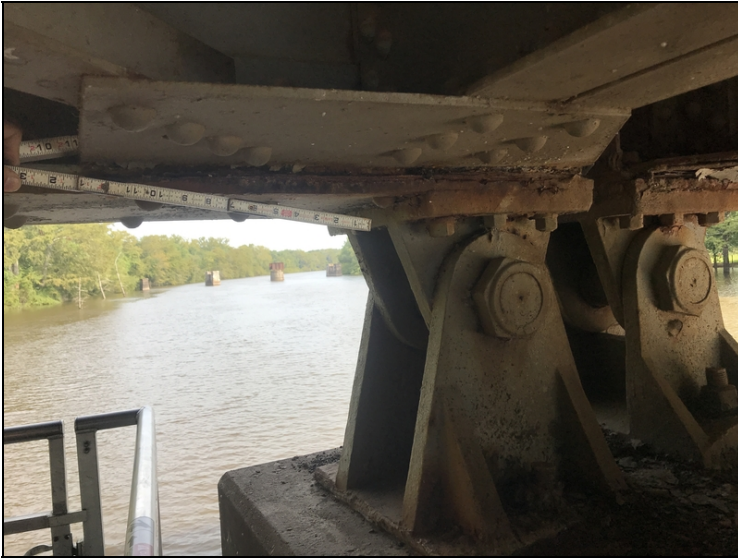
Pier 2 , Girder 1, span 3 Pack rust has developed between the diagonal brace gusset plate and the top of the bottom flange.
