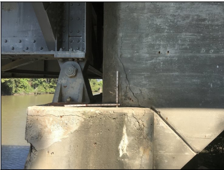
Right side pier 4: diagonal crack in the step up of the cap, also the main cap below.
