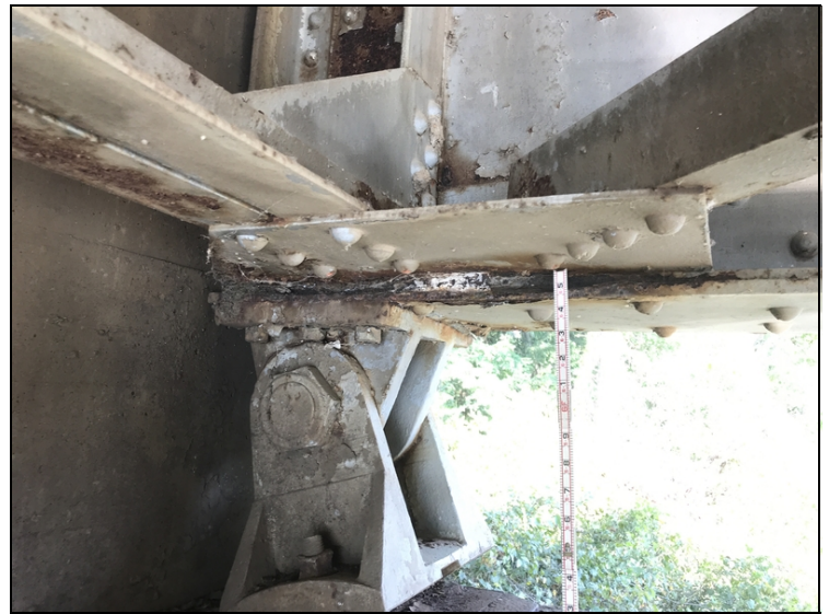
Pier 1, girder 1: pack rust between bottom flange and gusset plate above bearing. This is a common condition at all piers near the bearings
