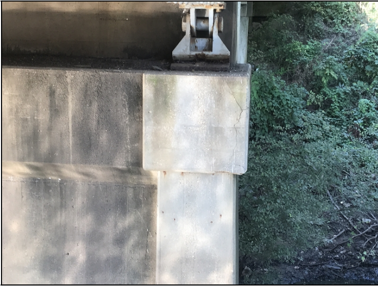
Ahead Pier 1, under girder 1: vertical crack under bearing
