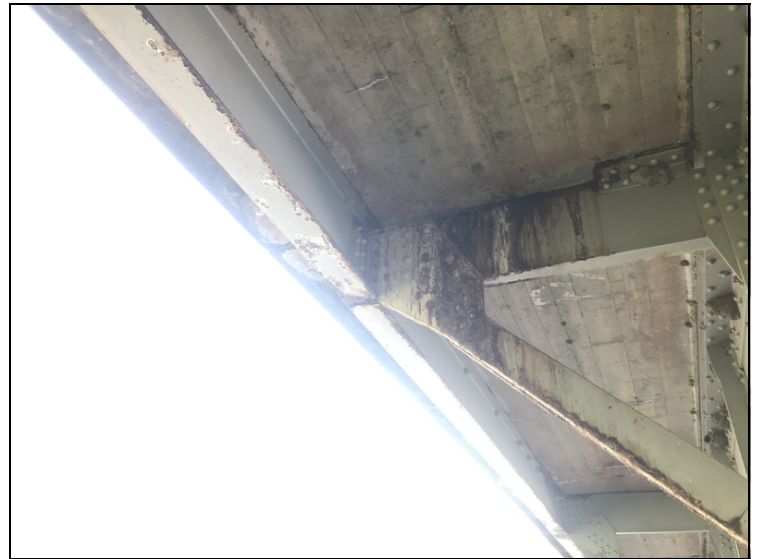
Span 3 left of girder 1 active rust on the cantilevered floor beams.
