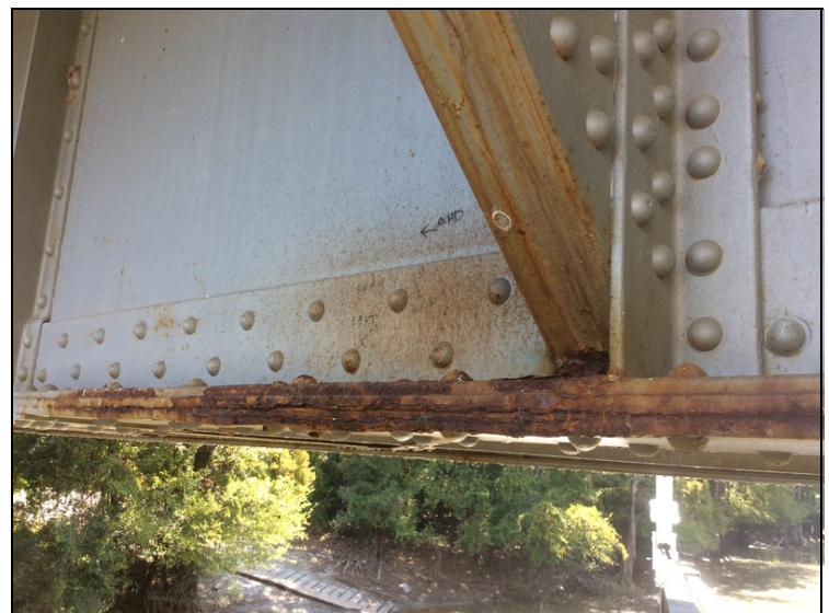
Span 5, girders 1 pack rust has deformed bottom flange at riveted built up section.
