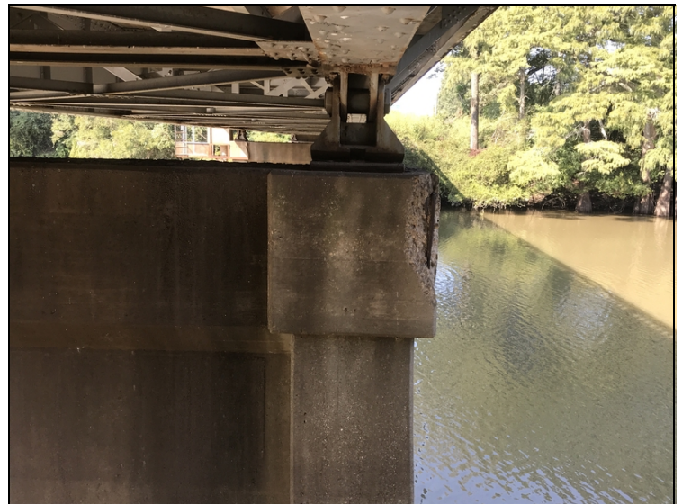
Ahead side of pier 3, left side: large spall with exposed rebar
