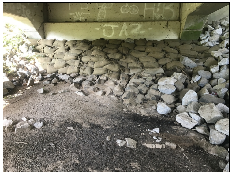
State forces have placed erosion countermeasures
