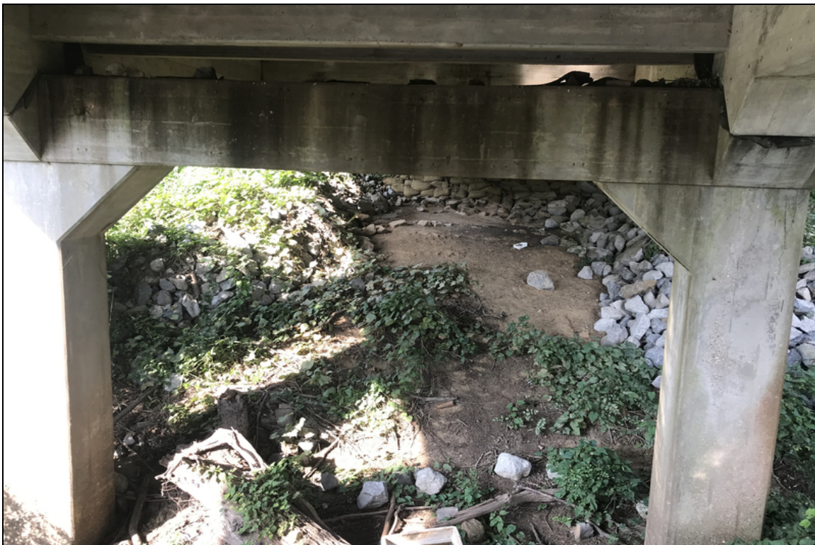
Bent 2 spall with exposed rebar on cap, cracks in both columns.
