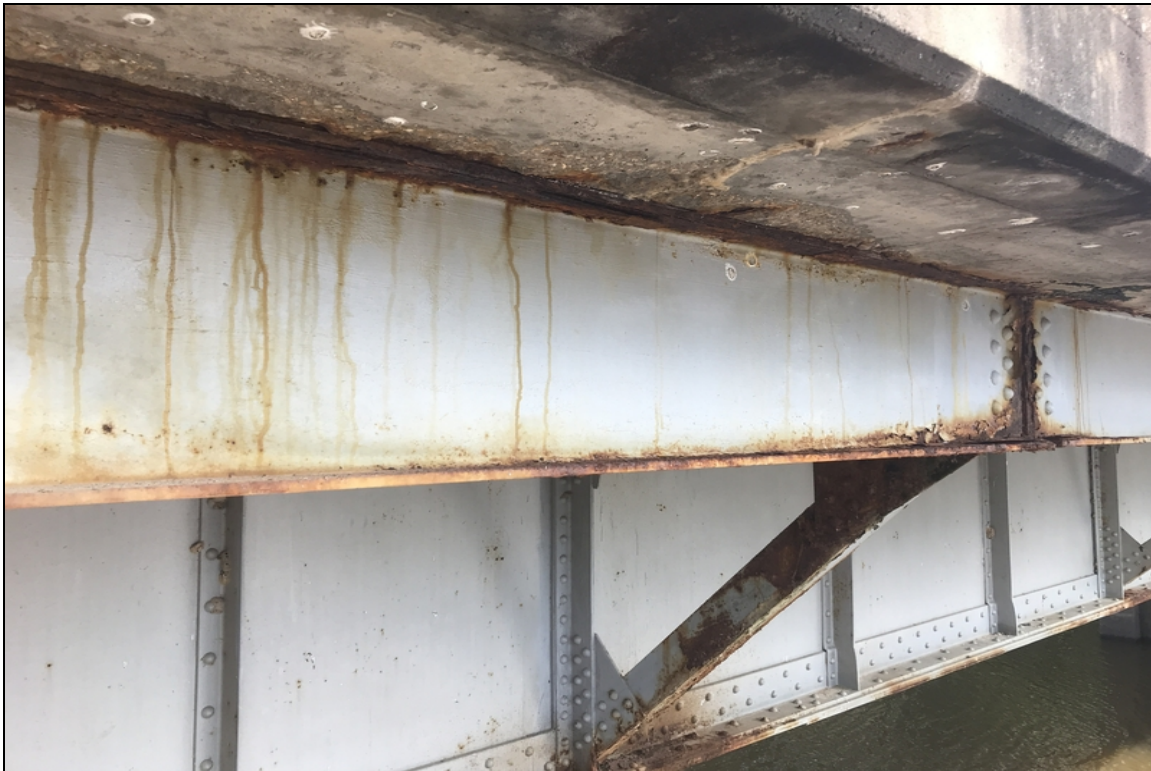
Span 5 outside stringer corrosion
