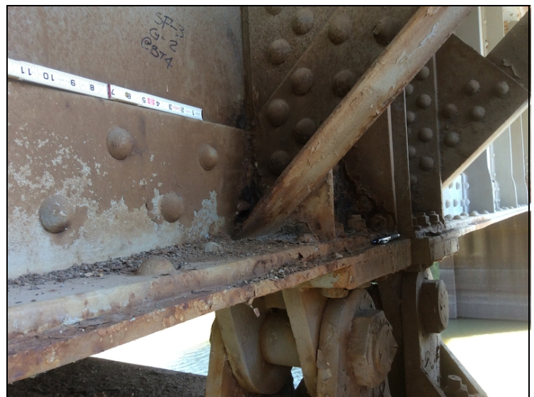
Span 3, girder 2, right side at bent 4. The web plate is pitted to 1/8 inch at the diagonal brace and the end vertical stiffener.
