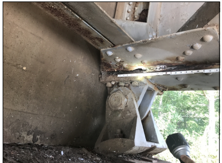
Pier 1, Span 3, girder1, 6"x1" hole in gusset plate were lateral bracing ties in above bearing 1.
