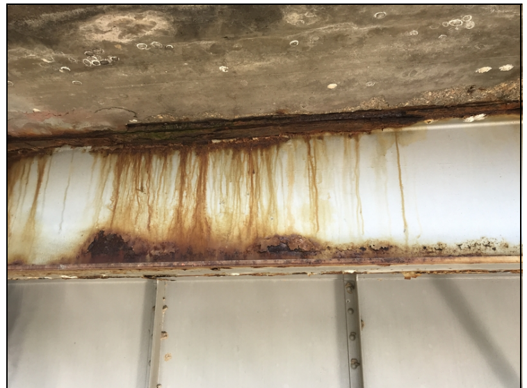
Span 4, stringer 4: top flange with laminating rust and lower web with measurable section loss. (8' from pier 2 joint)
