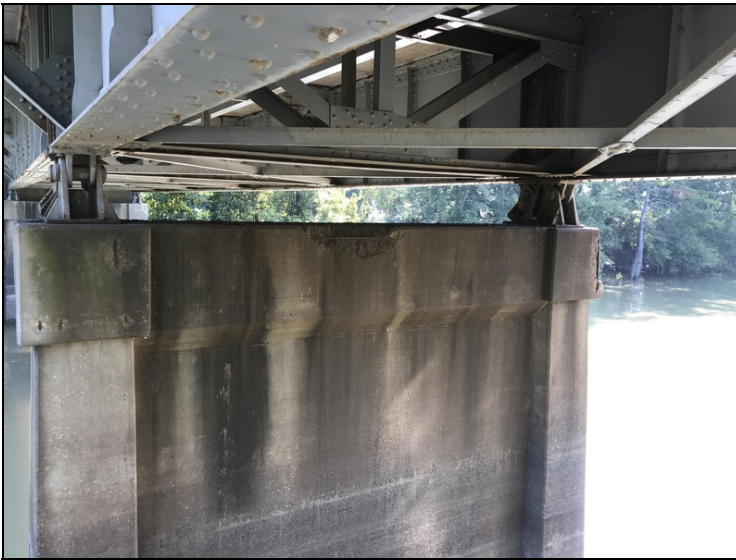
Backside of pier 3 cap has spalls with exposed rebar
