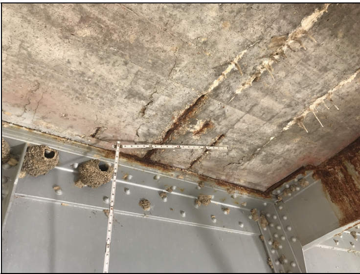
Span 5 right of girder 2: spalls with exposed rebar and transverse cracks with heavy efflorescence build up. Common deficiency at this span
