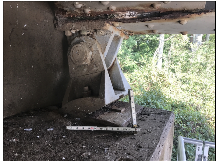
Span 3, girder1 The left edge of the bottom flange at the bearing is corroded down approx. 1/4"
