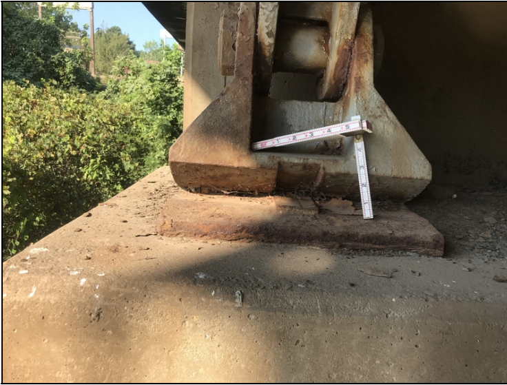
Pier 1, span 3, girder 2: right bearing fully rotated back. Girder 2 bearing in similar condition
