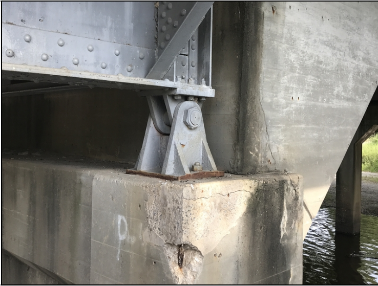
Right side pier 4: diagonal crack in the step up of the cap, also the main cap below.
