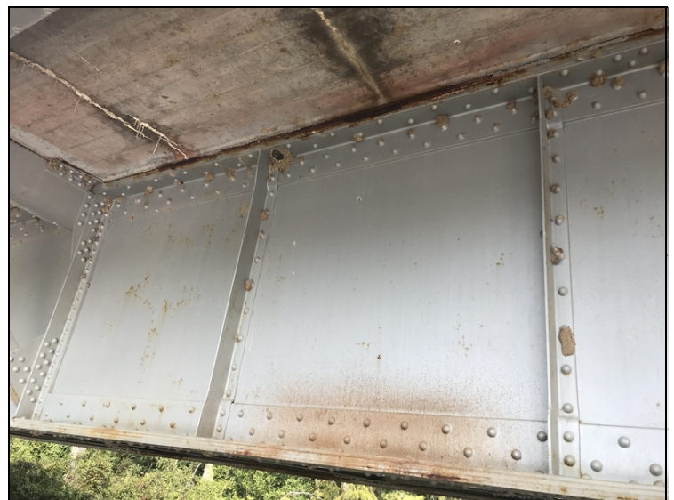
Span 3, right girder left face. Deck cracking is allowing water to rust the top flange and "wash out" on the web and bottom flange.
