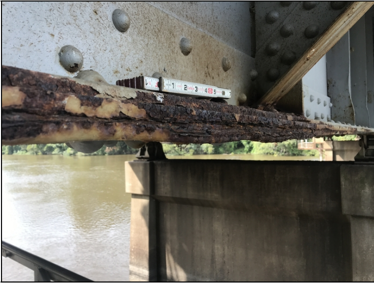
Span 5 girder 1, left side 1/2" of pack rust between the plates of the bottom flange, Approx. 20 feet ahead of bent 5.
