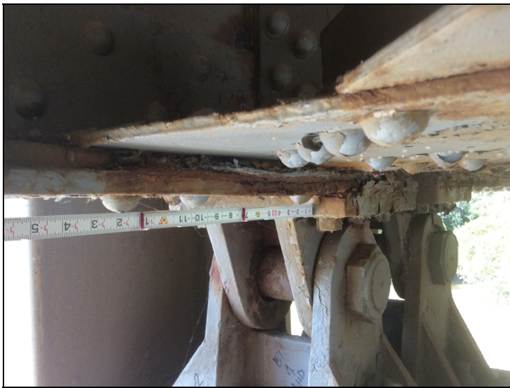
Span 4, girder 2 at bent 4 on the left side. Pack rust has deformed the bottom flange near the bearing.
