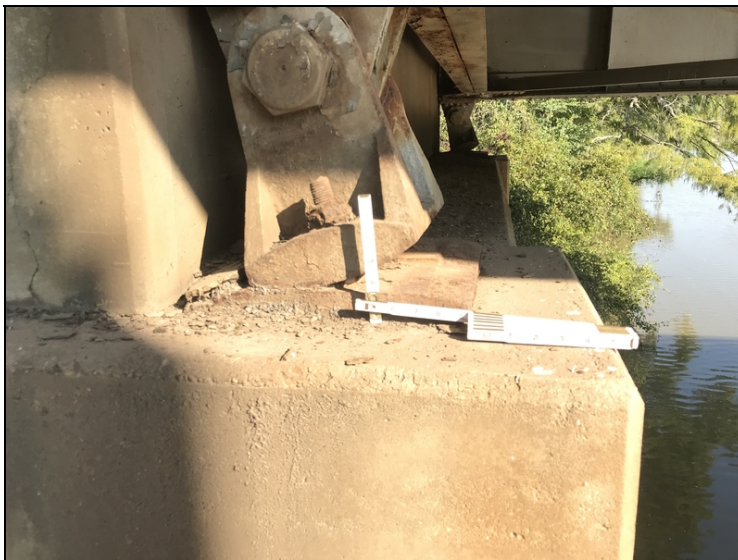
Pier 1: both right and left bearing are fully rotated back.
