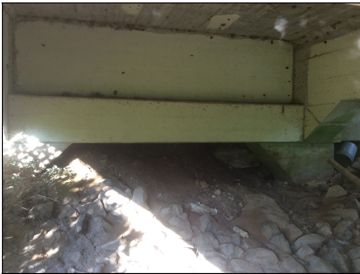
Abutment 1 erosion.
