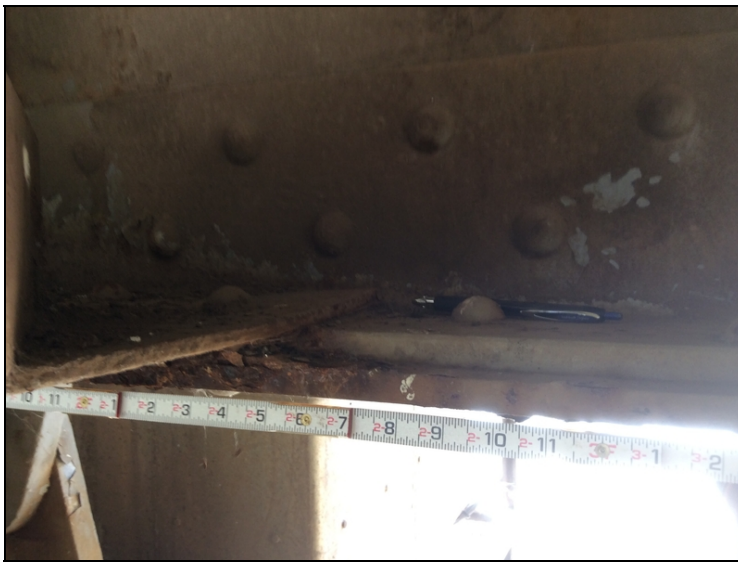
Girder 2, three feet back from bent 4. Pack rust has developed between the diagonal brace gusset plate and the top of the bottom flange.
