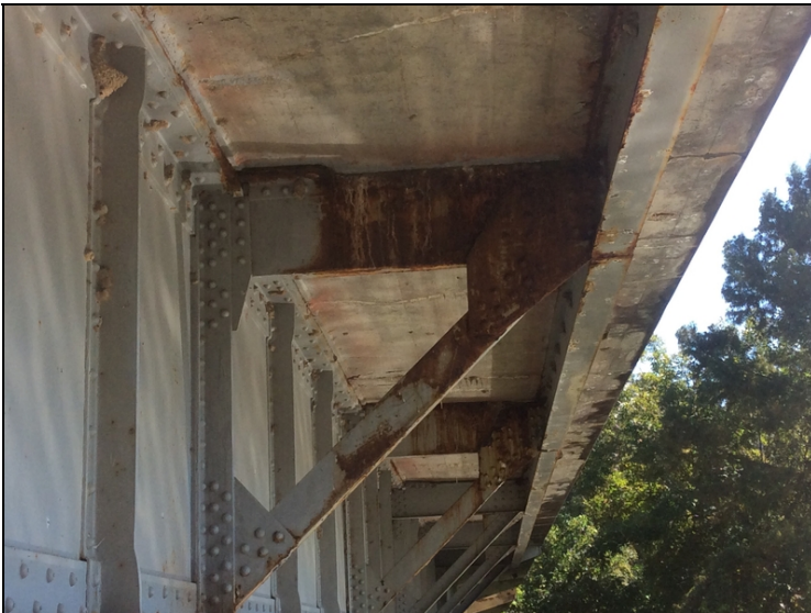
Span 5 right of girder 2 active rust on the cantilevered floor beams.
