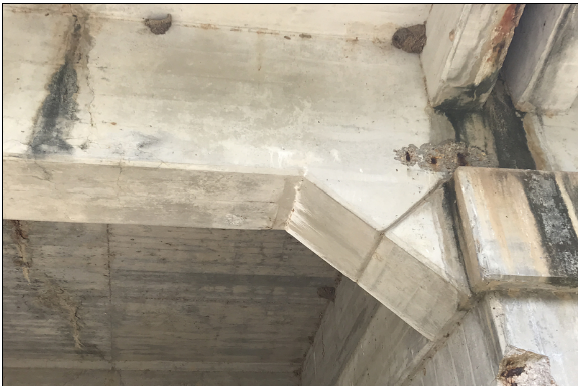
Span 7 girder 2 at bent 8 spall with exposed rebar on right side.
