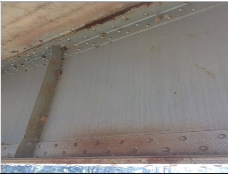
Span 3, right girder left face. Deck cracking is allowing water to rust the top flange and "wash out" on the web and bottom flange.
