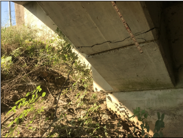
Bent 1, span 1, girder 2: Transverse crack in the girder near the cap.
