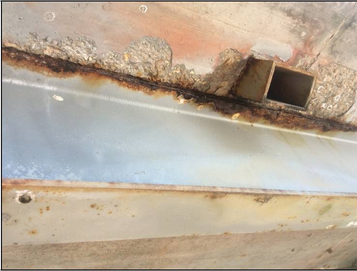
Span 3 right side stringer 4 active rust to top flange at scupper drain.
