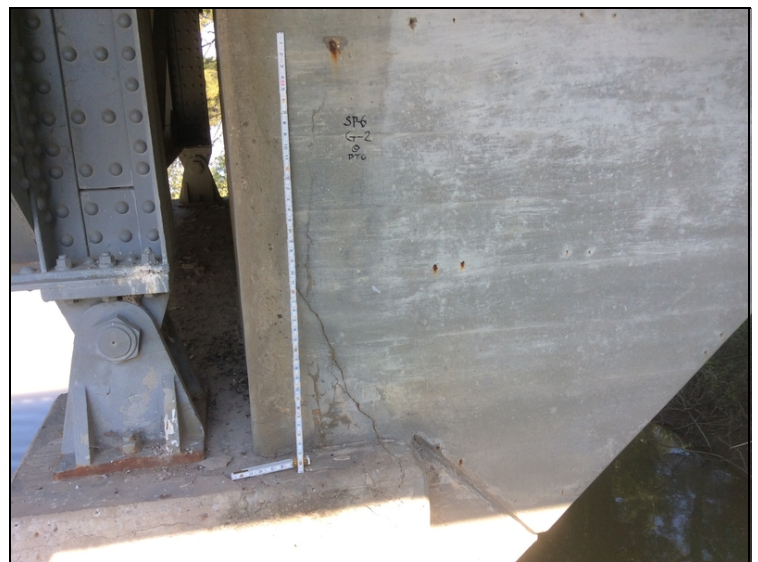
Span 6, girder 2 Cracking at the end of the girder.
