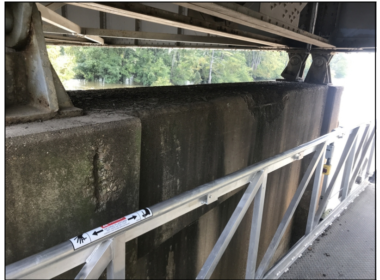
Pier wall 3 cap spalls with exposed rebar
