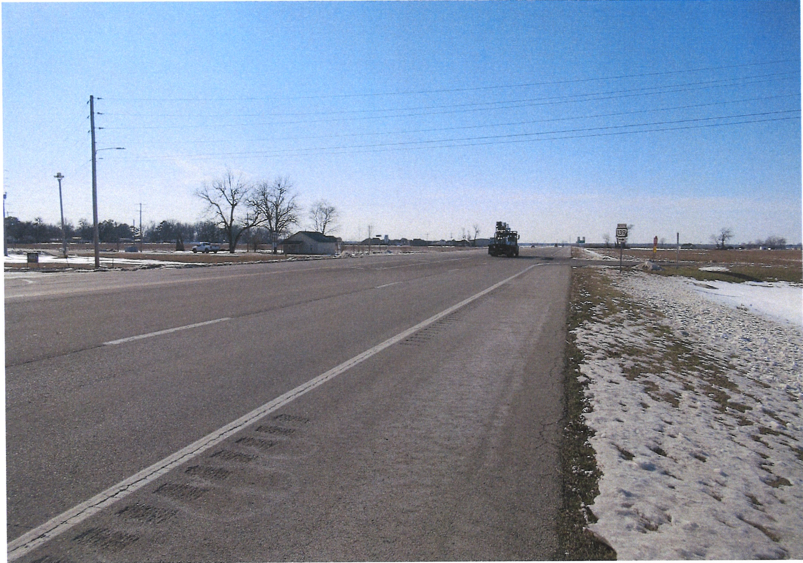
Looking west on Highway 18.
