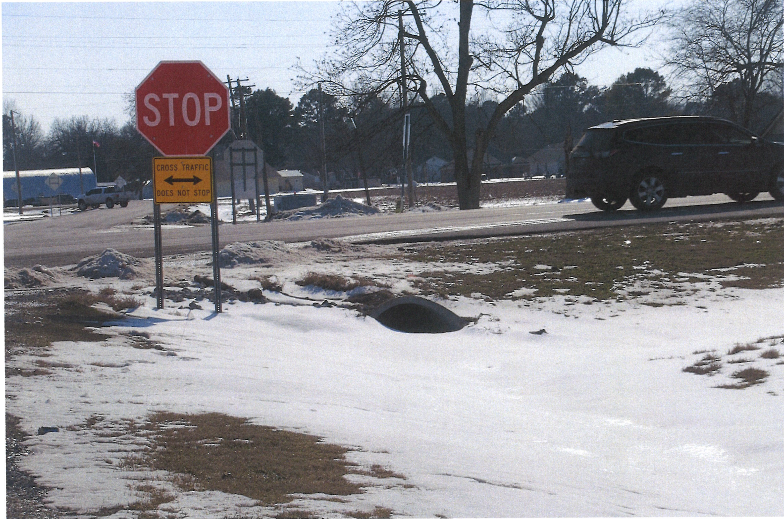
Culvert under Highway 18, west side of intersection.
