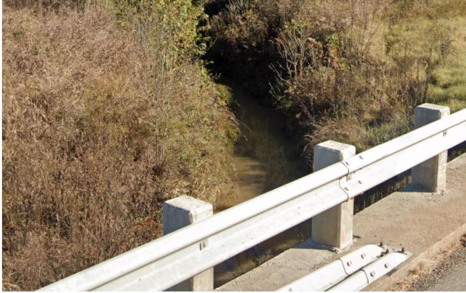
OW 105 (Oak Creek Ditch) - Upstream
