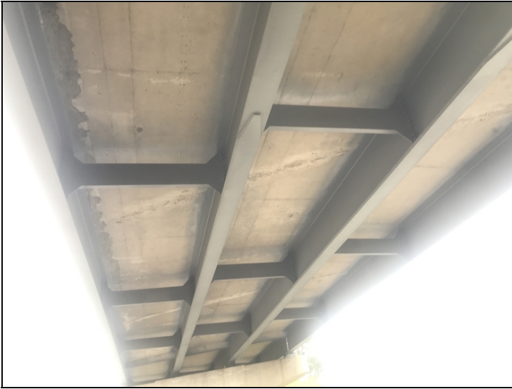
Span 3 girders repaired
