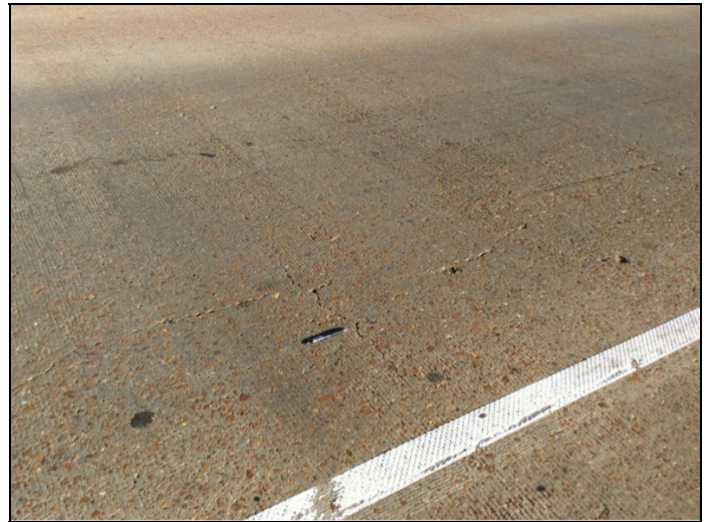
Typical deck cracking
