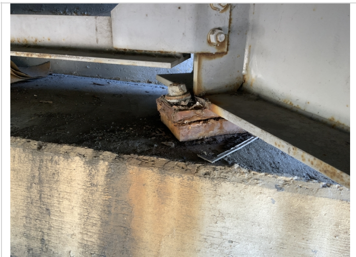
Bent 2 (Girder 6 / Bearing 6) has heavy corrosion with flaking rust, pack rust, and section loss.
