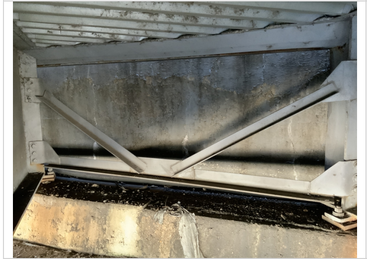
Typical cracking with efflorescence along the back walls of both abutments
