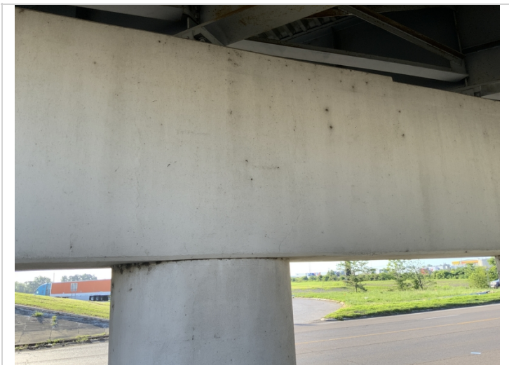
Typical cracking along bent 2 cap.
