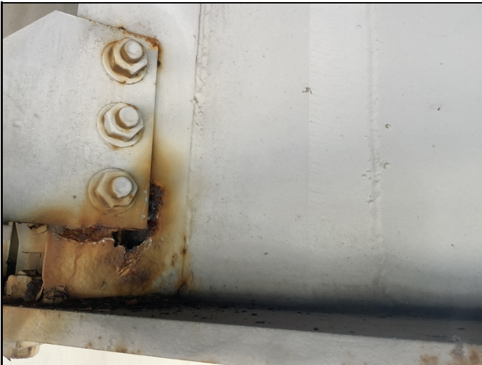
Girder 3 (Span 2) has active corrosion with 100% section loss along the bottom diaphragm connection adjacent to bent 3.
