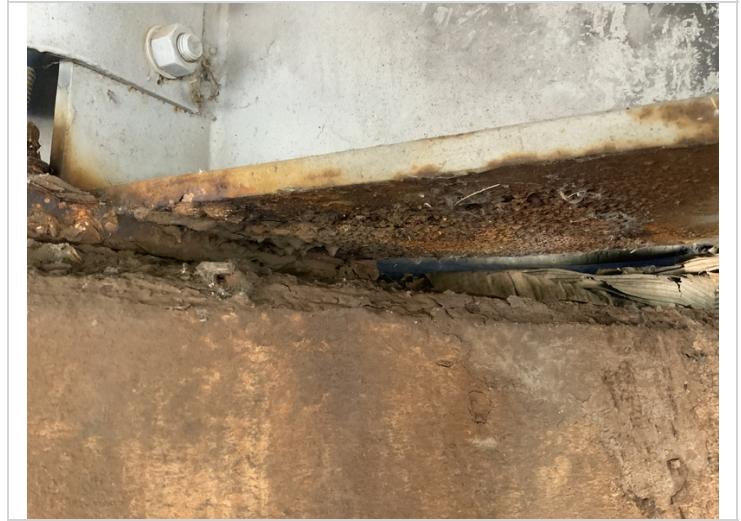
Bent 1 (Girder 4) has active corrosion with heavy pitting along the bottom flange. Bt1 sp4 g4 heavy corrosion flaking rust
