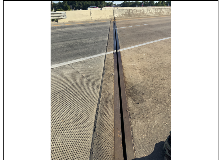
Bent 1 compression joint has 100% of the joint laying on top of the bridge seat causing water and road debris to leak onto the bridge seat and beam ends.
