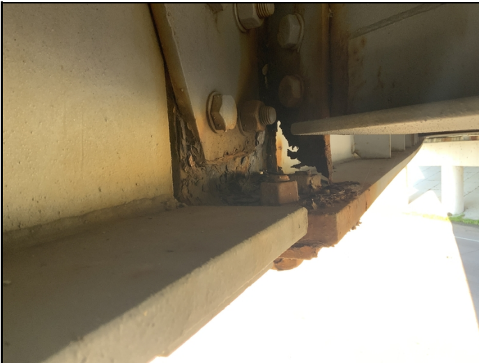
Girder 5 (Span 2) has active corrosion with 100% section loss along the bottom diaphragm connection adjacent to bent 3.
