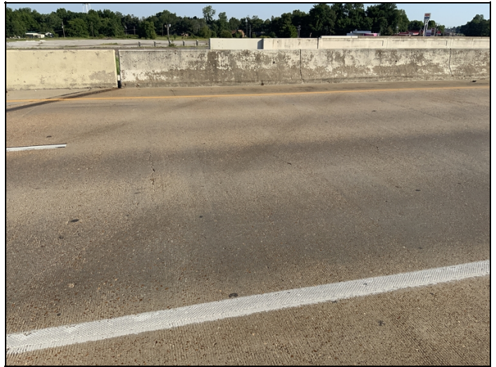
Typical transverse cracking at various spacing throughout the driving structure
