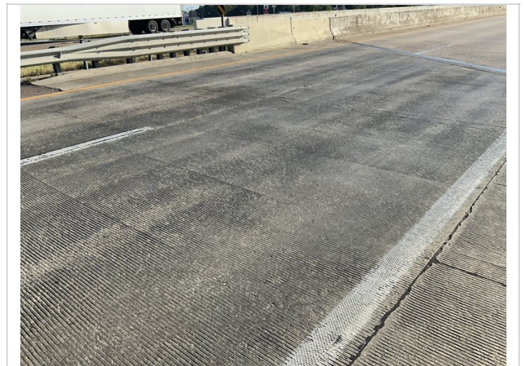
Typical map cracking in various locations throughout the driving surface
