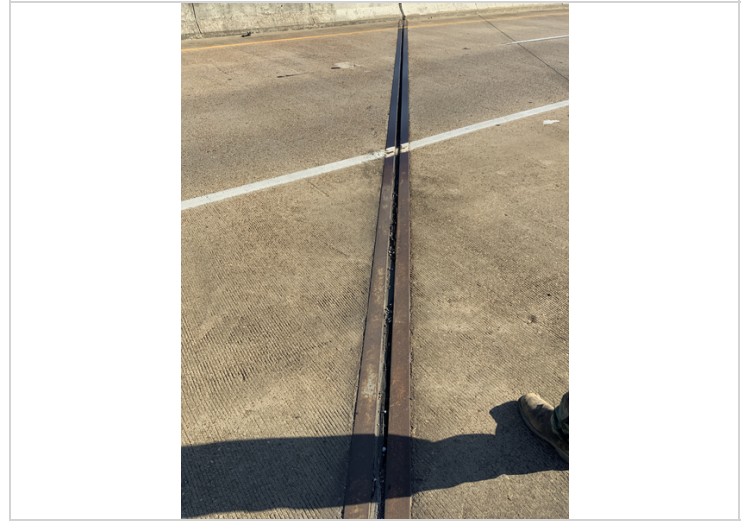
Bent 3 joint has seal cracking along the gutter lines and 100% leakage along the travel lanes allowing water and road debris to accumulate along the bent caps and beam ends.
