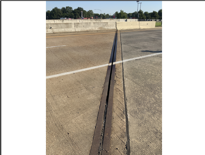
Bent 4 joint seal has adhesion failure and loss of joint material causing 100% leakage.
