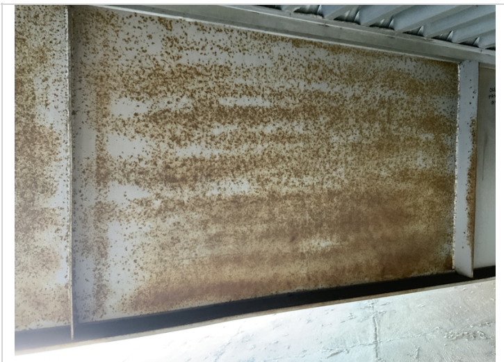
Typical failing paint with light to moderate corrosion along the webs of the girders throughout the structure.
