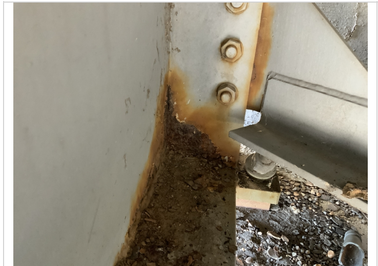
Bent 1 (Girder 6) has active corrosion with flaking rust and light to moderate pitting along the beam end.
