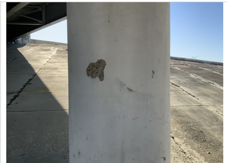
Bent 3 (Column 3) has one shallow spall
