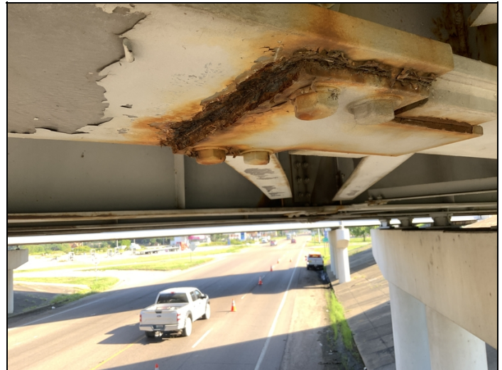
Girders 4 and 5 (Span 2) wind-locks adjacent to bent 3 have 1/8" section loss along the bottom flanges.
