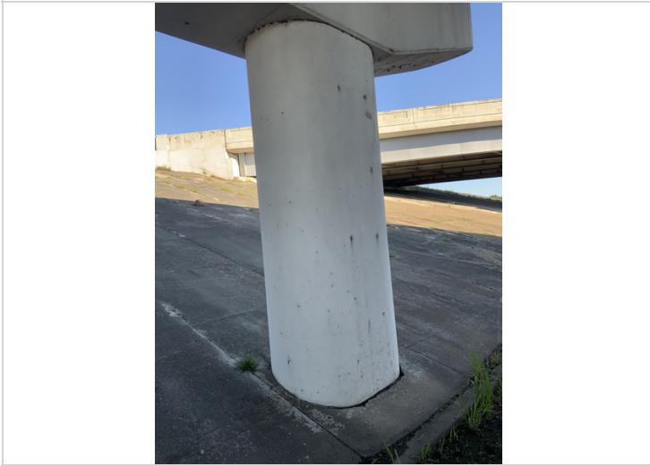
Bent 2 (Column 1) has cracking going around the column.
