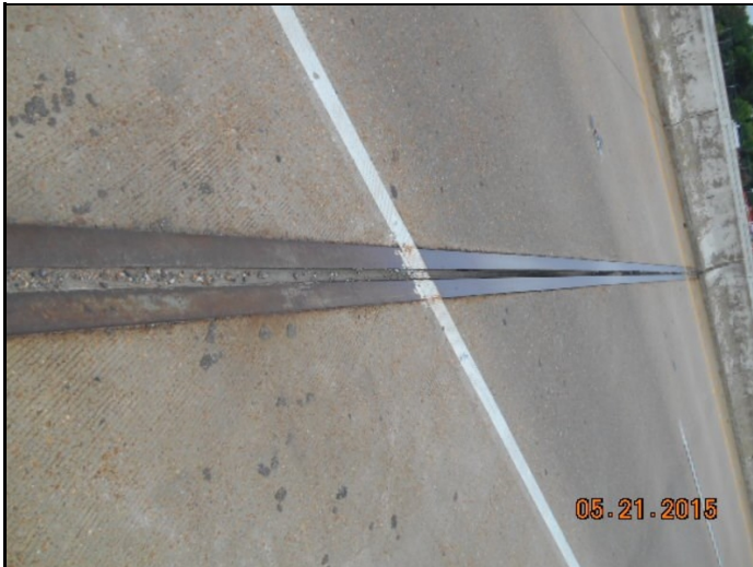
B3162 05-21-2015 Bent 2 Joint seal
