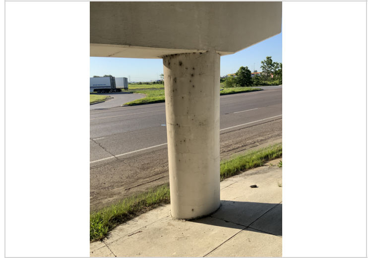
Bent 2 (Column 4) has map cracking going around the column.
