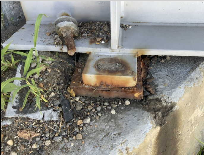
Bent 4 (Girder 1 / Bearing 1) has active corrosion along the bearing and one anchor bolt that has been sheared off due to corrosion.
