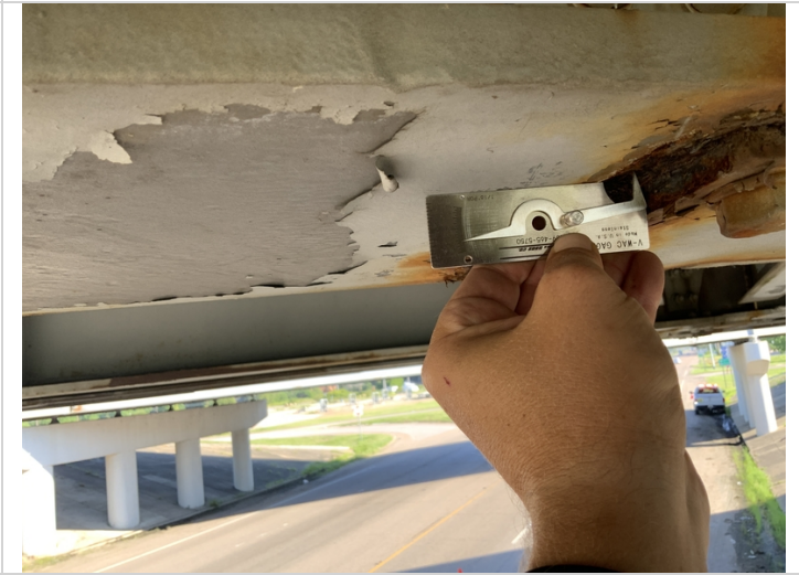
Girders 4 and 5 (Span 2) wind-locks adjacent to bent 3 have 1/8" section loss along the bottom flanges.
