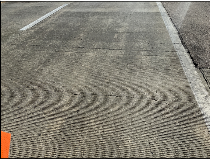
Typical map cracking in various locations throughout the driving surface
