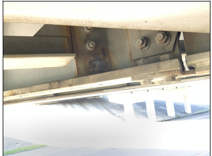
Girder 4 (Span 2) has active corrosion with 100% section loss along the bottom diaphragm connection adjacent to bent 3.
