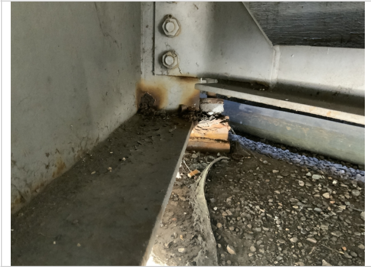
Bent 1 (Girder 6) has active corrosion with flaking rust.
