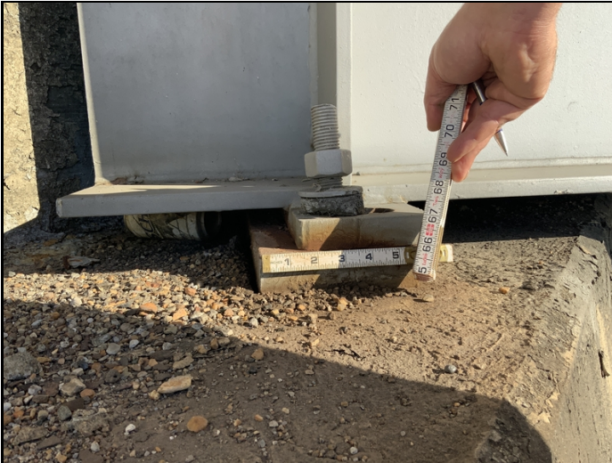
Bent 1 (Girder 6 / Bearing 6) has 1.75" of misalignment
