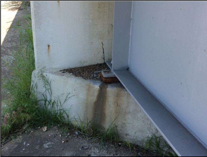
Bent 4 girder 1. Anchor bolt missing.
