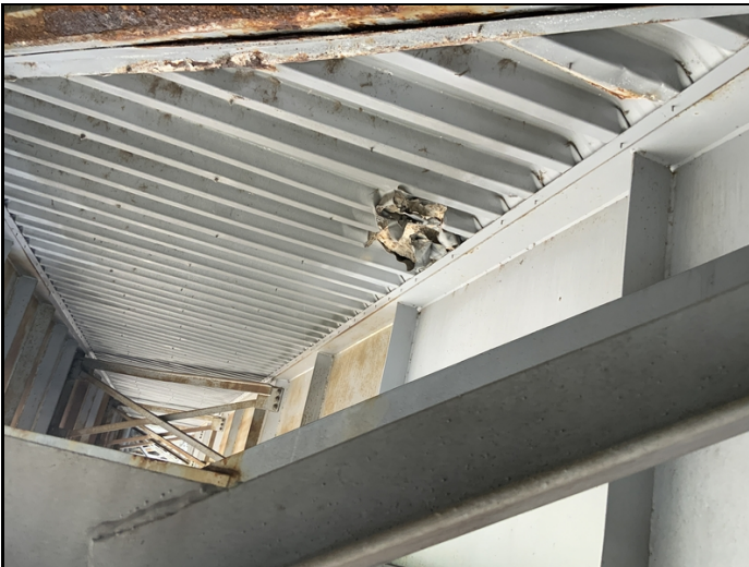
Between girders 4 & 5 (Span 2) adjacent to bent 3 there is damage to the SIP form along with spalling (This is visible from the undersurface of the deck)
