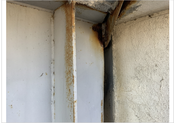
Bent 1 (Girder 1) has active corrosion with flaking rust along the top web juncture.
