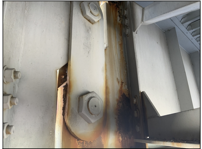
Typical active corrosion with flaking rust and pack rust along the hanger bars
