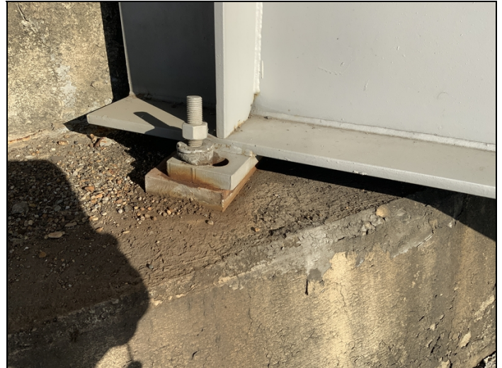
Bent 1 (Girder 6 / Bearing 6) has 1.75" of misalignment
