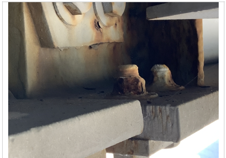
Girder 2 (Span 2) wind-lock connections adjacent to bent 3 has active corrosion with section loss.
