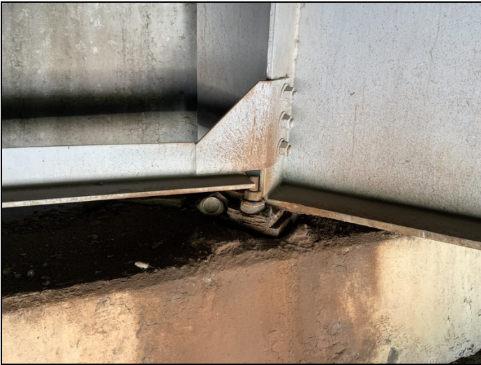
Bent 1 (Girder 3 / Bearing 3) is floating and has heavy corrosion.
