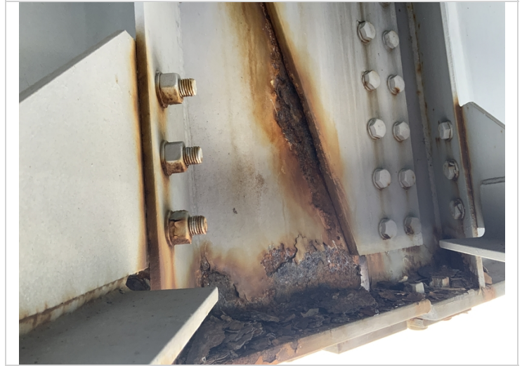
Girder 6 (Span 2) has 3/16" section loss along the web adjacent to the pin and hanger assembly.
