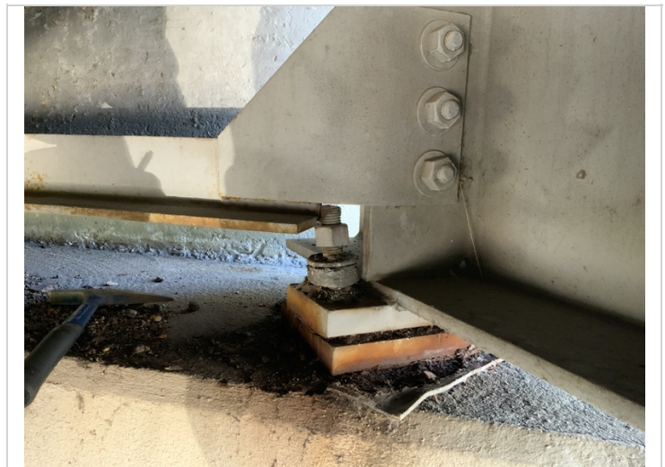
Bent 1 (Girder 1 / Bearing 1) has active corrosion with pack rust.
