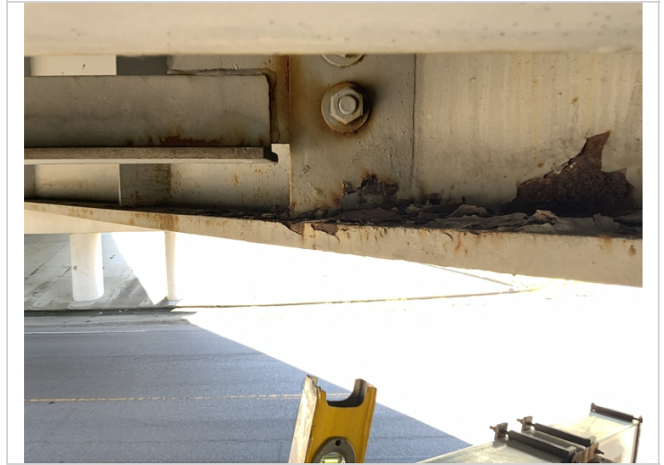
Girder 2 (Span 2) has active corrosion with a 100% section loss along the bottom section of the diaphragm connection.
