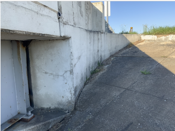
Typical cracking along the wing walls of both abutments
