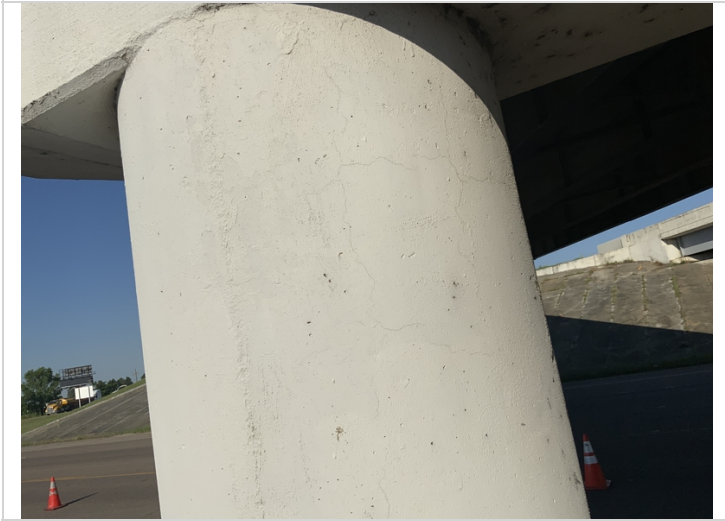
Bent 3 (Column 4) has map cracking
