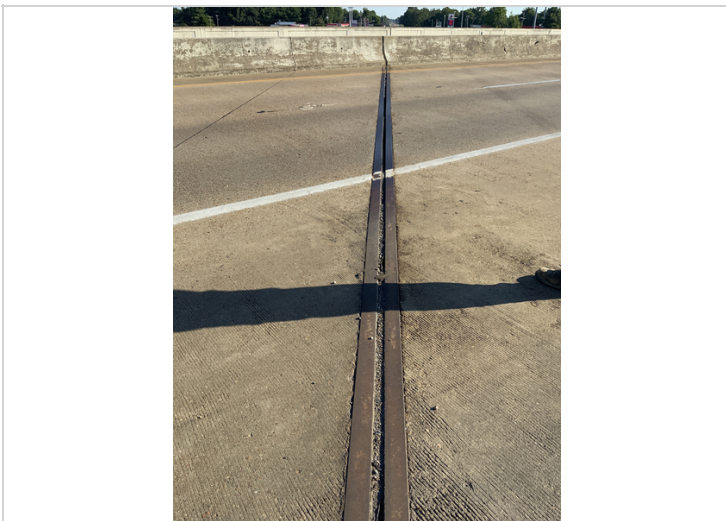
Bent 2 joint has debris impact and seal cracking along the gutter lines, plus 100% leakage along the travel lanes allowing water and road debris to accumulate along the bent caps and beam ends.
