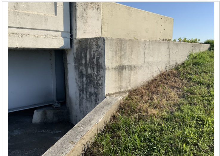
Typical cracking along the wing-walls of both abutments
