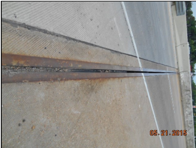
B3162 05-21-2015 Bent 1 Compression seal
