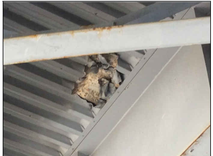
Span 2 bay 3. collision damage to stay in place form.
