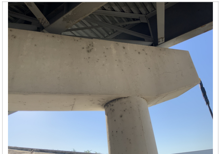
Bent 3 cap has map cracking on both sides
