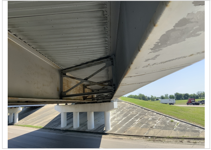
Girder 6 in span 2 has out of plane bending along the bottom flange likely from vehicular collision as evidenced by impact marks.
