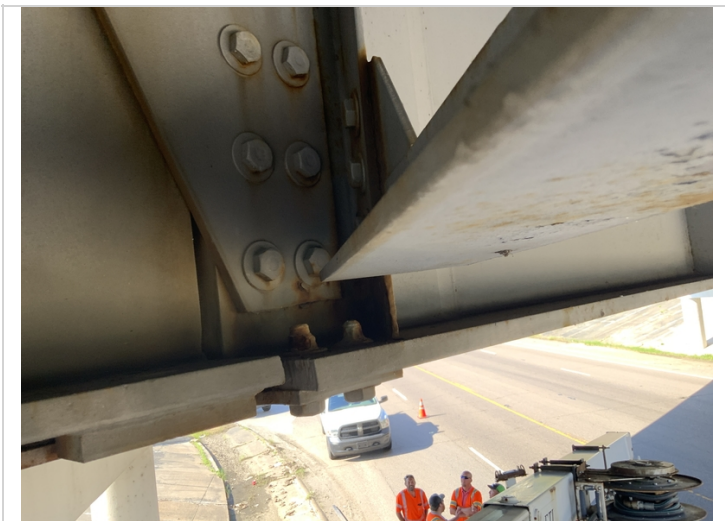
Typical section loss along the wind-lock connections
