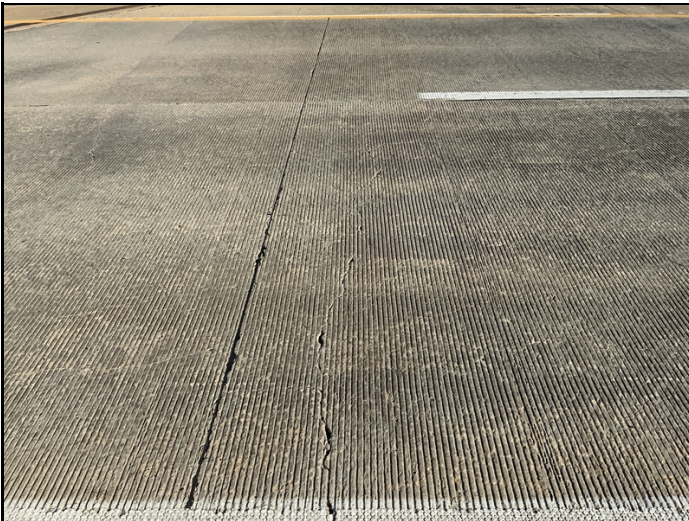
Bent 4 (East Approach Slab) has open transverse cracking
