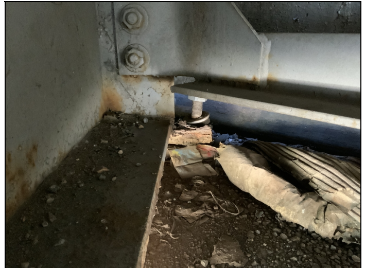
Bent 1 (Girder 4 / Bearing 4) is floating and has heavy corrosion.
