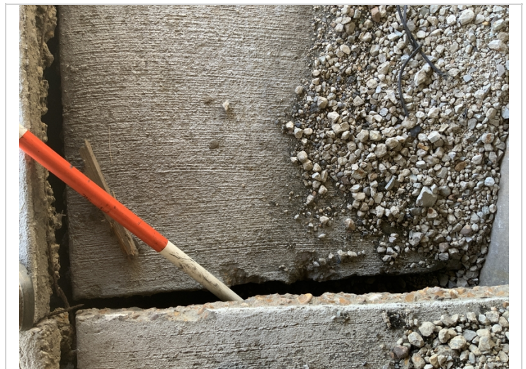
Bent 4 (East Abutment) has erosion and undermining along the bridge seat on the North end of the abutment.
