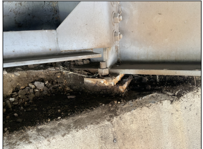
Bent 1 (West Abutment) - (Girder 5 / Bearing 5) has active corrosion with measurable section loss. The bearing at this locations is floating (See files for video of floating bearing).
