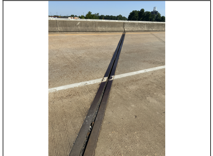
Bent 2 pourable joint has 100% along both of the travel lanes
