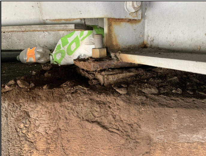
Bent 4 (East Abutment) - (Bearing 4) has active corrosion with measurable section loss. The bearing at this locations is floating (See files for video of floating bearing).
