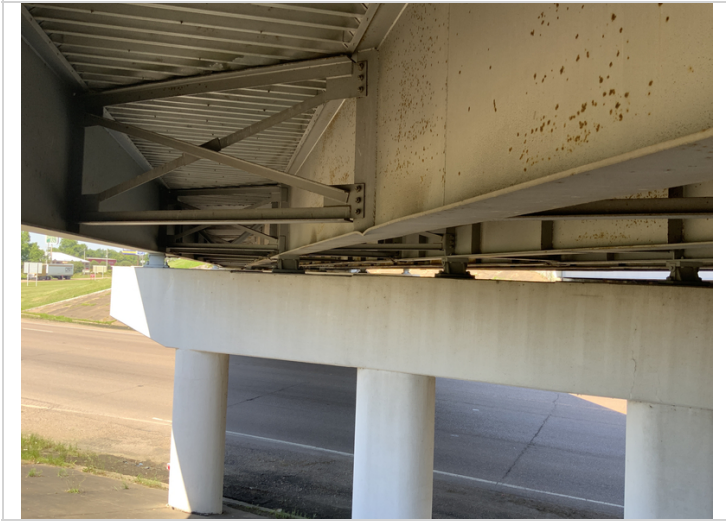
Span 2 (Girders 1 thru 6) distortion along the bottom flanges in the Northbound lane from what appears to be from vehicular impact.
