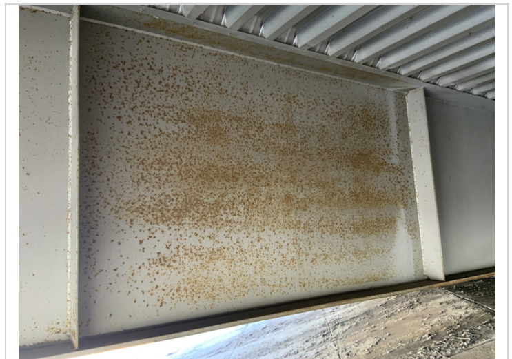
Typical minor pitting in various locations throughout structure.
