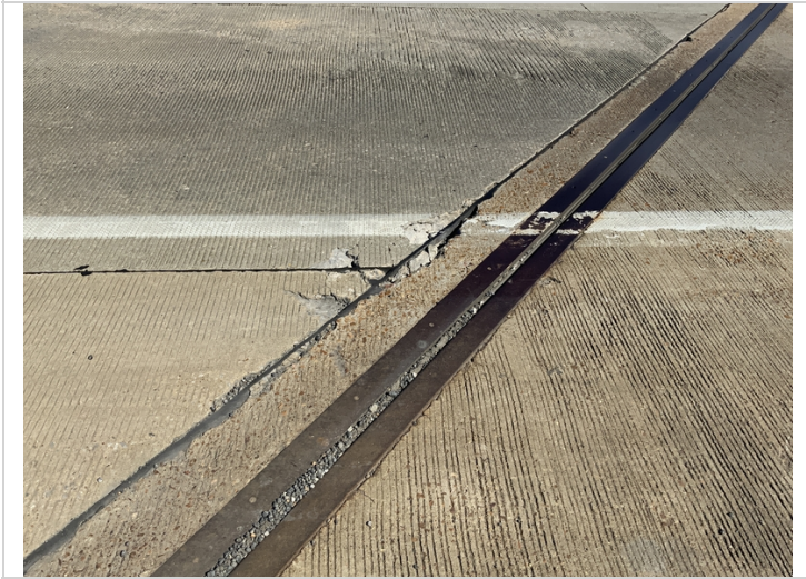
East approach slab has spalling along the outside lane adjacent to the top head wall of bent 4 abutment.
