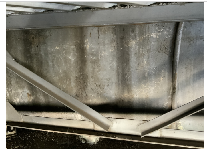
Bent 1 (West Abutment) has map cracking with efflorescence along the backwall between girders 1 and 2 (Bay 1)
