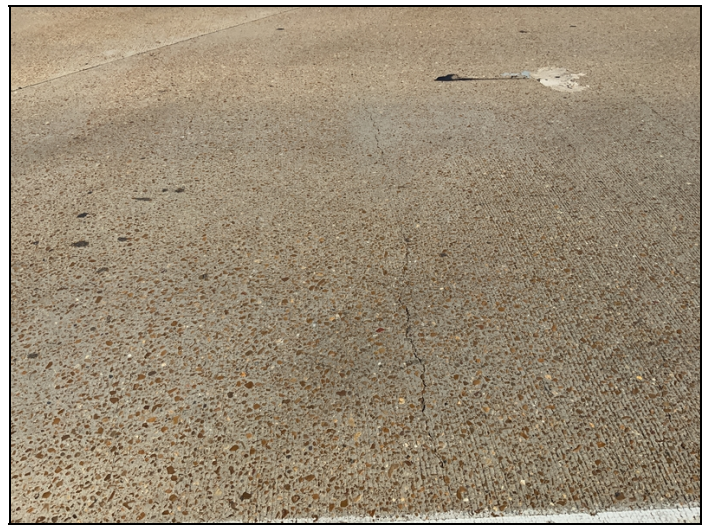
Typical transverse cracking at various spacing throughout the driving surface
