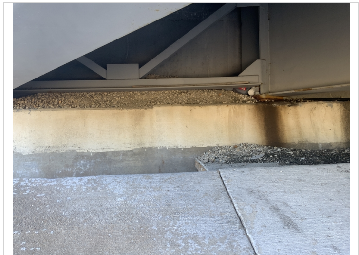
Bent 1 (West Abutment) and Bent 4 (East Abutment) has an accumulation of roadway debris from the failed joints.
