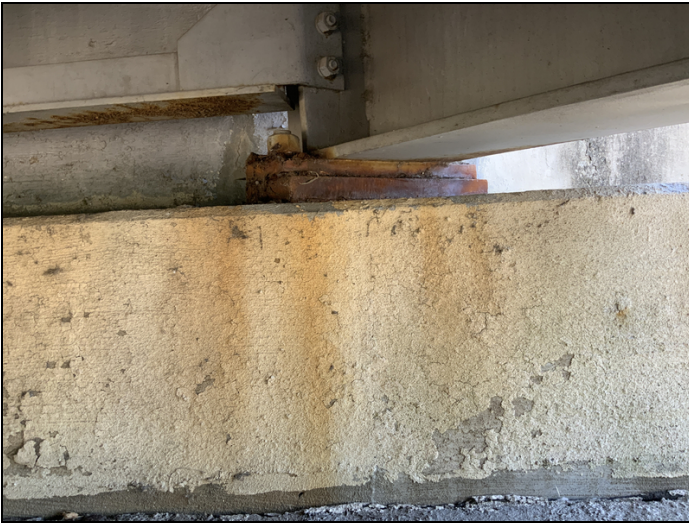
Bent 1 (West Abutment) - (Girder 1 / Bearing 1) has active corrosion with flaking rust and section loss
