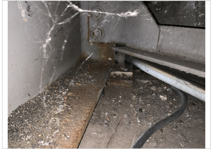
Bent 1 (West Abutment) - (Girder 4 / Bearing 4) has active corrosion with flaking rust along with one sheared anchor bolt.
