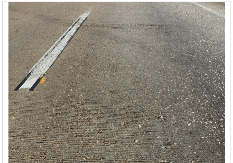
Typical abrasion throughout the driving surface
