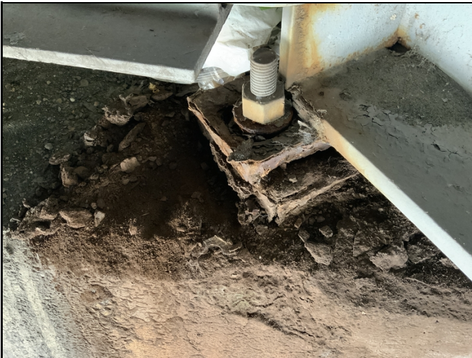
Bent 4 (East Abutment) - (Bearing 4) has active corrosion with measurable section loss.
