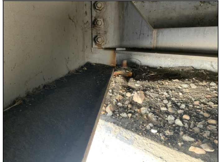
Bent 1 (West Abutment) - (Girder 6 / Bearing 6) has active corrosion with flaking rust along with one anchor bolt that is sheared of on the North side and one missing nut on the South side. (Bearing 6 also has misalignment of approximately 3.25")
