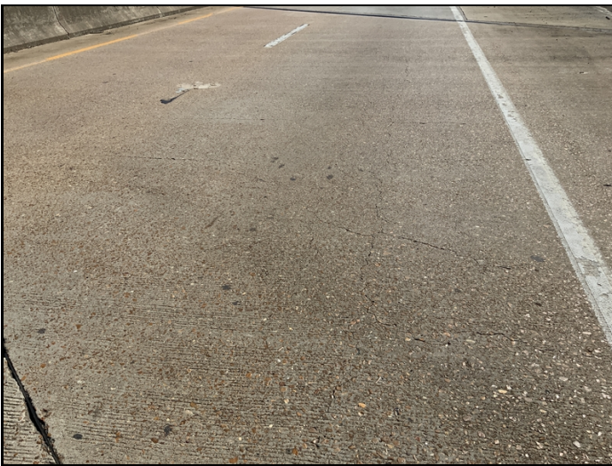
Typical map cracking along the outside lane throughout the length of the driving surface
