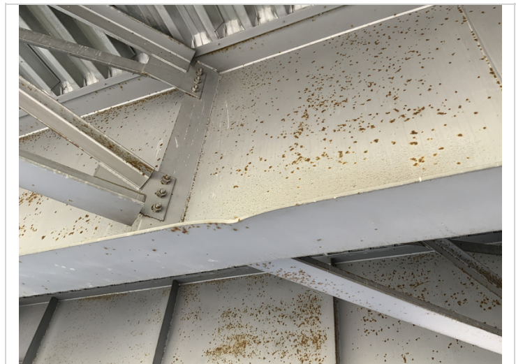
Span 2 (Girders 1 thru 6) distortion along the bottom flanges in the Northbound lane from what appears to be from vehicular impactation.
