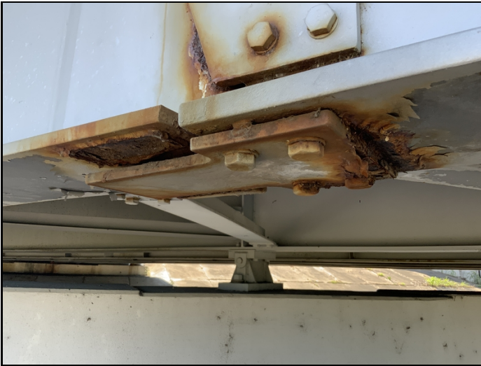
Span 2 (Girder 1) has active corrosion with flaking rust and section loss along the wind-lock connection adjacent to bent 3.
