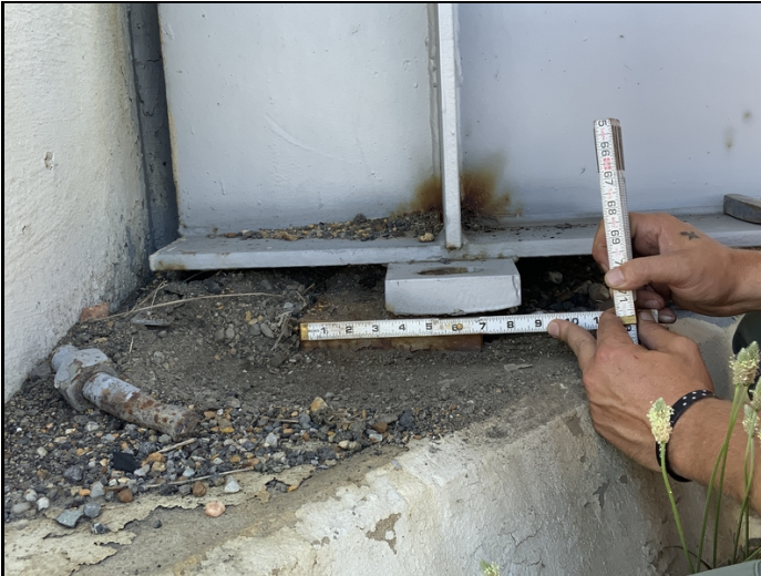
Bent 1 (West Abutment) - (Girder 6 / Bearing 6) has a anchor bolt that has been sheared off with misalignment of approximately 3.25"
