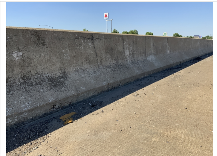
Typical cracking along the concrete bridge railing
