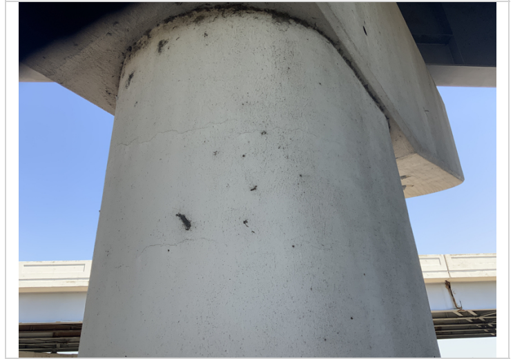
Bent 2 (Columns 3 & 4) has cracking going around the columns
