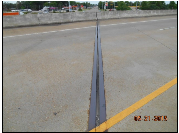
A3162 05-21-2015 Bent 3 Joint seal
