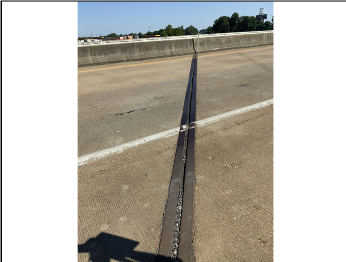
Bent 3 pourable joint has sections of adhesion failure, 100% joint failure (Inside lane approximately 2'), and debris impaction (along the gutter lines).
