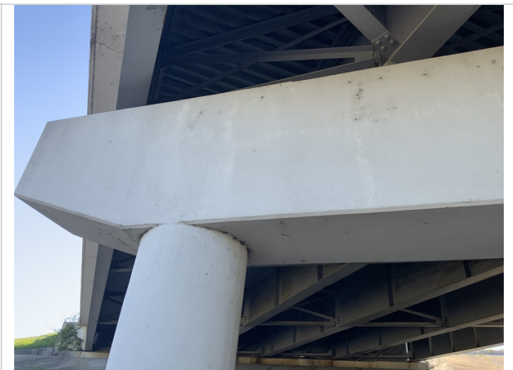
Typical cracking with efflorescence along bent 3 cap
