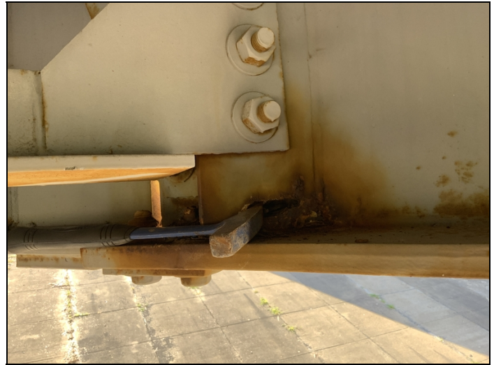
Span 2 (Girder 6) has active corrosion with 100% section loss along the diaphragm connection adjacent to bent 3.
