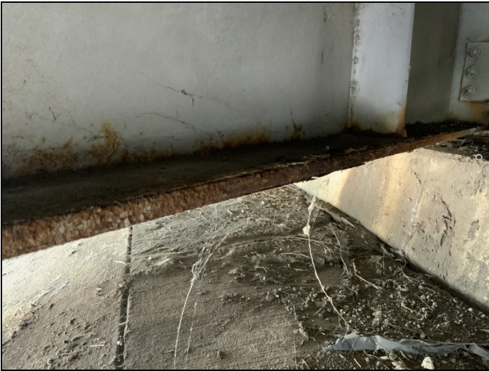
Bent 1 (West Abutment) - (Span 1 / Girder 4) has active corrosion with flaking rust along the bottom flange of the beam end.
