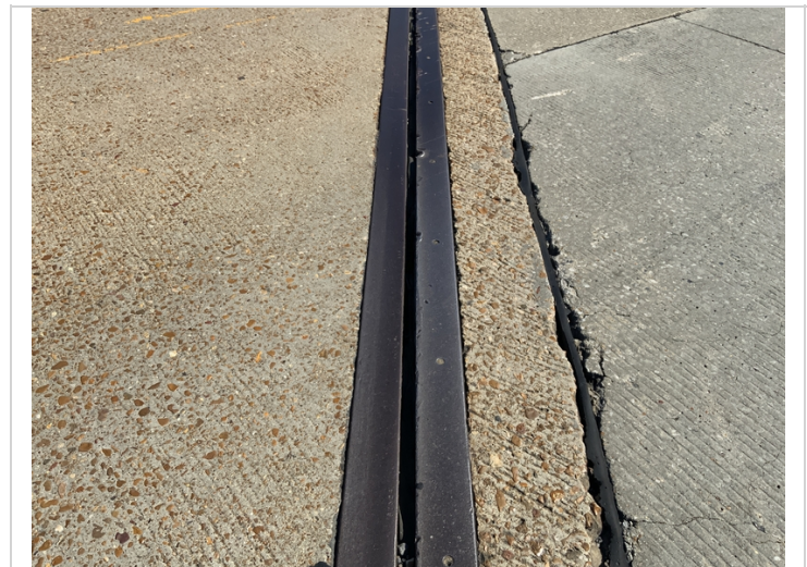
Bent 1 (West Abutment) has adhesion failure, cracking, and joint failure causing water and road debris to accumulate on top of the bridge seat.
