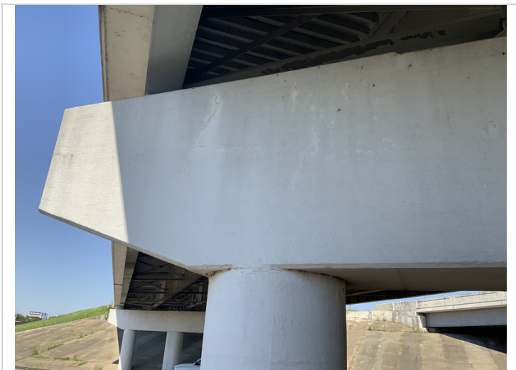
Typical vertical and horizontal cracking with light efflorescence along the cap at bent 2
