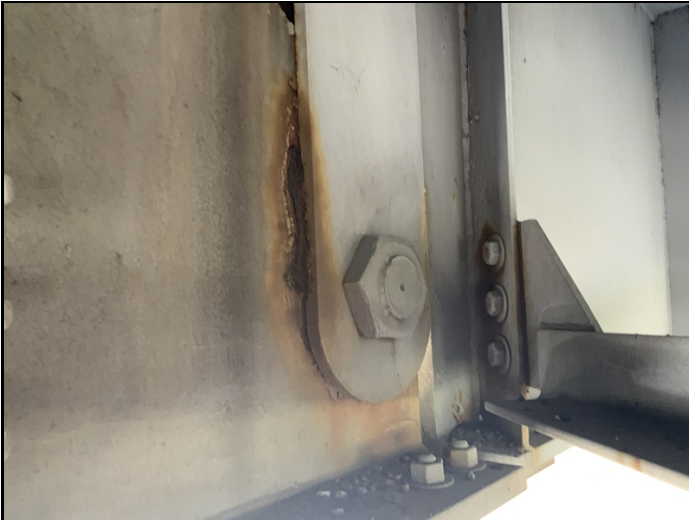
Typical active corrosion with flaking rust and pack rust along the pin and hanger connections
