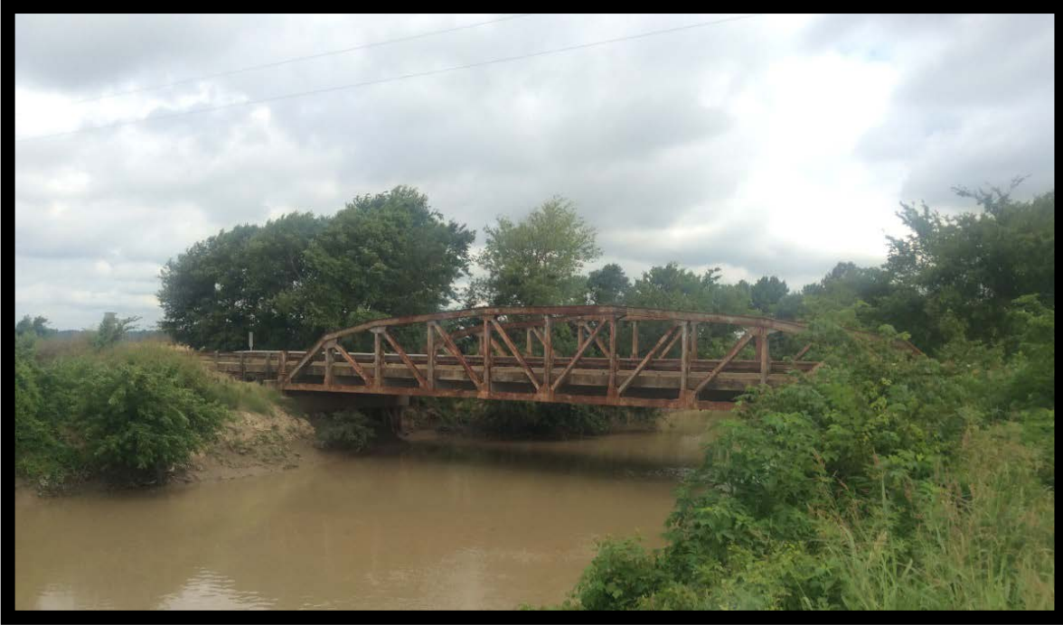
Figure 1: ARDOT Bridge Number M3187
