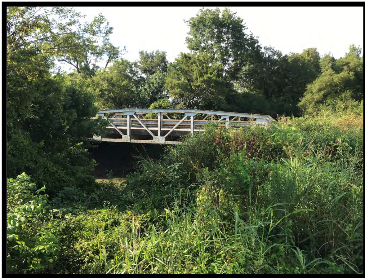
Figure 2: ARDOT Bridge Number M3817
