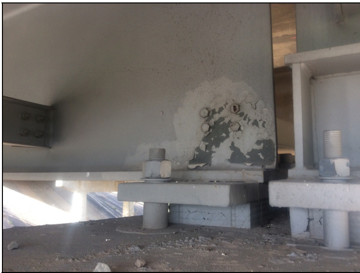
Typical paint peeling to Girder 2 of all spans
