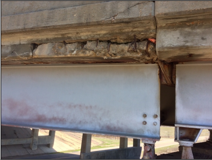
Bent 4 Joint has closed, causing damage to Rt. side curb and overhang.
