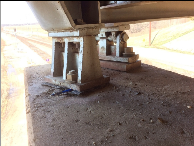
Bent 4 Bearing 7 tilted and twisted, typical for bearings on Bt. 4.
