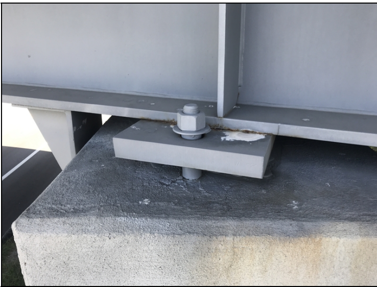
Bent 2 left side no weld.
