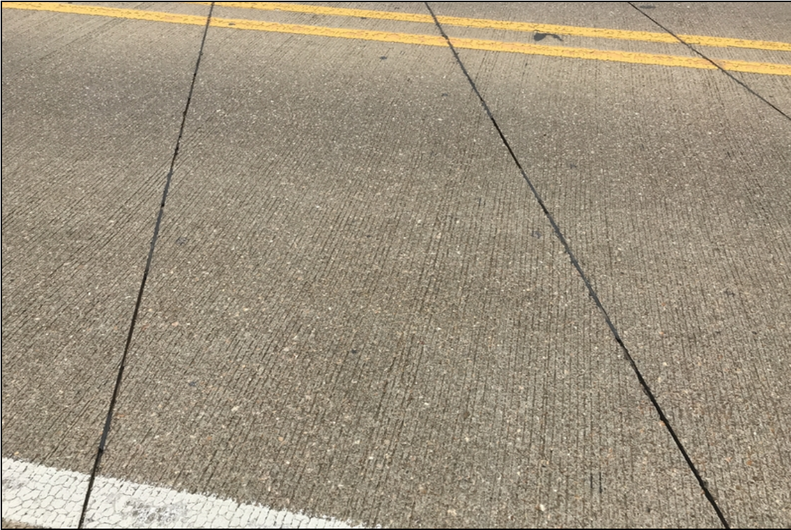
Saw cut joints
