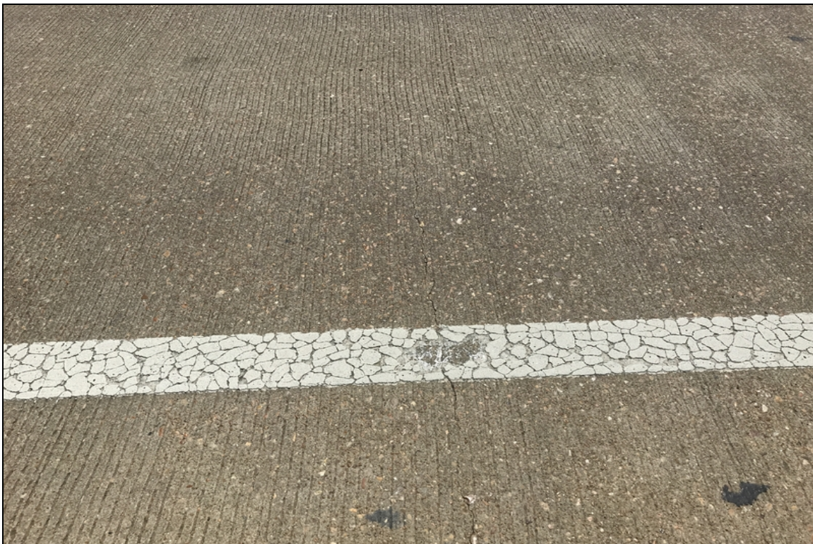
Deck transverse cracks
