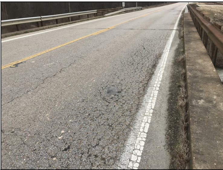
Map crack / rutting
