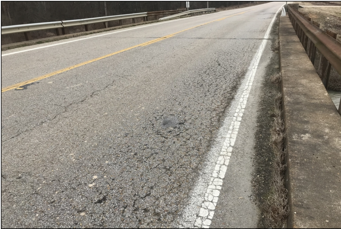
Map crack / rutting
