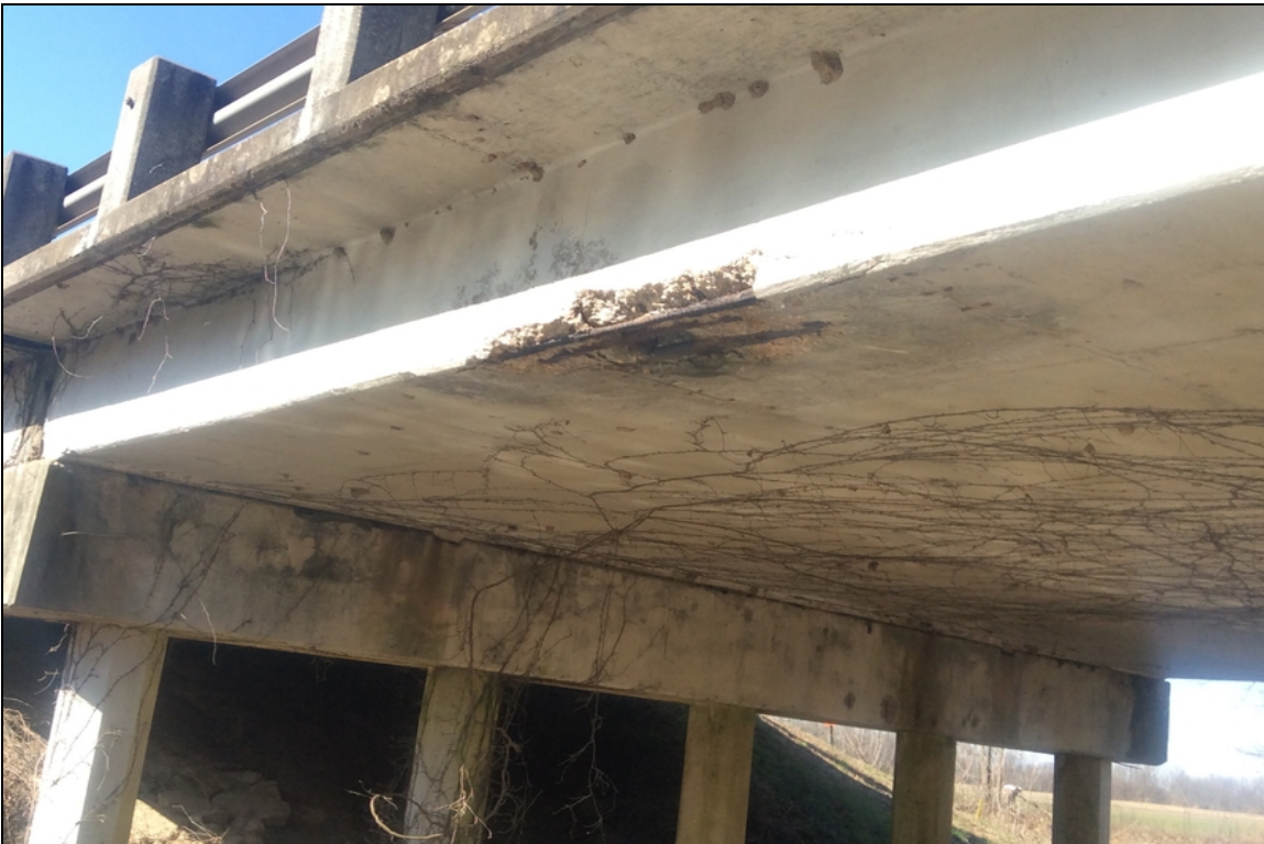
Span 2 shell out area left side to slab
