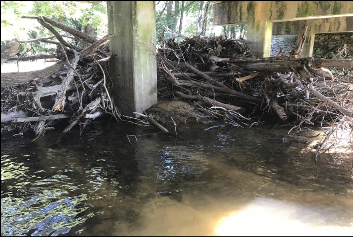
Drift Span 3 LT SIDE 2019
