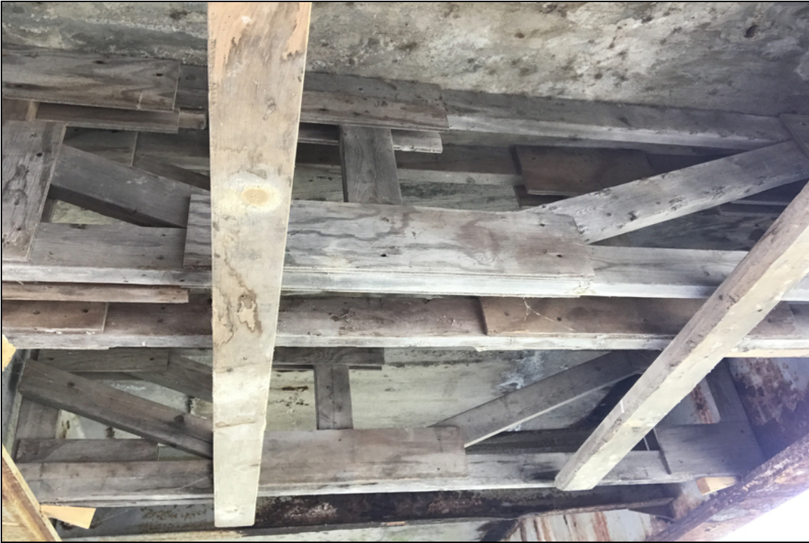
Span 2 bay 1 full depth patch
