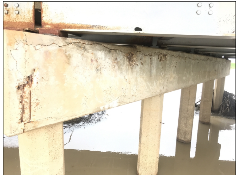
S4 side b4 cap cracks and rebar exposed
