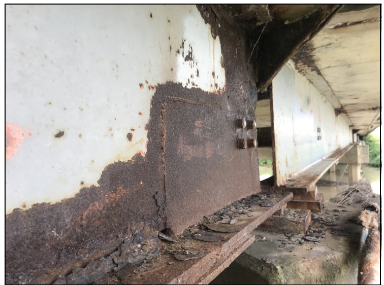
S5 b5 g1 crushing over tsplice
