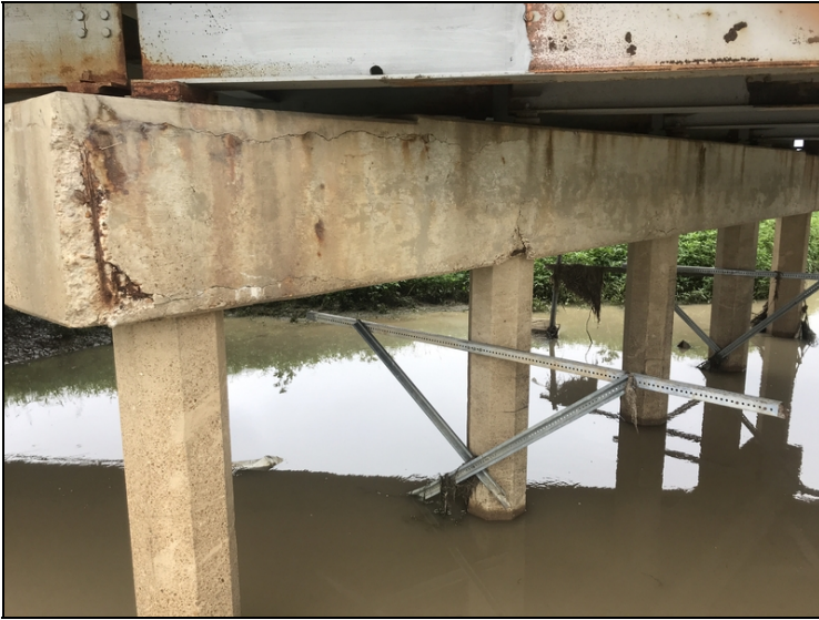
S3 side of b3 cap over piles 3, 4, & 5 delaminated with spalls and rebar exposed
