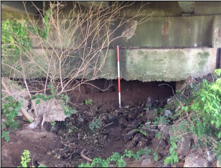
Bent 10 abutment embankment erosion.
