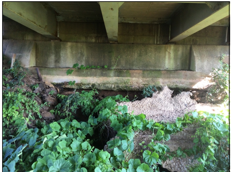
Bent 1 erosion.
