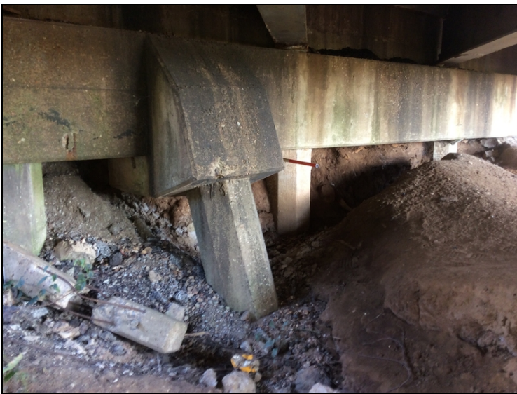
Bent 1 erosion, 2017
