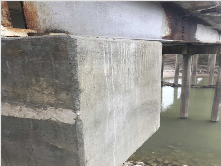
Bent 2 cap RT end repaired
