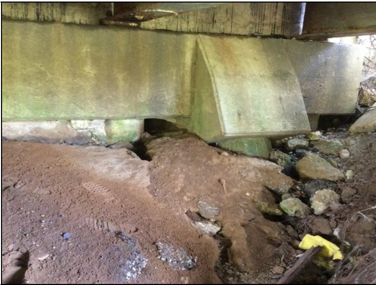
02871 10-01-2015 Bent 9 right end of abutment erosion.
