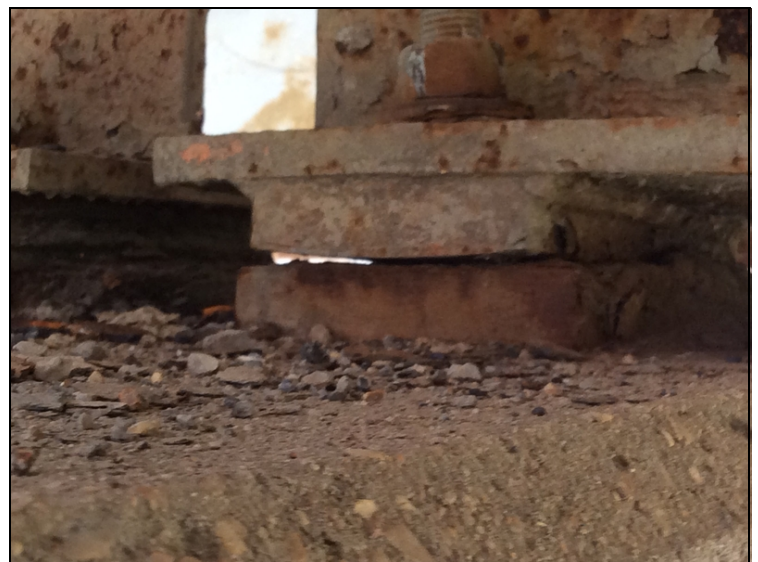
02871 10-01-2015 Span 2 Girder 2 over Bent 3 Movement under traffic.
