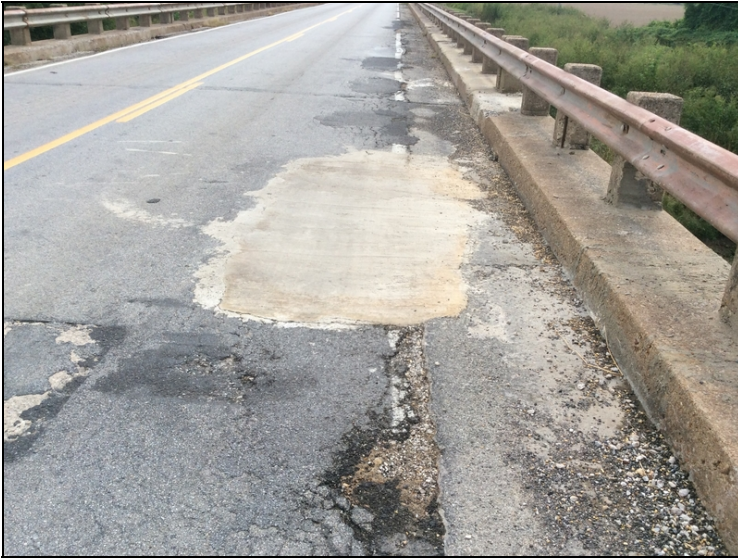
02871 10-01-2015 Span 3 Right lane repair.
