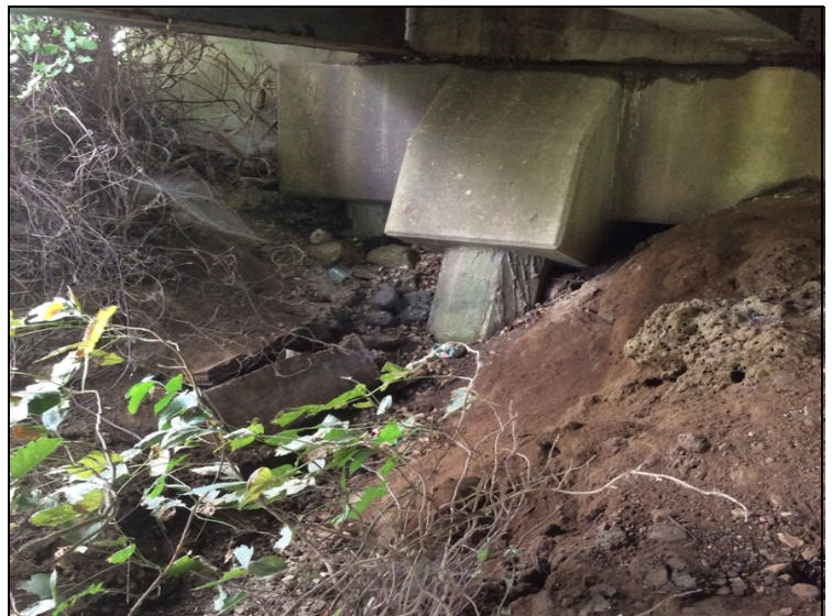
02871 10-01-2015 Bent 9 left end of abutment erosion.
