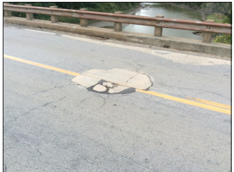
02871 10-01-2015 Span 2 centerline repair.
