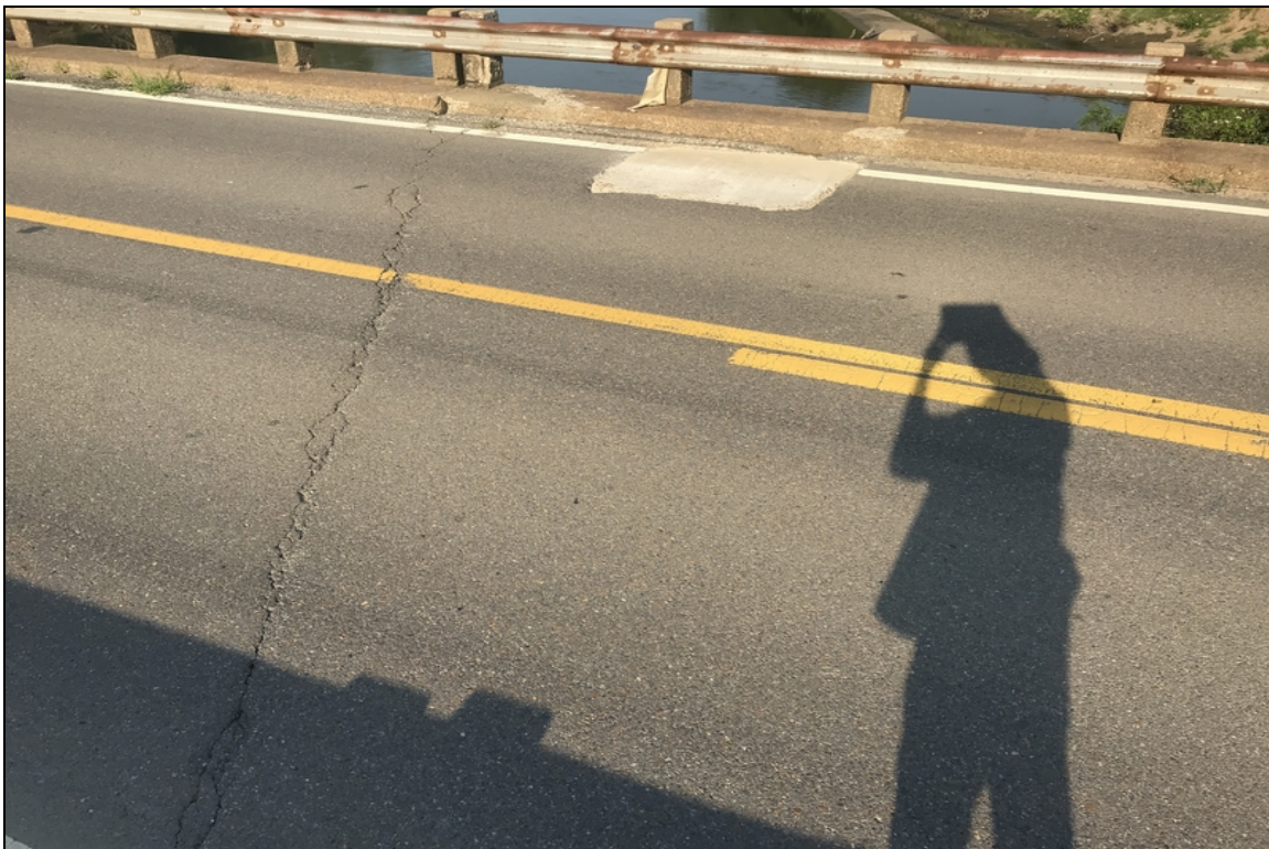
Span 2 near bent 3 full depth patch
