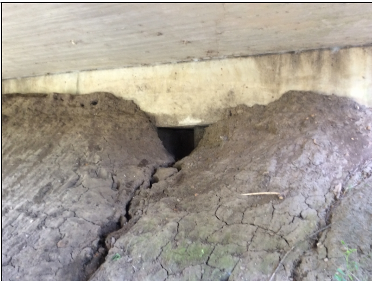
Bent 9 embankment erosion.
