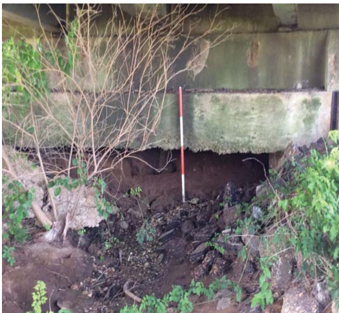
PHOTO 4 Description Bent 10 abutment embankment erosion.
