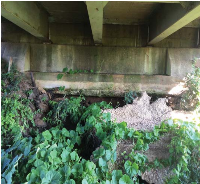
PHOTO 1 Description Bent 1 erosion.
