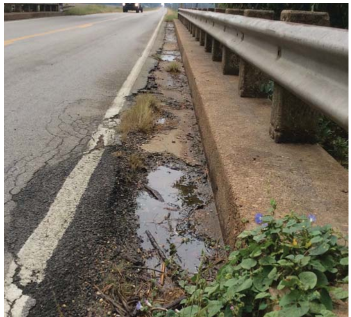
PHOTO 2 Description 02873 09-29-2015 Right gutterline Span 1
