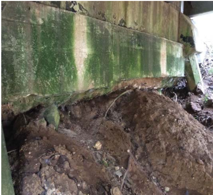
PHOTO 1 Description 02873 09-29-2015 Bent 4 Embankment erosion.
